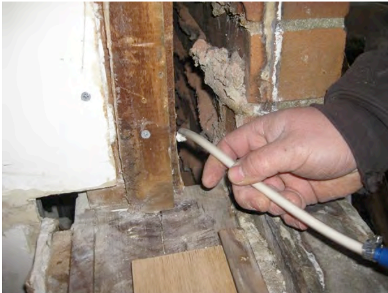
Figure 14. Foam sealant being applied between off-cut wood buck and CMU
