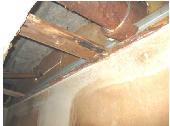
Figure 2: Soffit above kitchen
