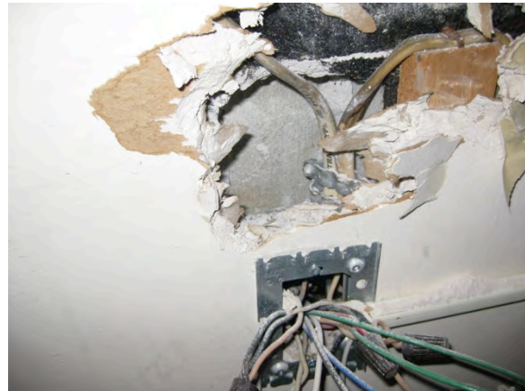
Figure 9. Left: Small hole in mortar joint of exterior wall; Right: Large existing hole in CMU of exterior wall apparently created to accommodate electrical and communication services.
