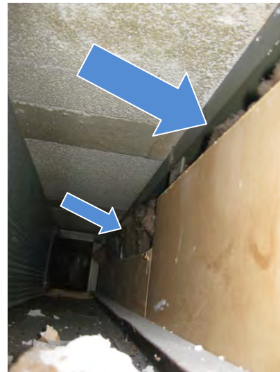
Figure 5. Left: Annular seal at easily accessible plumbing penetration; Right: Within the duct soffit enclosure, the demising wall is not continuous to the ceiling.
