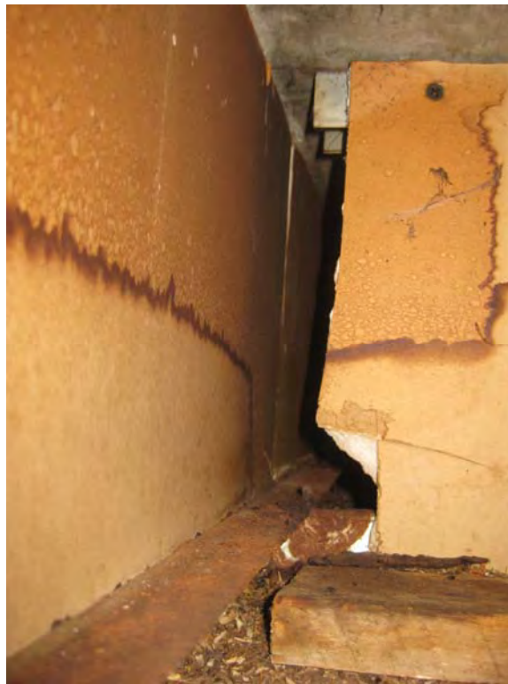
Figure 5: View from kitchen soffit (demolished) into perpendicular soffit containing supply duct
