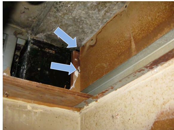
Figure 7. Left: Where work exposes the joint between the exterior wall and floor slab, there is an opportunity to ensure a robust air seal at this joint; Right: As seen in this exposed section above the kitchen soffit, the demising wall does not connect to the exterior wall structure. This leaves a path for airflow around the demising wall.
