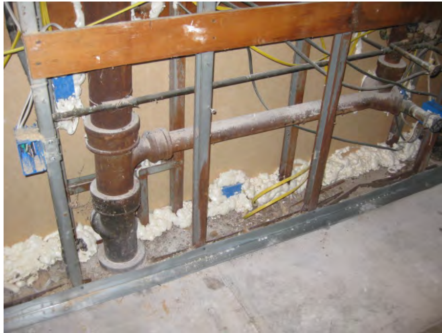
Figure 21. Demising wall at kitchen air sealed from open side of wall.
