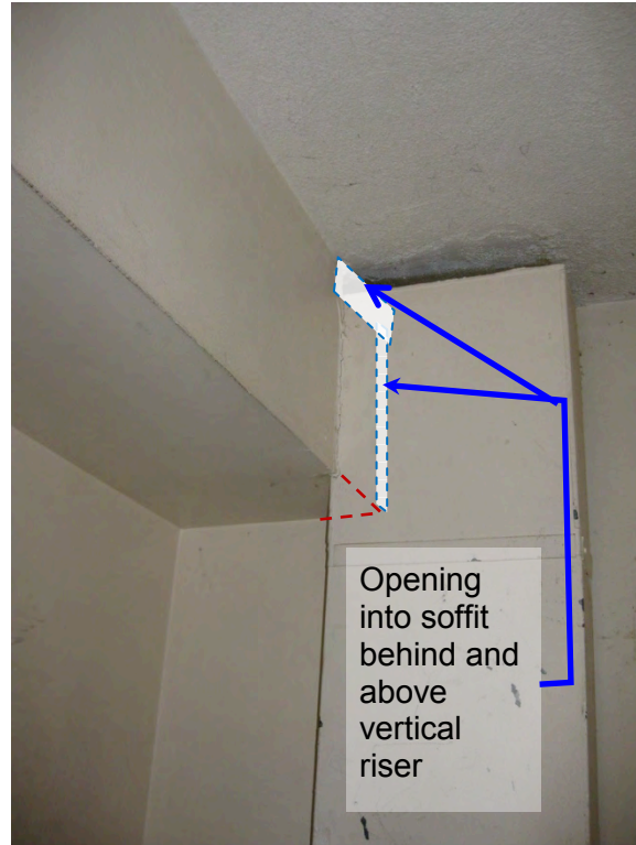
Figure 18. Opening into soffit at second floor of low-rise mock-up apartment.
