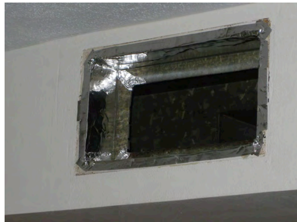
Figure 3. Left: Gaps between duct boot and drywall created a bypass for heating distribution and also represented significant leakage pathways into the demising wall and, consequently, between apartments; Right: The work scope called for metal extension sleeves and foil mastic tape to seal from the existing duct, over the extension sleeve to the face of the drywall.
