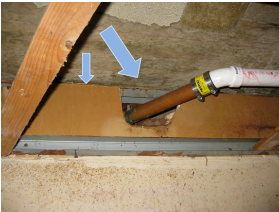
Figure 6. Left: Large discontinuities in demising wall surface round plumbing and other services above the soffit. Drywall surface is not sealed to floor/ceiling above; Right: Demising wall surface is not sealed to floor slab.
