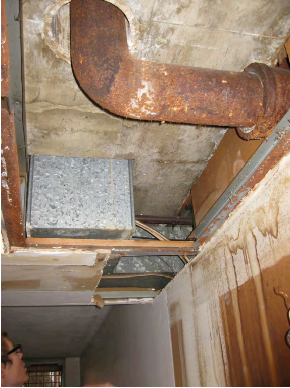
Figure 8. Dead-end stub of supply plenum extends through demising wall. Left: View of supply plenum with kitchen soffit and cabinets removed; Right: View into demising wall cavity through large opening around dead-end stub of supply plenum.
