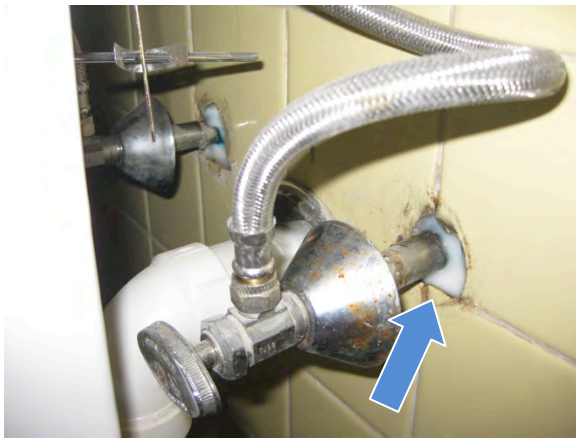
Figure 5. Left: Annular seal at easily accessible plumbing penetration; Right: Within the duct soffit enclosure, the demising wall is not continuous to the ceiling.
