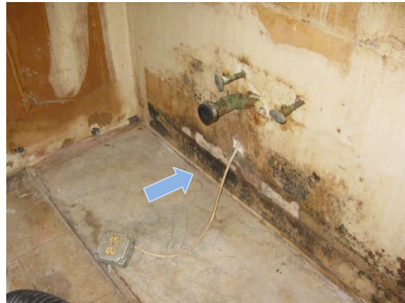
Figure 6. Left: Large discontinuities in demising wall surface round plumbing and other services above the soffit. Drywall surface is not sealed to floor/ceiling above; Right: Demising wall surface is not sealed to floor slab.
