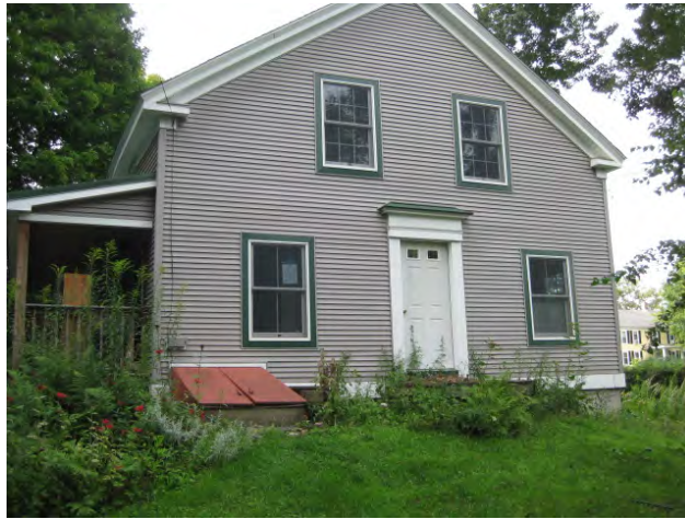
Figure 9. Pre-retrofit Belchertown Cape
