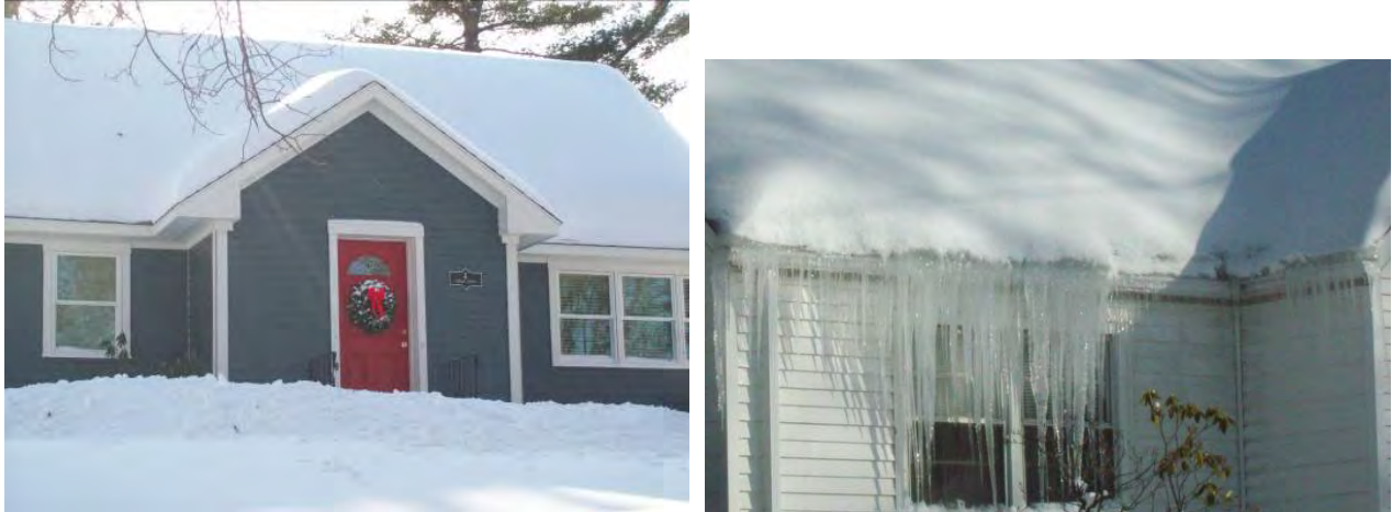
Figure 43. Left: Post-retrofit Millbury Cape; Right: Neighbor’s home with ice dams
