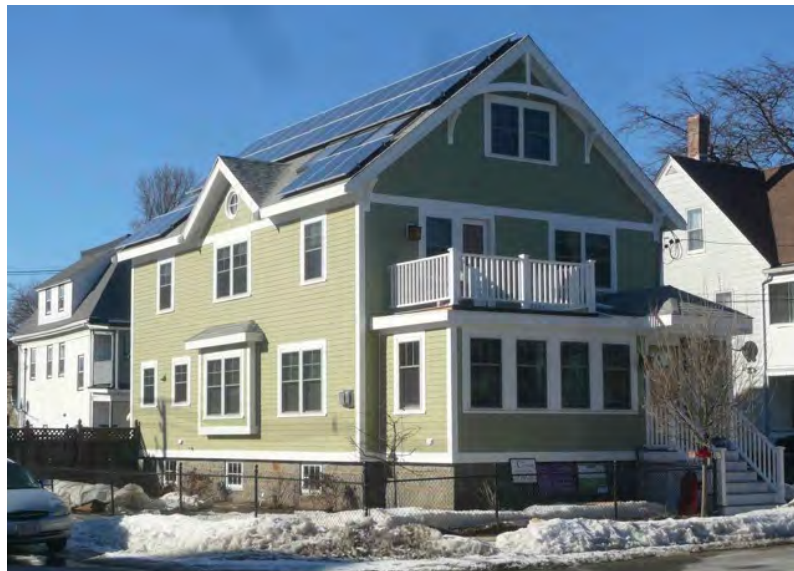
Figure 15. Post-retrofit Quincy Bungalow
