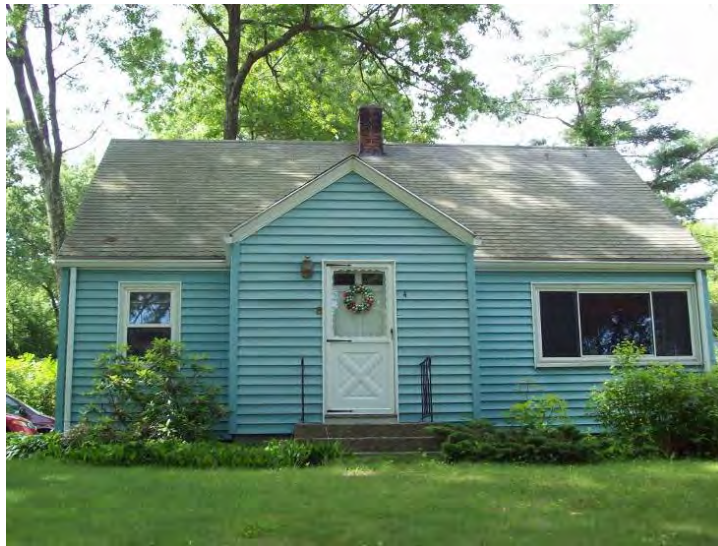
Figure 16. Pre-retrofit Millbury Cape
