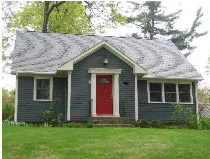
Figure 17. Post-retrofit Millbury Cape
