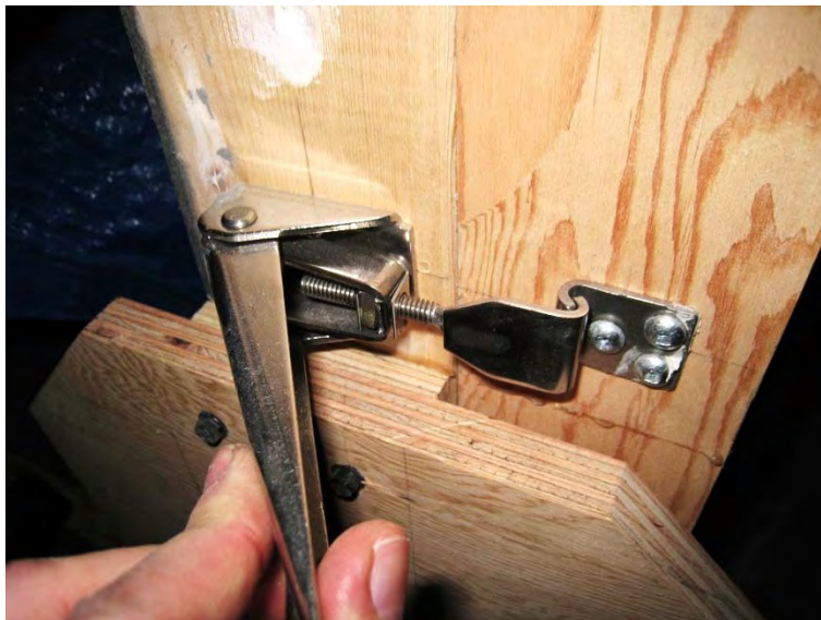
Figure 12 – Under-center draw latch and keeper (i.e. catch plate) at perimeter of panels (typ. of 8)
