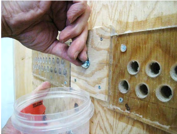
Figure 59 – Removing the wing nuts (qty of 14) from the field of the back panel
