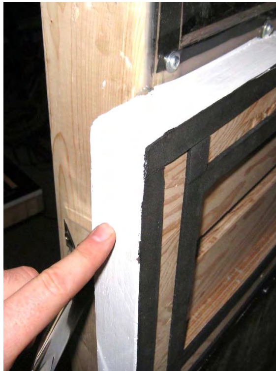
Figure 7 – Air seal coating applied to perimeter of flange
