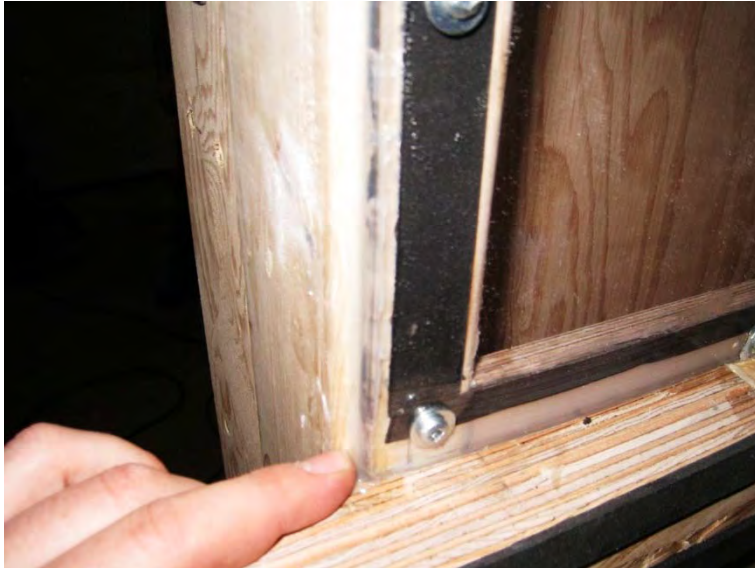
Figure 4 – Closed-cell foam gasket & wet seal around perimeter of polycarbonate sheet
