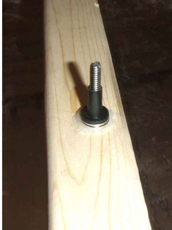
Figure 16 – 1/16” thick washer and tapered, sleeved rubber bushing to gap & seal plywood sheet
