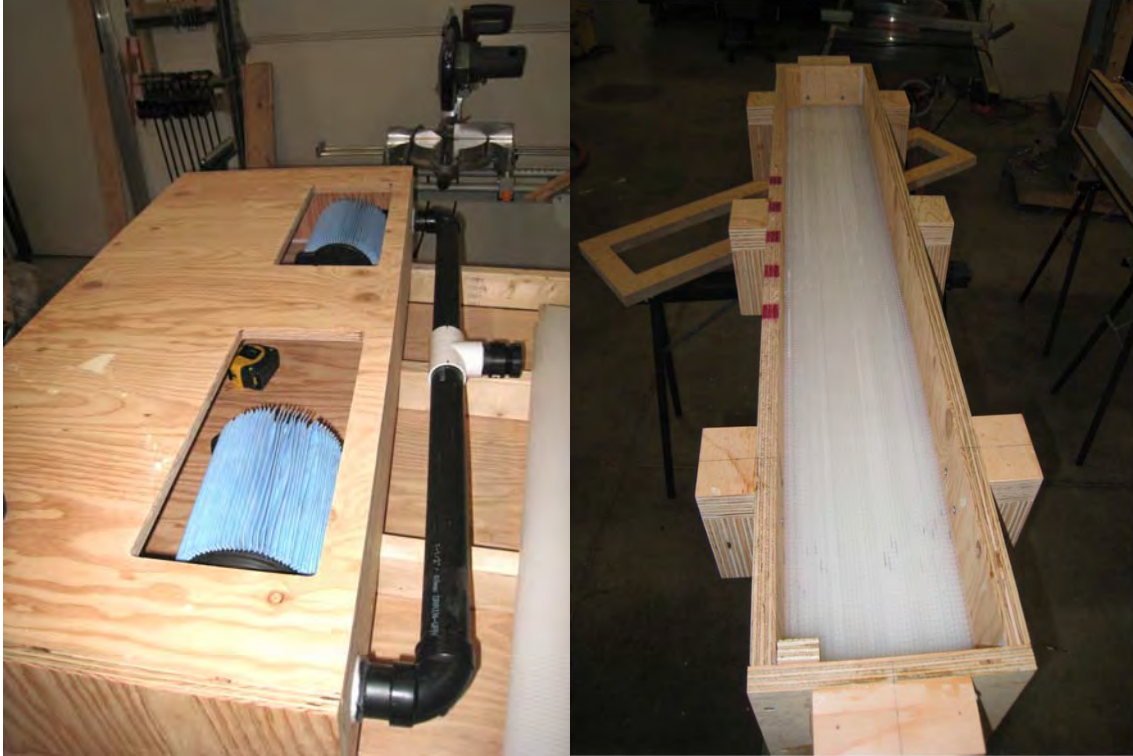
Figure 29 – Partially completed manifold with top installed (left) and latch blocks attached (right)
