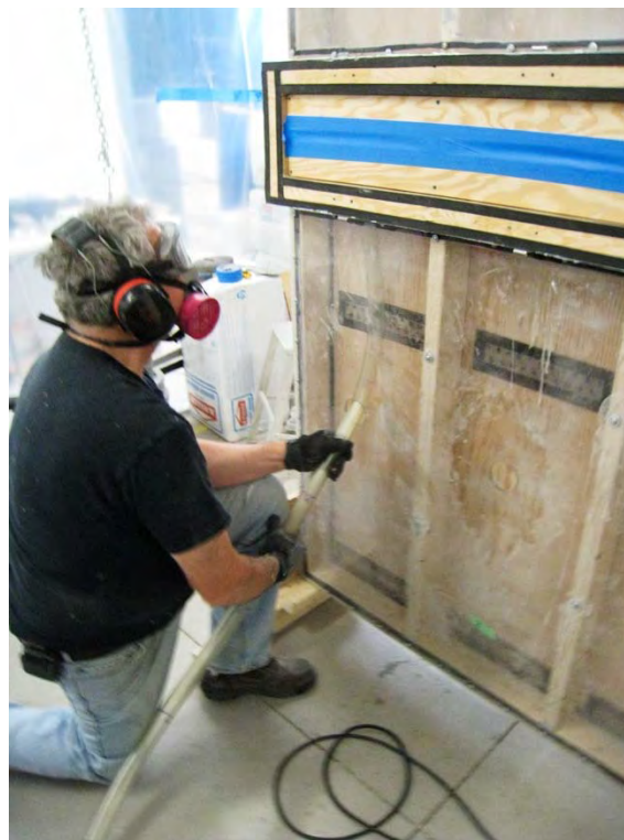
Figure 51 – Dense-packing the first stud bay
