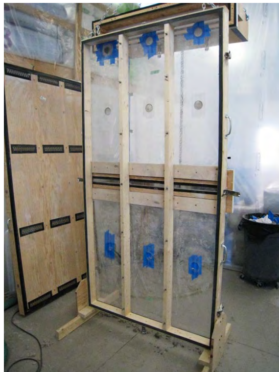
Figure 64 – Back & Front panels cleaned and ready for the next test specimen
