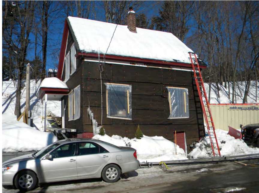
Figure 17. Pre-retrofit Colonial in Lancaster, Massachusetts
