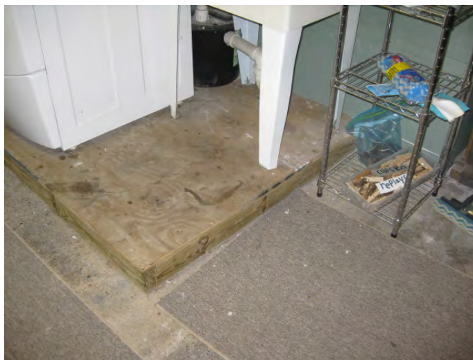
Figure 58. Equipment platform and shelving in basement of Test Home 2
