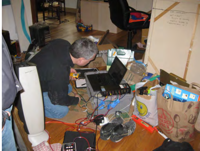
Figure 61. Post-DER guarded blower door testing at Test Home 3
