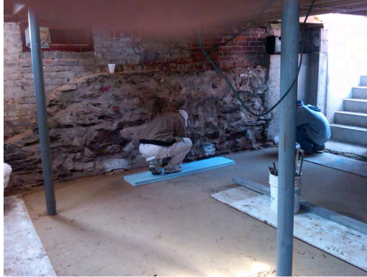
Figure 57. New basement slab and structural support at Test Home 5
