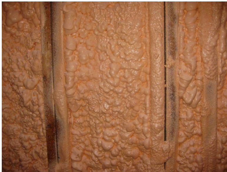
Figure 21. Airflow channels between double roof rafters at Test Home 1
