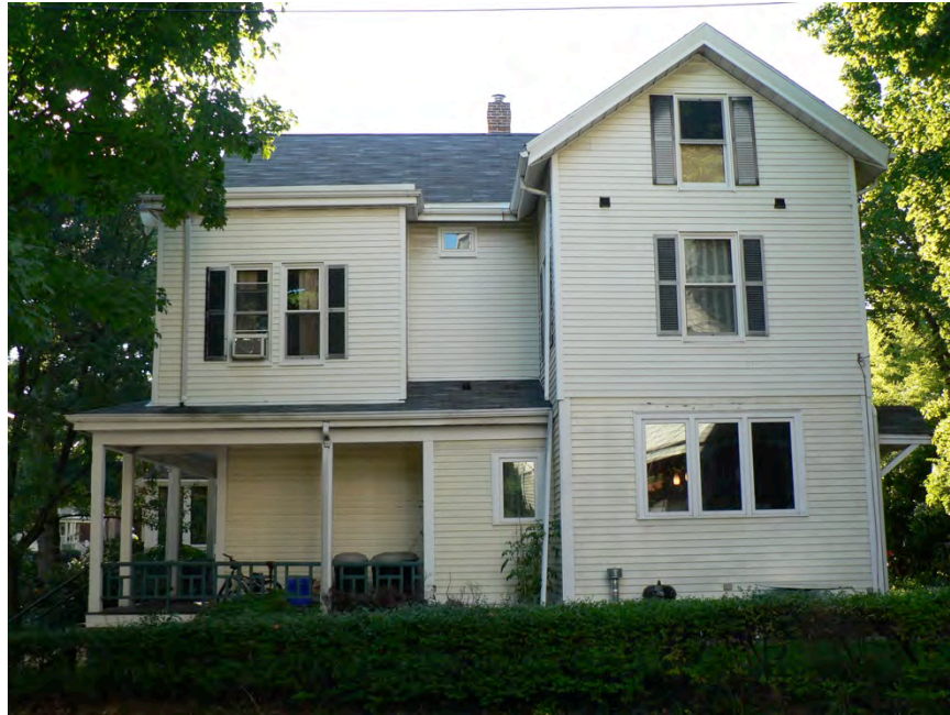
Figure 8. Pre-retrofit Victorian located in Brookline, Massachusetts
