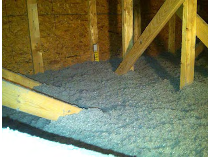
Figure 33. Loose-blown insulation in vented attic at Test Home 5
