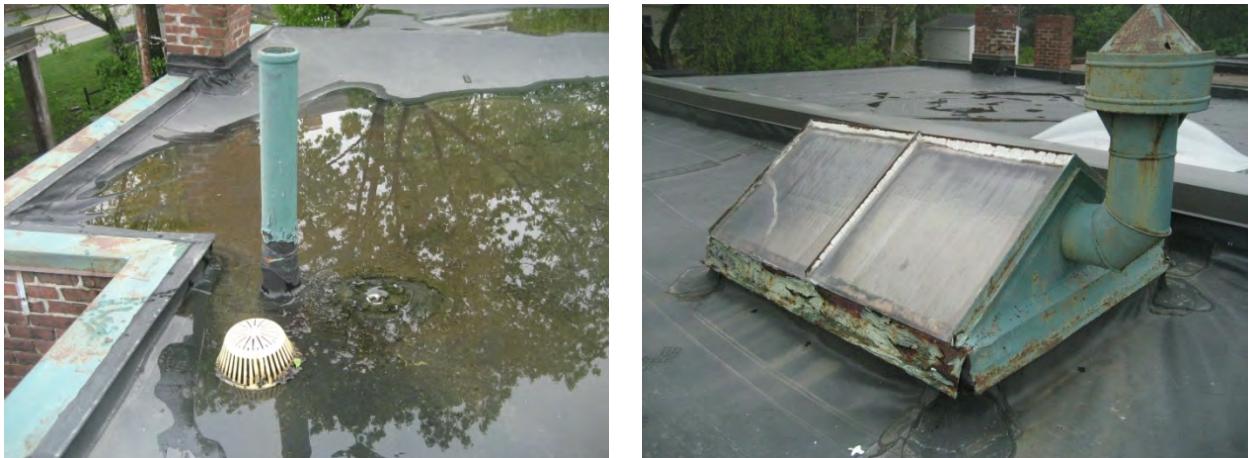
Figure 23. Roof drain (left) and stairway skylight (right)
