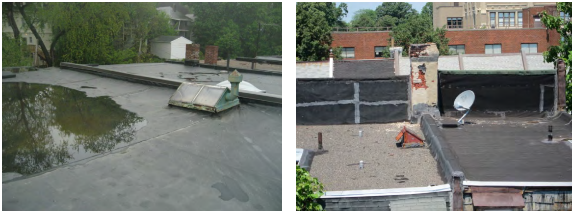
Figure 49. Capped party wall at J.P. Three-Family, and roof “wrap” over an exposed party wall
