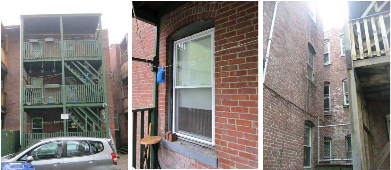
Figure 13. Rear building elevation (left), window detail (center), and light well area (right)
