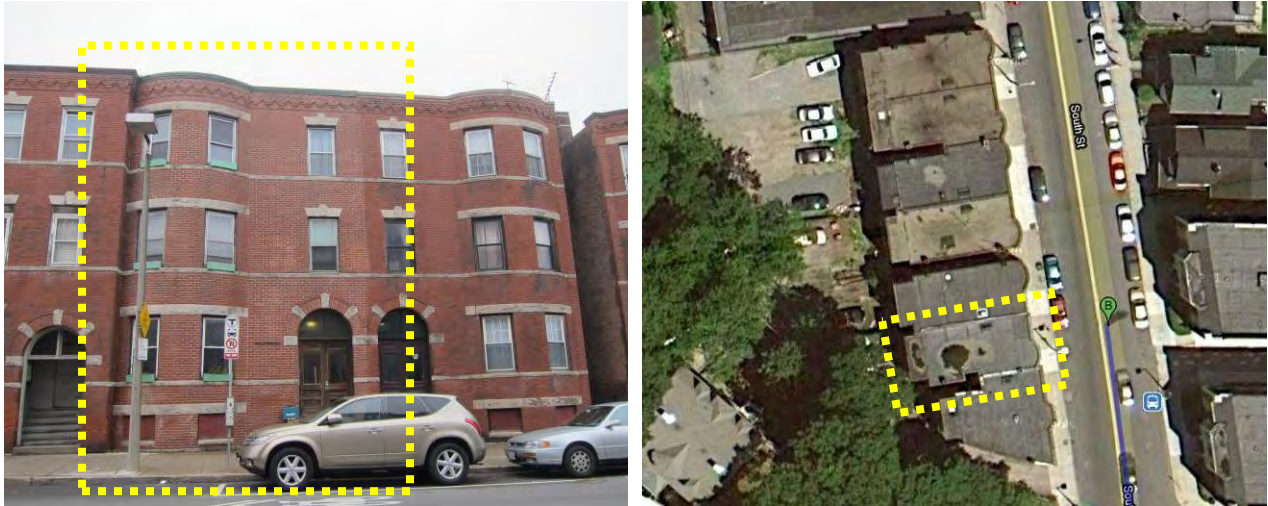
Figure 2. Exterior front and overhead view of masonry townhome project
