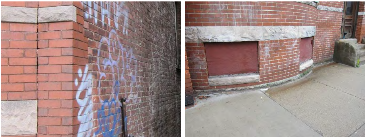
Figure 5. Front face brick/side brick transition (left) and brick termination at grade (right)
