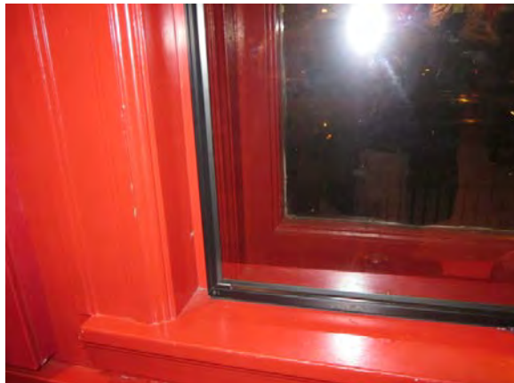
Figure 27. Interior storm window on double-hung original window
