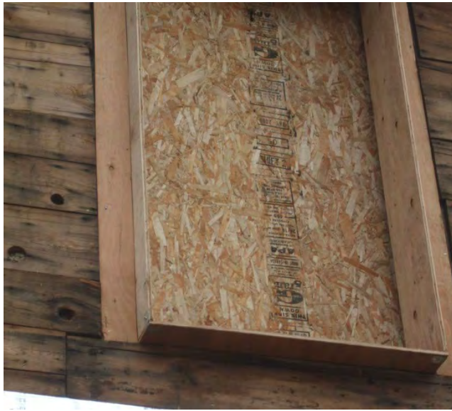
Figure 34. New window rough opening framed with and extension box to allow for the addition of exterior insulation
