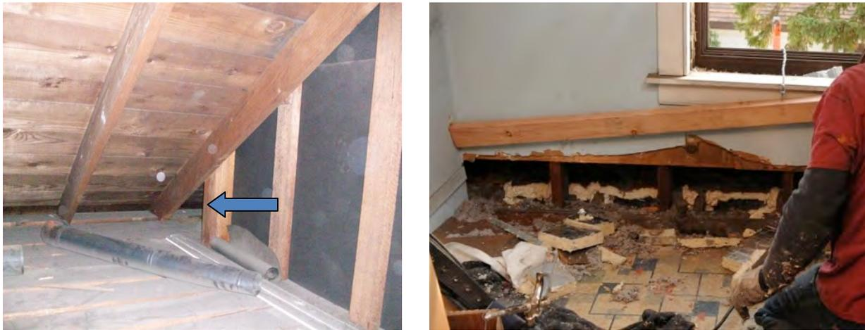
**Figure 21. Left: Small space with limited access at face of dormer. Right: section of interior finish removed to allow air sealing (Photo credit: E. Haber, printed with permission)**
