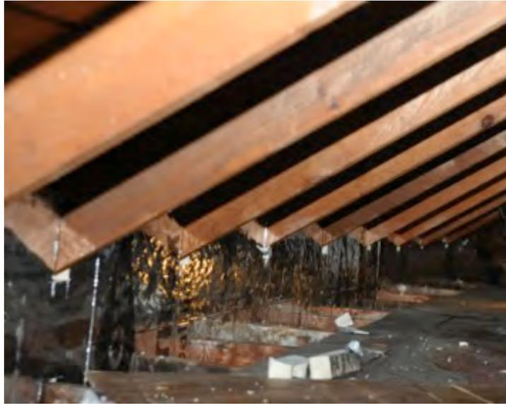
**Figure 19. Foil-faced polyisocyanurate insulation notched around roof and ceiling framing** (Photo credit: E. Haber, printed with permission)
