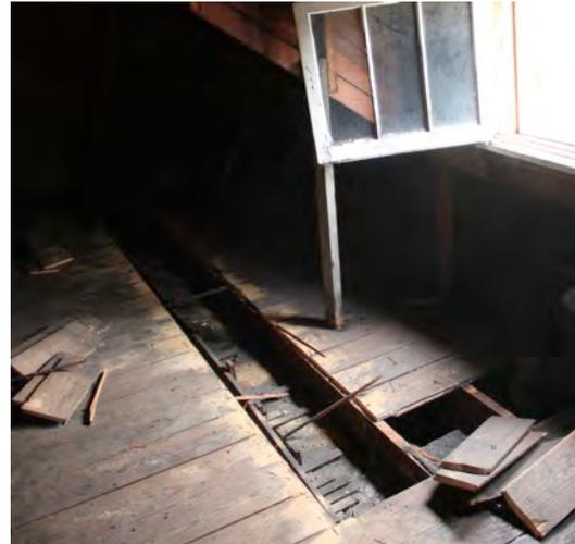
**Figure 18. Left: Workers cutting access to expose top of exterior wall and furring cavity; Right: Access cut to expose top of exterior wall and furring cavity at inset opening** (Photo credit: S. Marchese, printed with permission)
