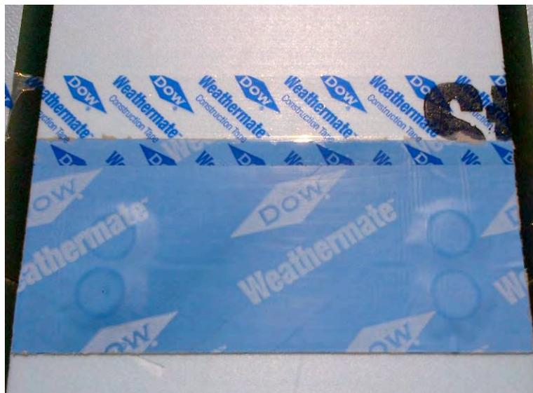
**Figure 14 – Example Termination Tape Offset High on Butyl Tape**
