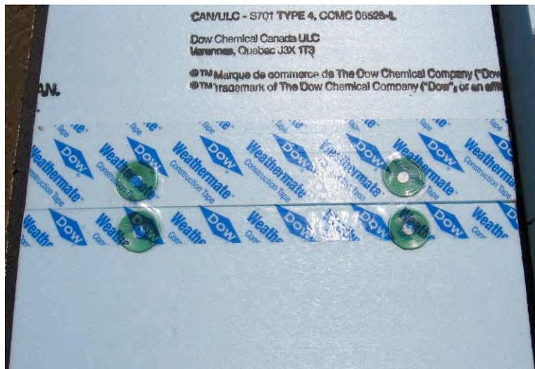
**Figure 15 – Example Wide Tape Intentionally Offset High**
