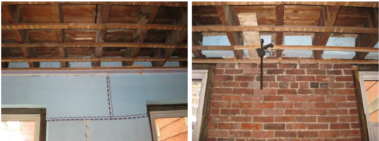
Figure 44: Rim joist foam blocks (left); close-up showing clamping jig (right)
