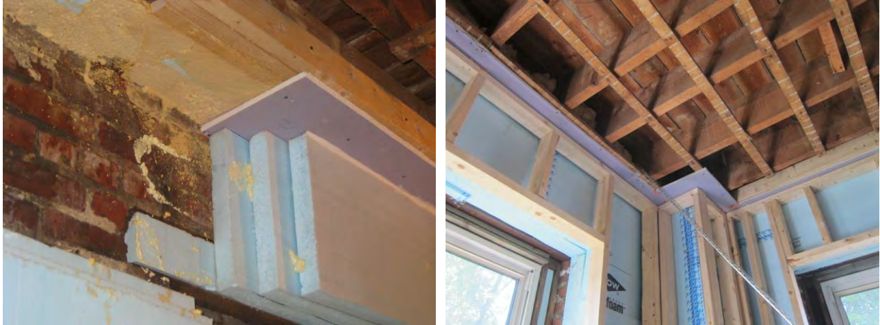
Figure 43: Floor/ceiling fire separation gypsum board (left); conditions after interior framing (right)
