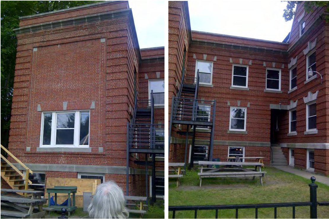
Figure 18: Addition - North Façade
