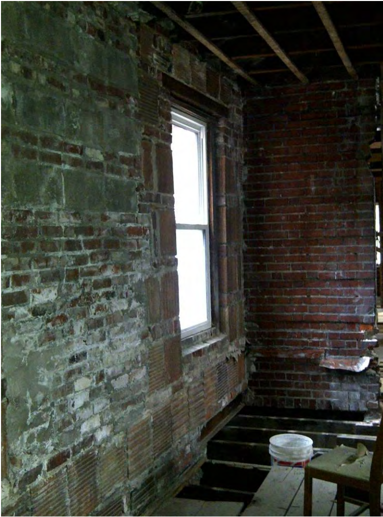
Figure 24: Addition - a typical window
