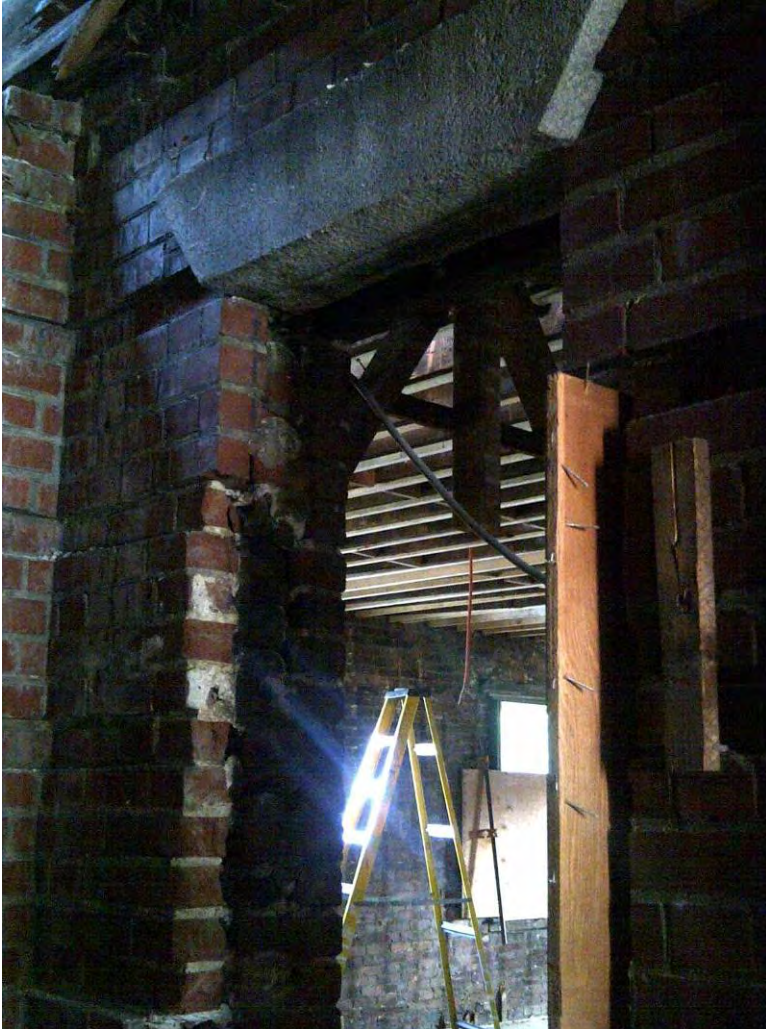
Figure 2: Original building – view of masonry wall section where doorway was shifted to interior
