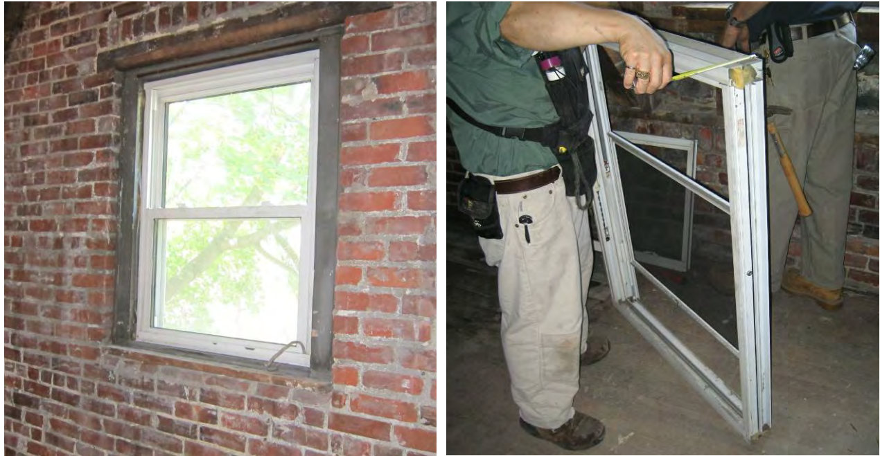
Figure 20: Existing vinyl double glazed (clear) insert replacement windows
