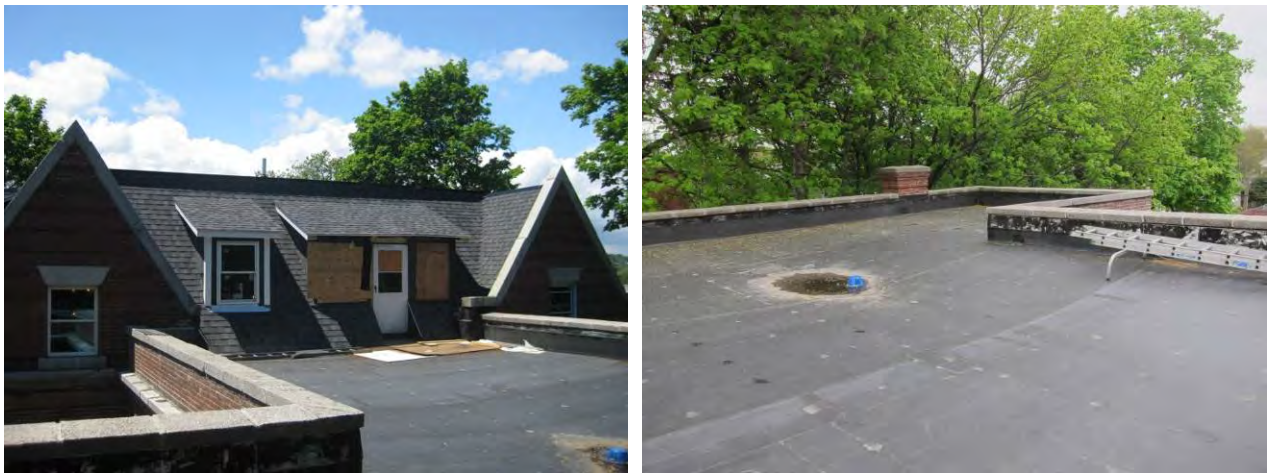
Figure 31: Lower roof, showing upper roof (left) and upper roof (right)
