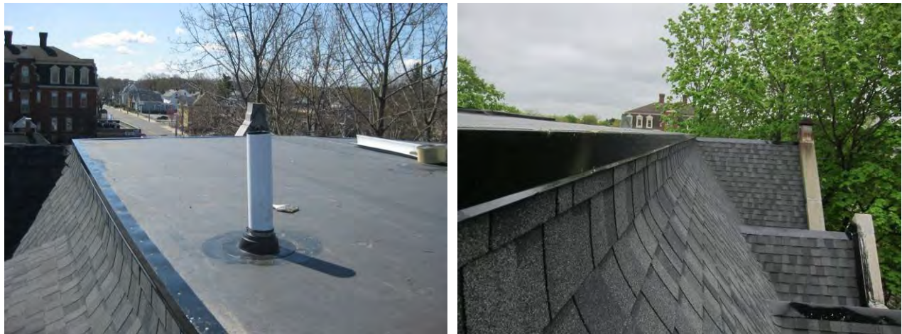
Figure 33: Upper roof typical conditions (left) and upper roof edge detail (right)
