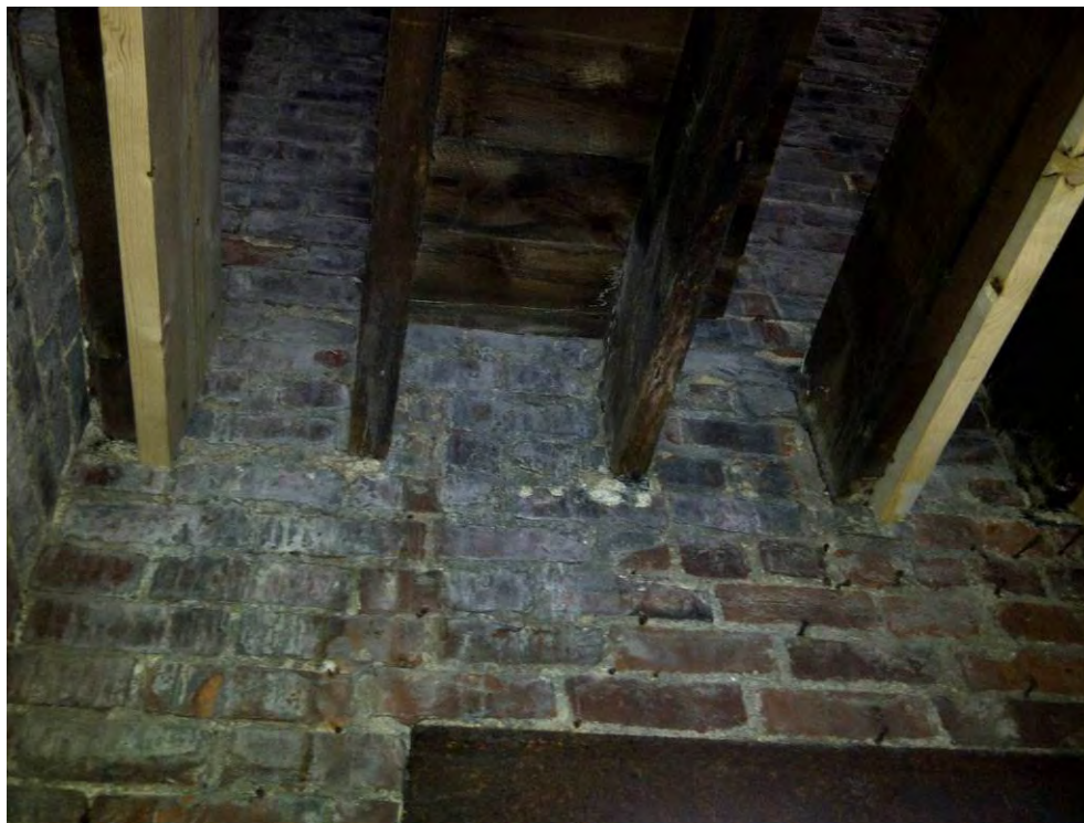
Figure 13: Floor joists set in masonry wall
