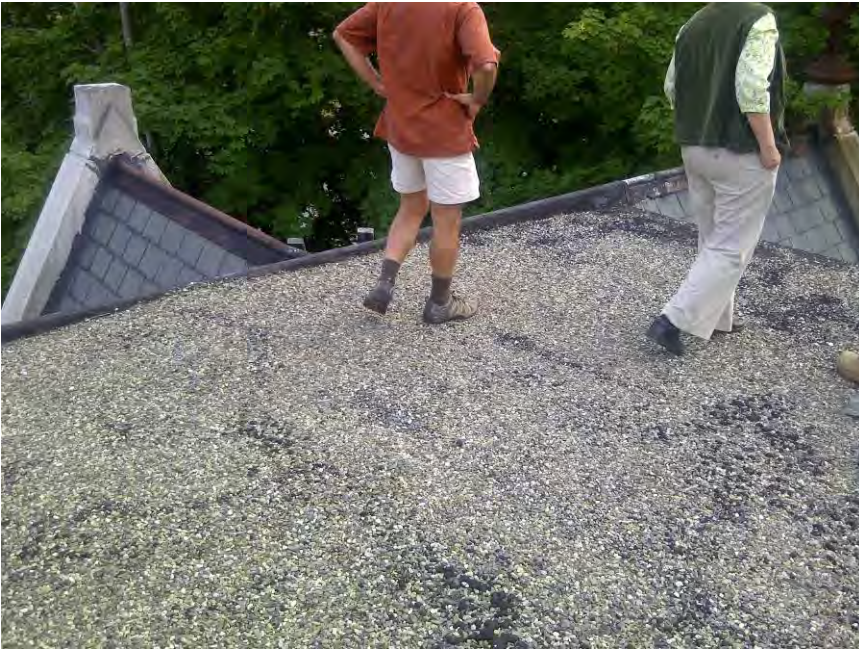
Figure 10: Original building – flat roof area
