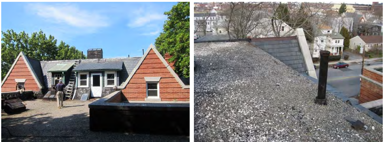
Figure 28: Lower roof, showing upper roof (left) and upper roof (right)
