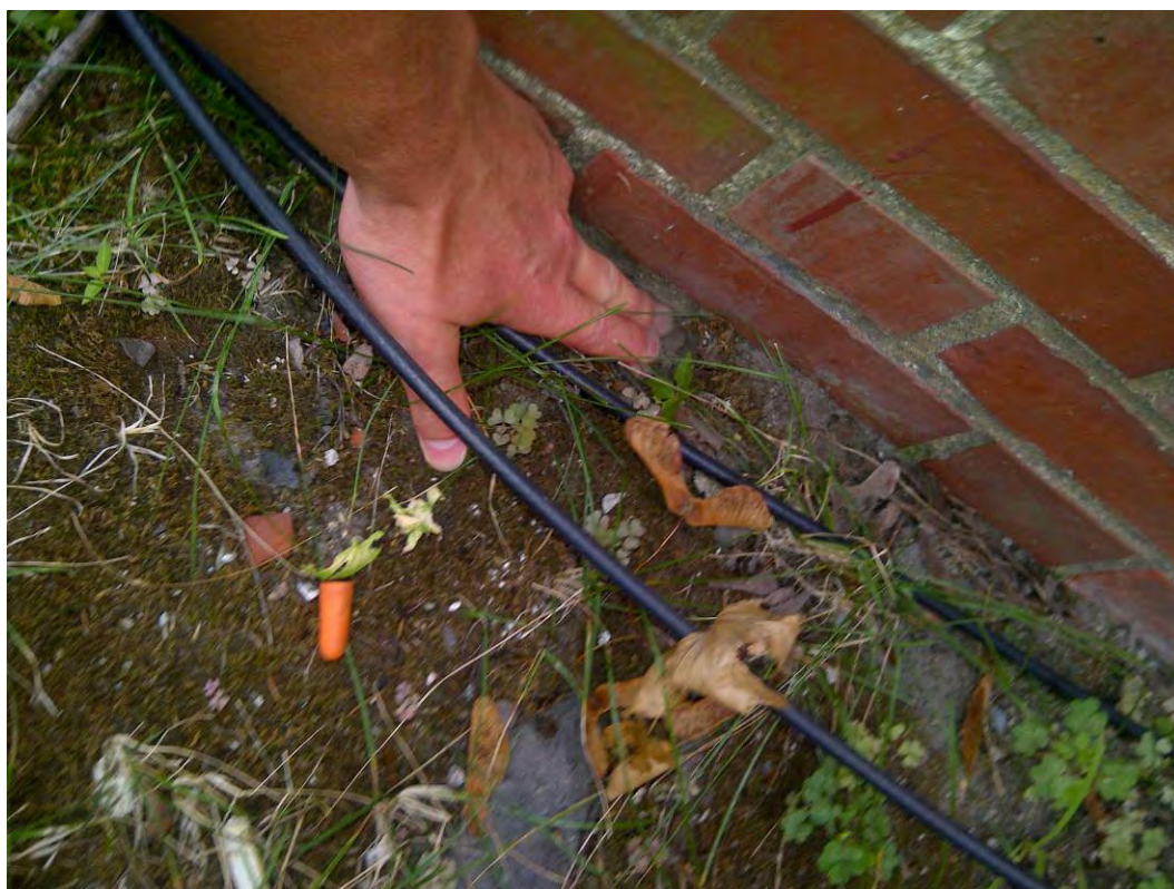
Figure 6: Original building – façade to ground interface
