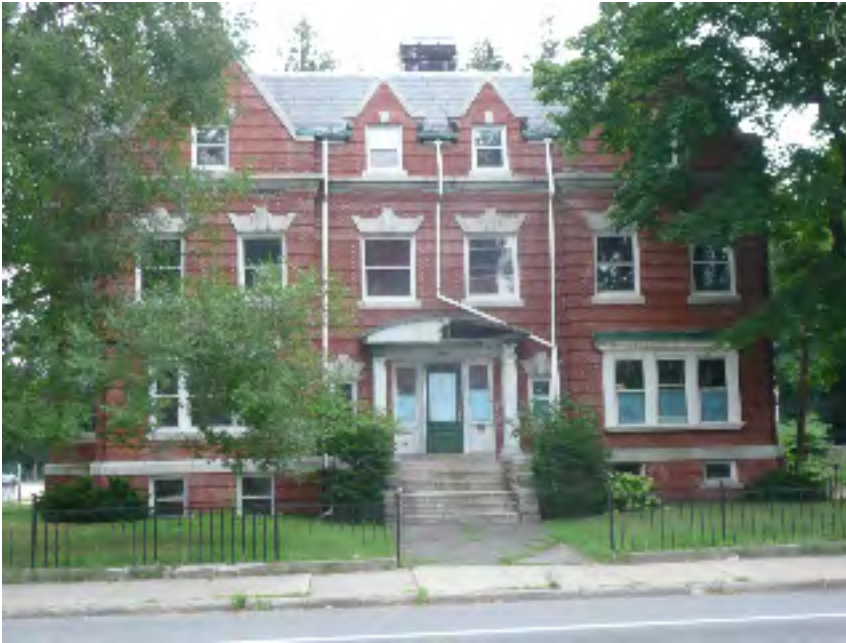
Figure 4: Original building – general view of building frontage.
