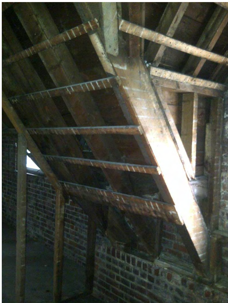
Figure 15: Original building – interior view of sloped roof
