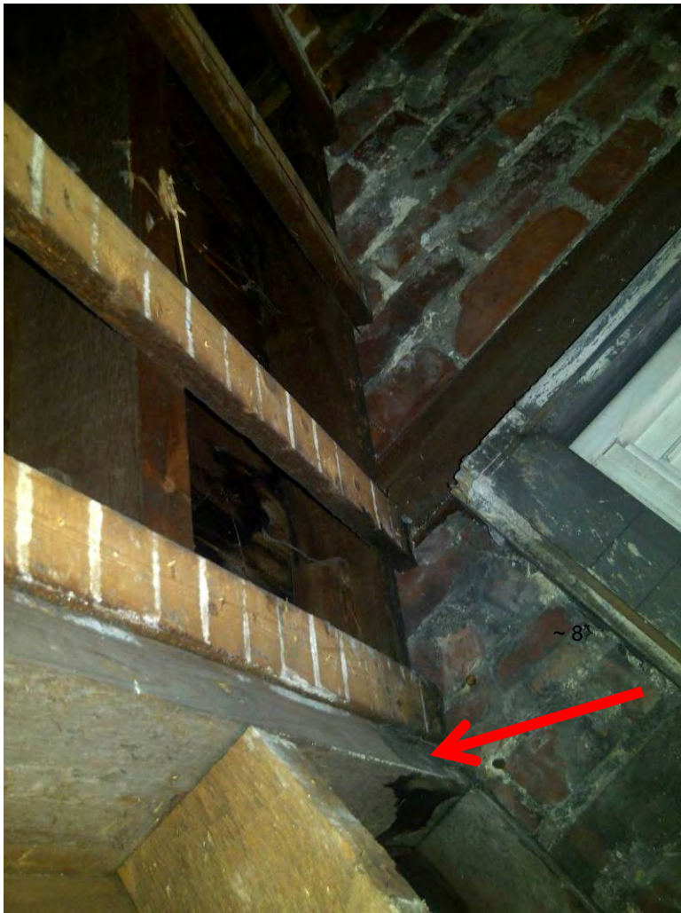
Figure 16: Original building – interior view of sloped roof
