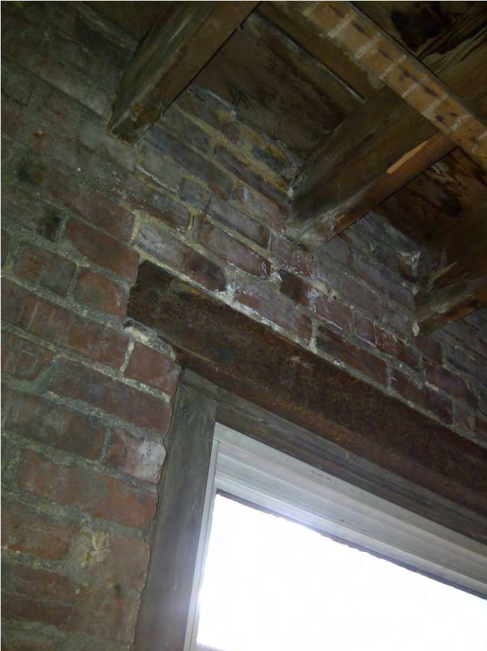
Figure 27: Addition – floor joists sitting in masonry and window
