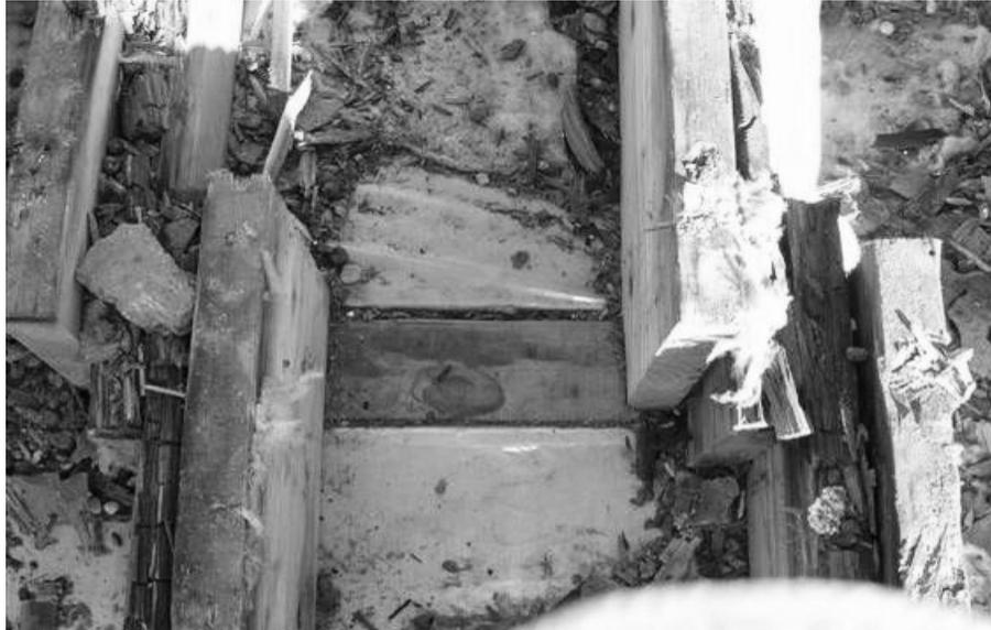
**Figure 10 – Air Leakage Resulted in Rot of Framing and Roof Deck in 2 Years (Fitzgerald 2010)**
