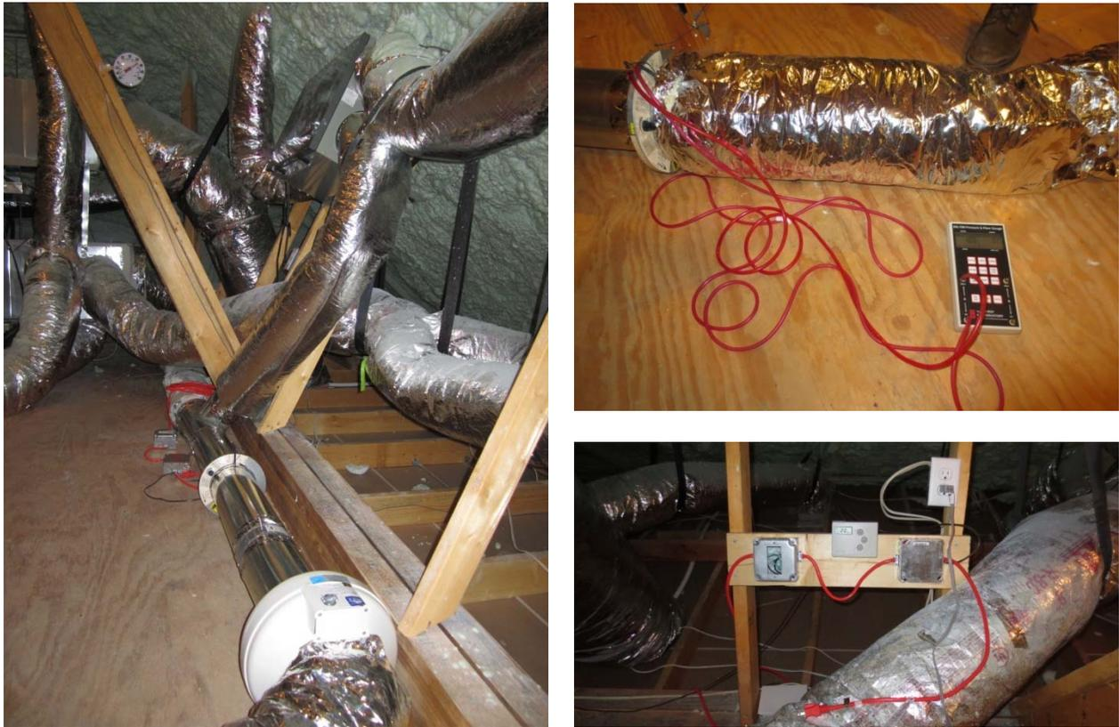
**Figure 9. Wye'd outside air duct, airflow stations, and inline fan for retrofitting a CFIS ventilation system in each attic (left); setting the CFIS airflow rate with Iris damper airflow station (top); fan timer and relay arrangement (bottom)**
