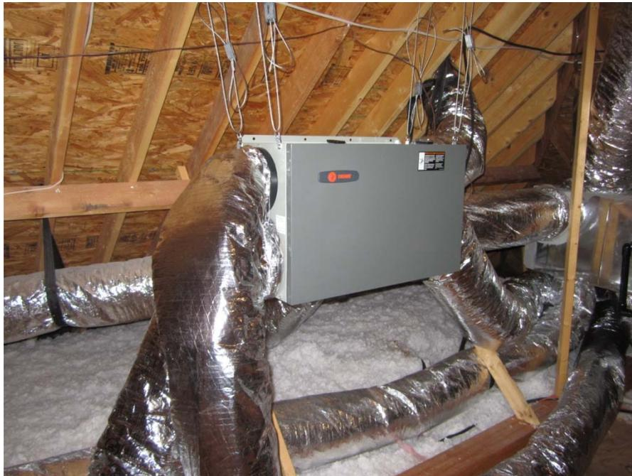
Figure 8. Energy Recovery Ventilator installed in House 1 to match that of House 2
