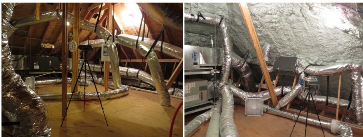
Figure 6. House 1 vented attic (left) and House 2 unvented attic (right)
