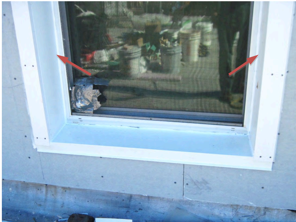
Figure 37. Return trim at the larger building butting into the vinyl window frame
