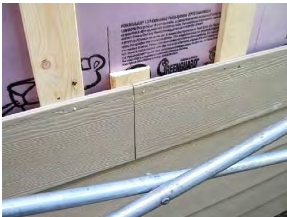
Figure 54. (L) Fiber cement lapped siding with fasteners at the top edge concealed by lap of subsequent piece; (R) fasteners for the panel cladding system exposed (Credit: Scott Sanders, CEDA)
