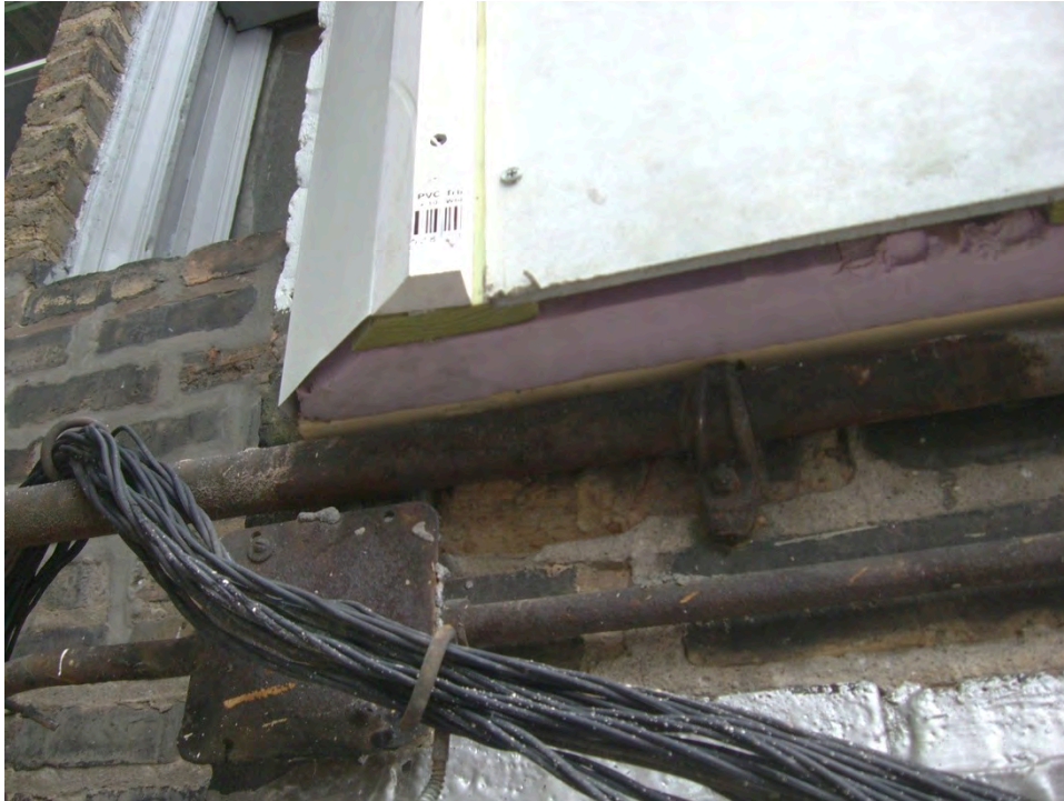
Figure 32. Base of wall with constricted access for attachment of screening (Credit: John Yi, CEDA)
