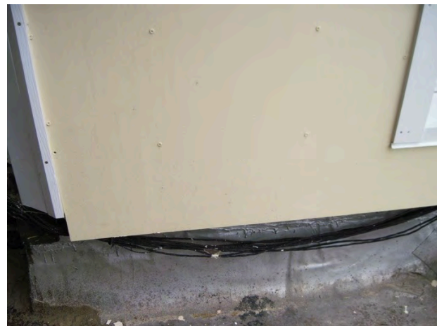
Figure 54. (L) Fiber cement lapped siding with fasteners at the top edge concealed by lap of subsequent piece; (R) fasteners for the panel cladding system exposed (Credit: Scott Sanders, CEDA)
