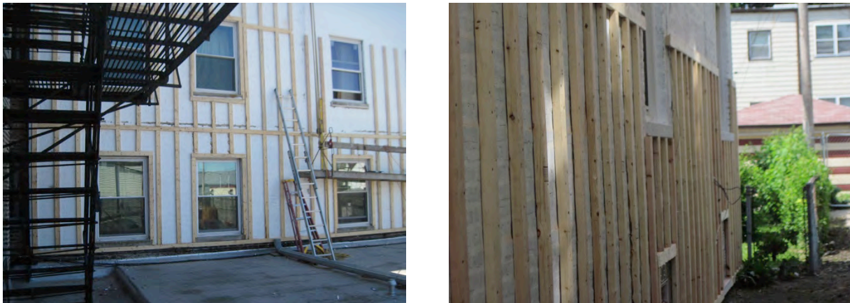
Figure 18. (L) Framing installed in a vertical orientation at 16 in. o.c. as well as horizontally at 8-ft increments in the field of the wall. Each window opening is also picture framed with the framing material; (R) Framing installed against masonry at two-family building with horizontal framing at top of window openings and at 8-ft vertical increments. (Credit: Scott Sanders, CEDA)
