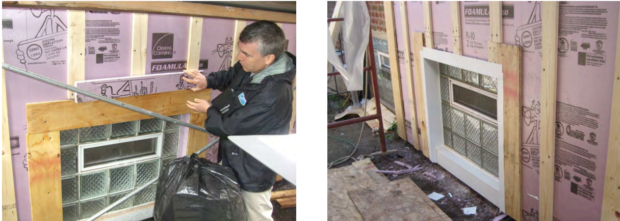
Figure 25. (L) BSC personnel explaining the attachment of trim to vertically oriented strapping; (R) the same window after the contractor reconfigured the strapping (Credit: John Yi, CEDA [L] and Scott Sanders [R], CEDA).
