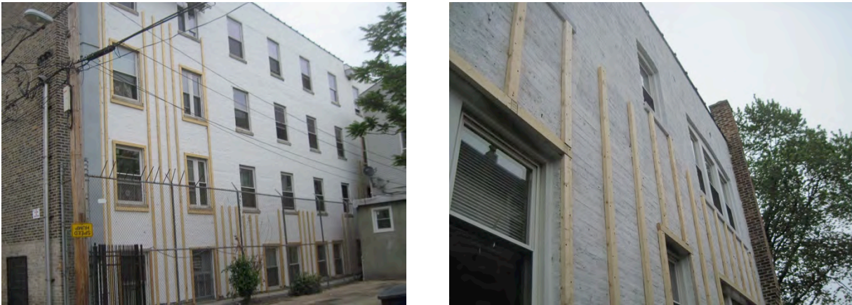
Figure 19. (L) Framing installed at in a vertical orientation only in the field of the wall. Each window opening is picture framed with the framing material. (R) Framing installed against masonry at two-family building with horizontal framing at top of window openings but in a vertical orientation elsewhere. (Credit: Scott Sanders, CEDA)
