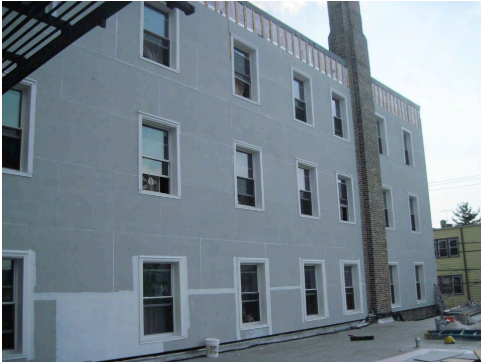
Figure 51. Caulked butt joints between 4 × 8 panels
