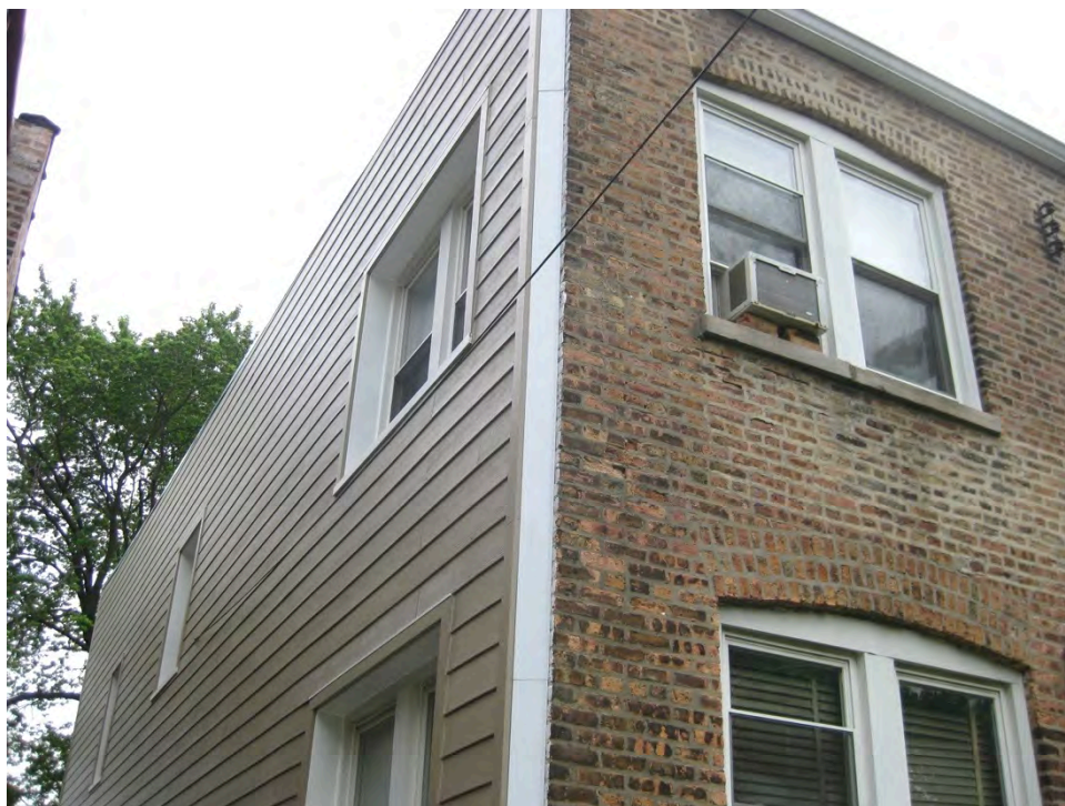
Figure 49. Treated wall at the smaller building striking a contrast with the untreated wall at the rear of the building
