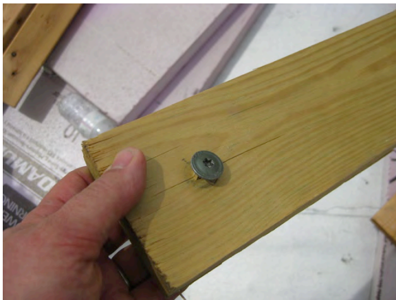
Figure 24. (L) Wood strapping with fastener used for attachment through rigid foam insulation to 2 x 4 framing; (R) longer size fasteners used to attach strapping through thicker rigid foam insulation layer at parapet
