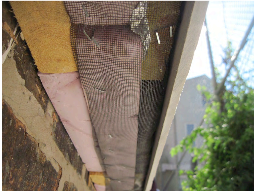
Figure 62. Screening at the base of the wall that fails to protect the exposed edge of the insulating sheathing near grade (Credit: Scott Sanders, CEDA)
