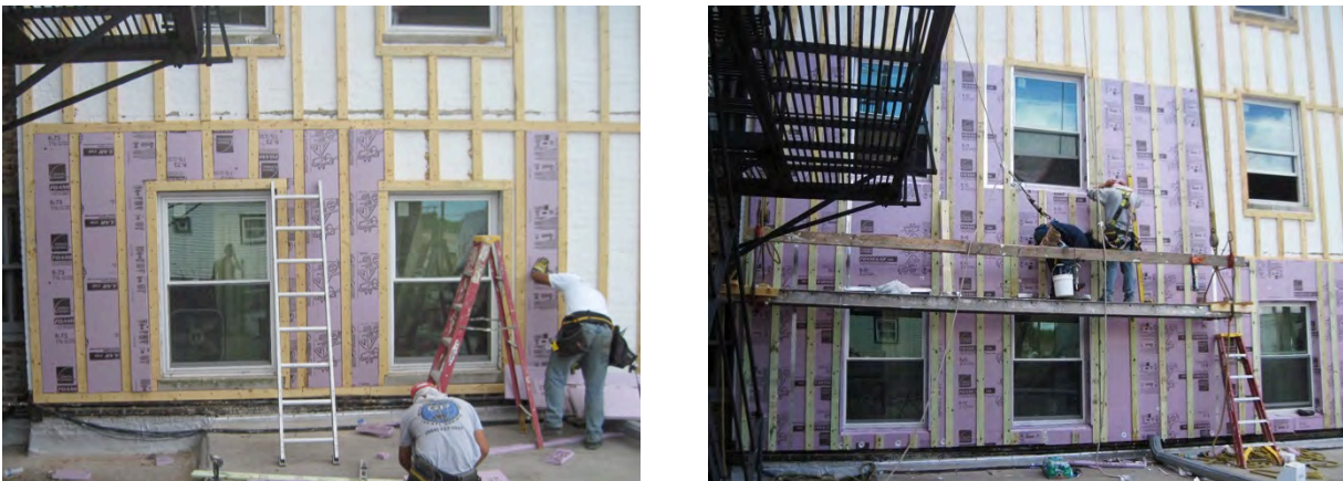
Figure 21. (L) Crews installing rigid insulation between furring; (R) second layer of rigid insulation installed over same section of wall as shown at left. Photo taken 1½ hours after photo at left. Finished first floor insulation extends another three window bays to the right of the image. (Credit: Scott Sanders, CEDA)
