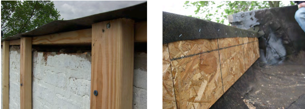
Figure 27. (L) Contractors mock up of frame over parapet using 2 × 12 attached to vertical furring attached to face of wall; (R) OSB attached to 2 × 12 at inside face of parapet. (Credit: John Yi, CEDA)
