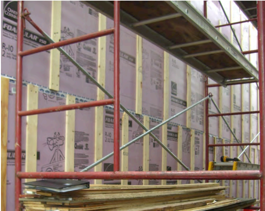
Figure 20. Strapping over insulating sheathing showing switch from 16 in. o.c. to 24 in. o.c. at the two-family building (Credit: John Yi, CEDA)
