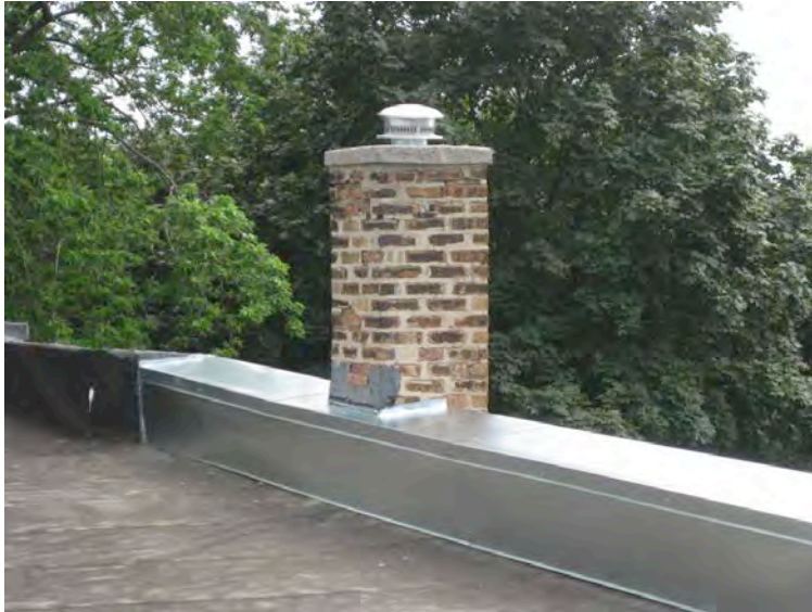
Figure 29. Finished parapet cover at two-family building
