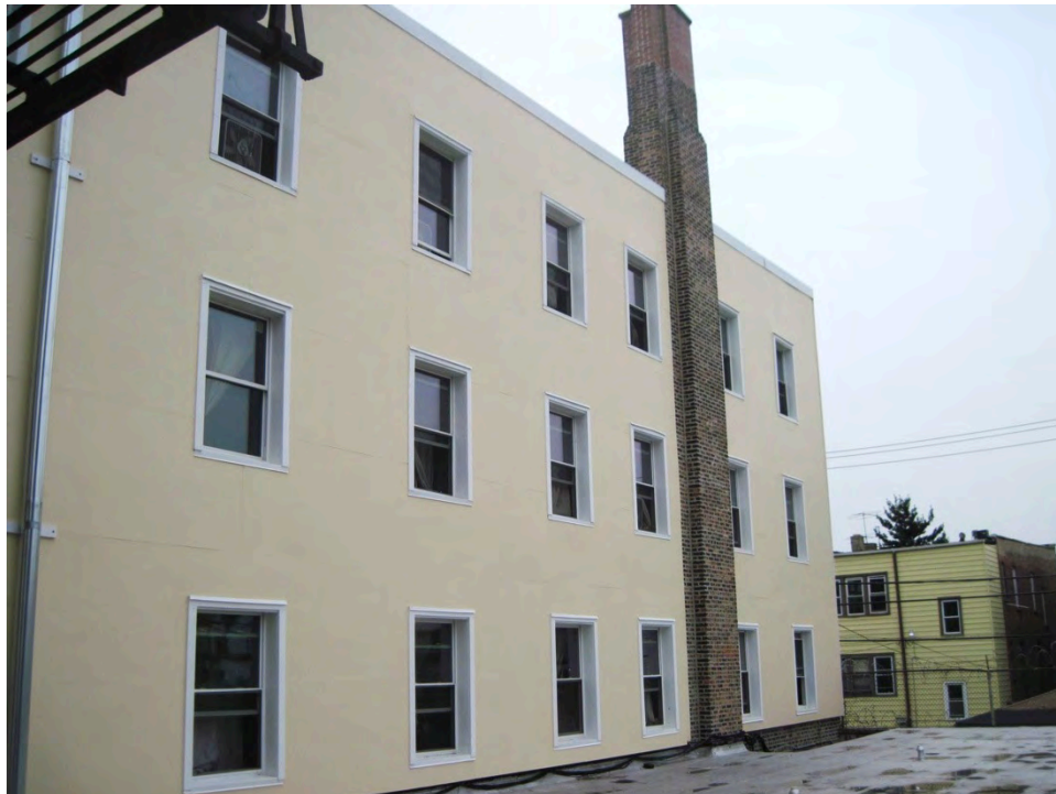
Figure 48. Finished side of the larger building
