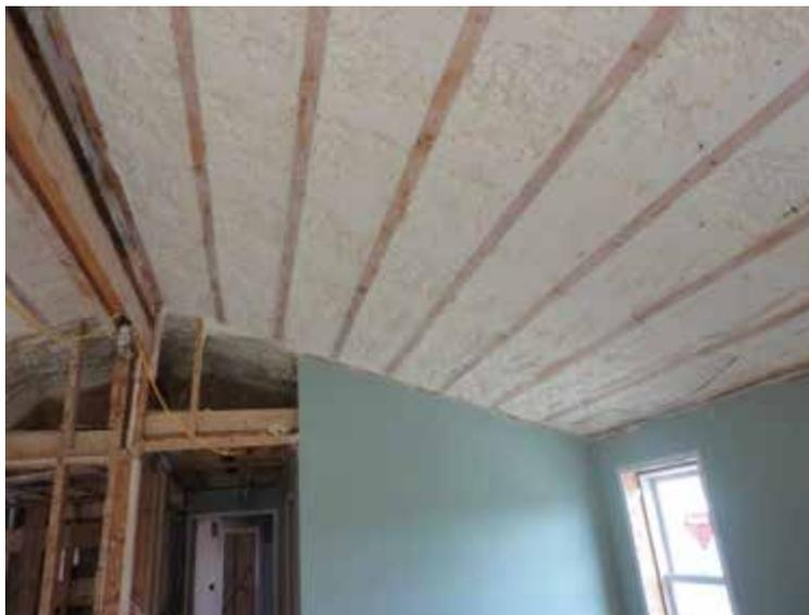
**Figure 2. Spray foam insulation used for air control in rafter cavities (with cross strapping)**
