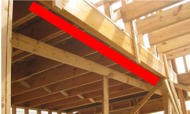
Figure 28. Plan 4069 first floor kitchen “raceway” location
