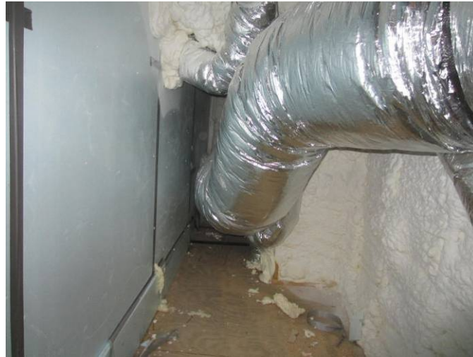
Figure 20. Plan 4128 return duct in knee wall
