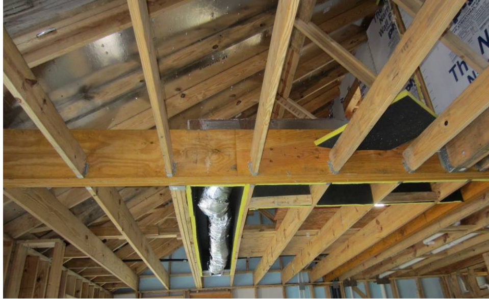
Figure 22. Plan 4128 dining room duct coffer
