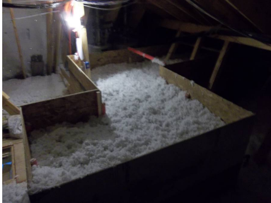
Figure 26. Plan 4069 insulation trough
