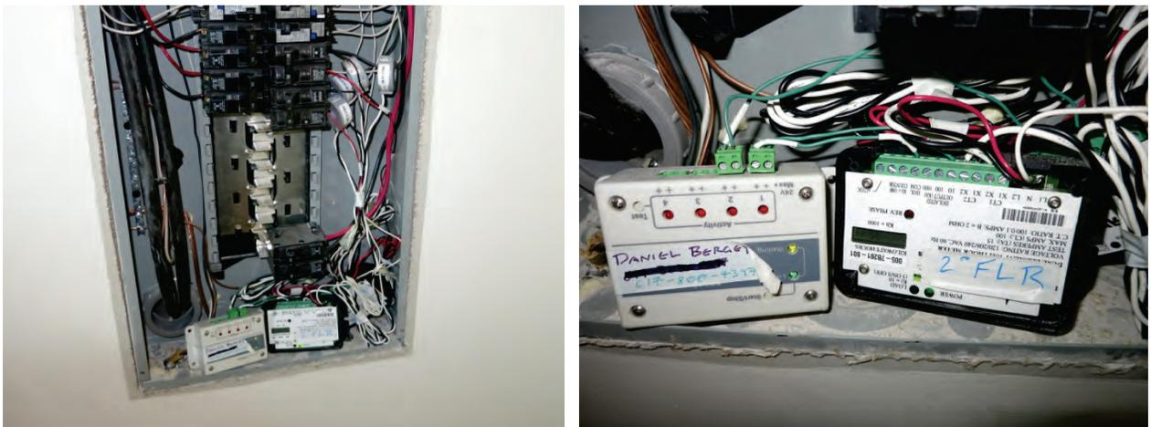
Figure 17. MSHP electrical power monitoring at electrical panel
