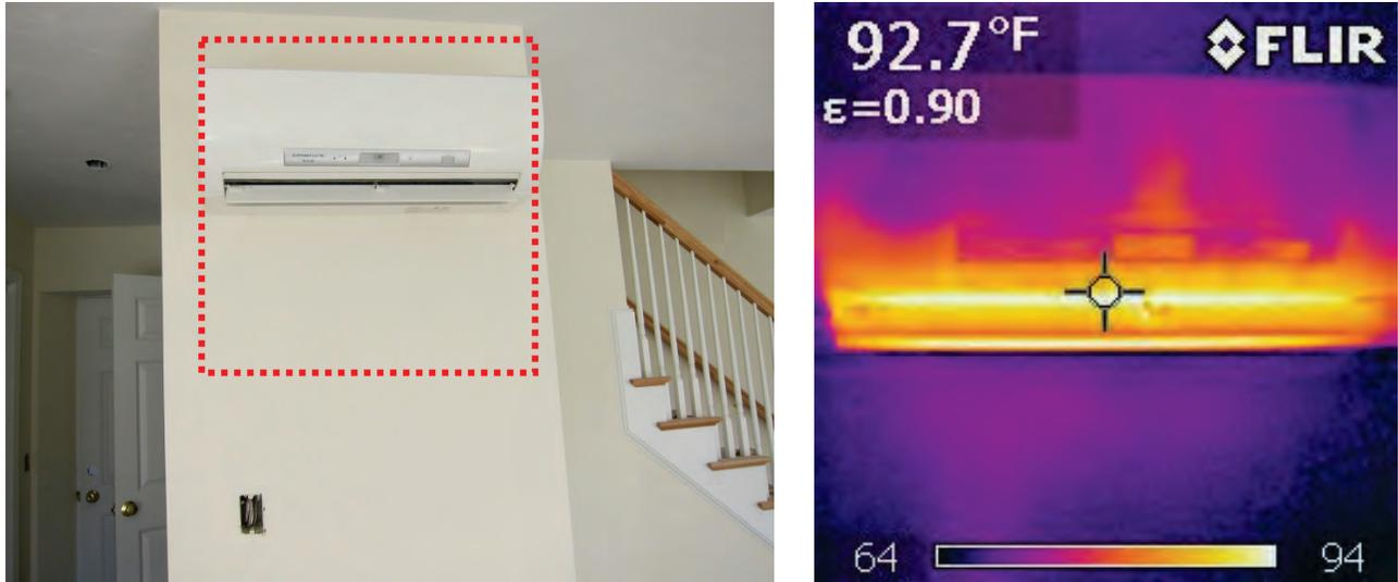
Figure 7. Indoor MSHP unit in heating mode, showing delivery temperature
