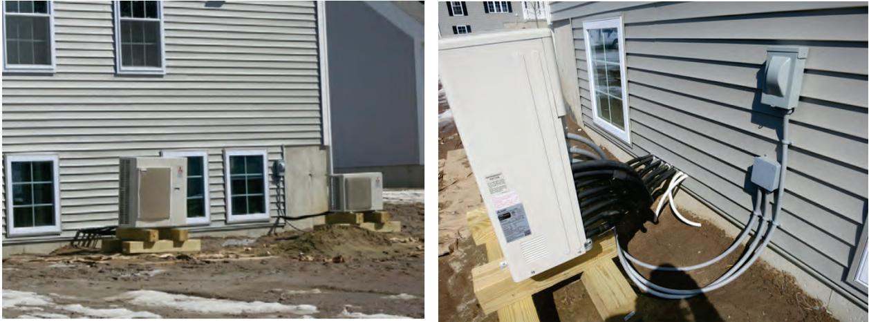
**Figure 9. 3:1 multi-split DHP (Mitsubishi MXZ series) installed at Easthampton**
