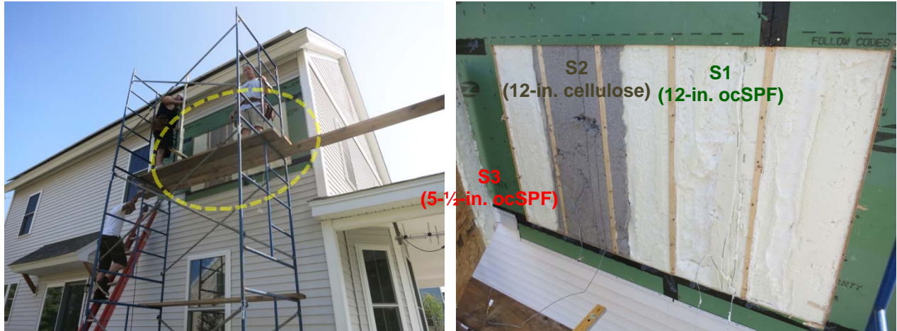
Figure 39. South-facing wall disassembly, showing test bay cavities
