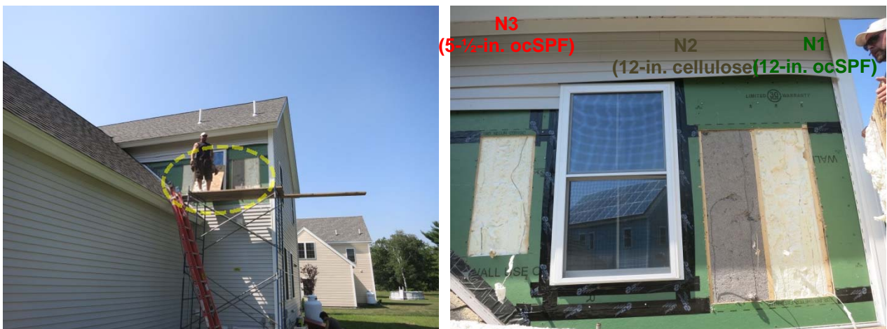
Figure 42. North-facing wall disassembly, showing test bay cavities
