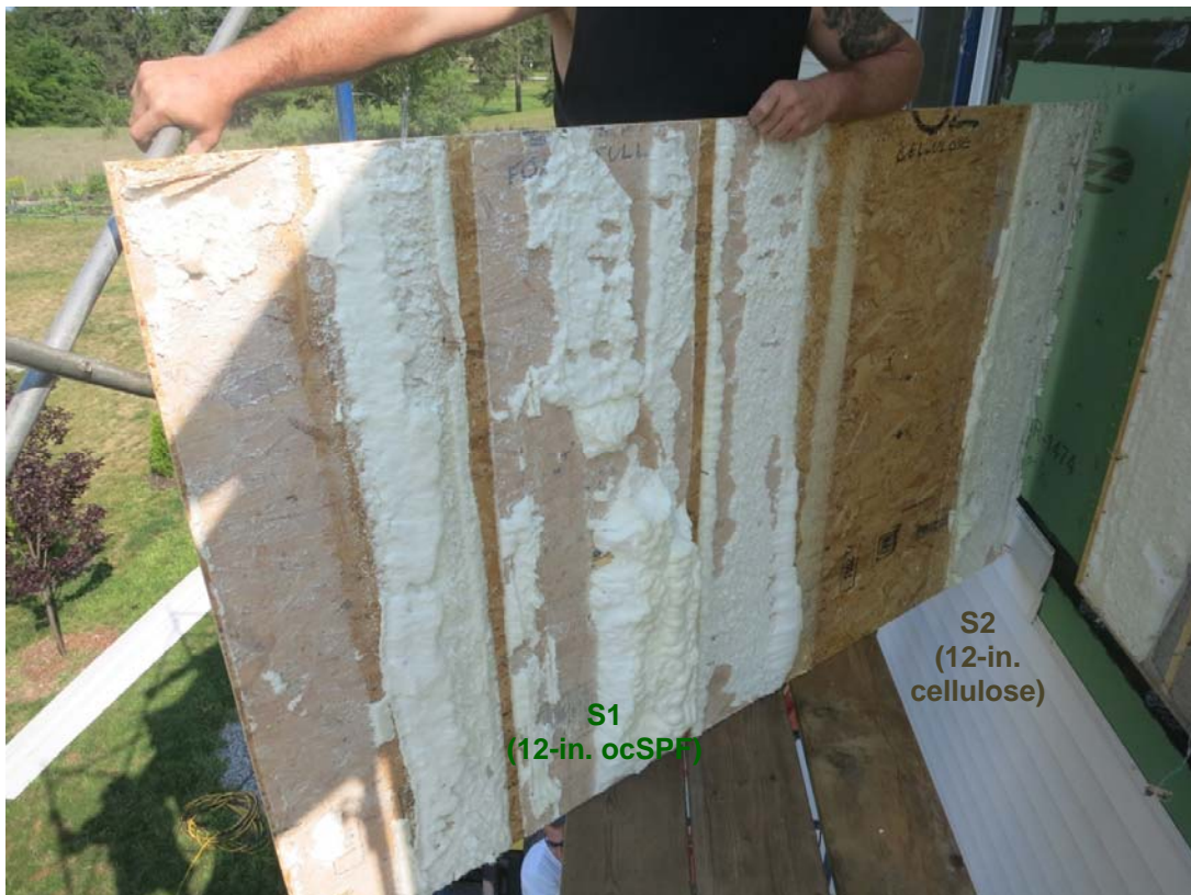
Figure 40. South-facing wall sheathing conditions
