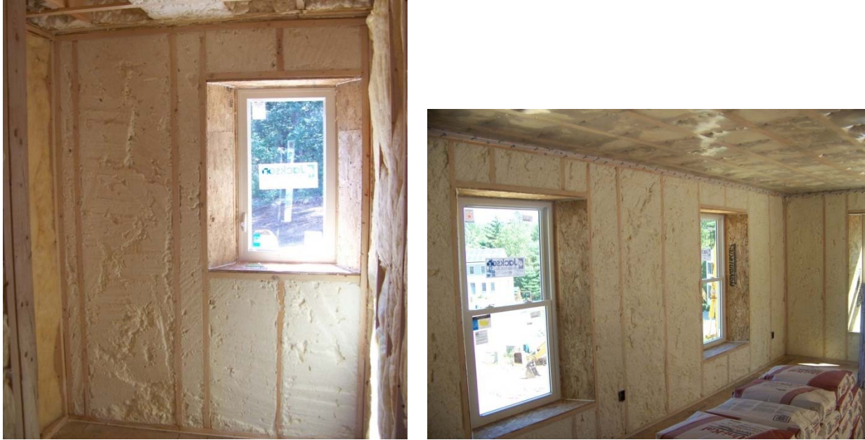
Figure 2. Typical installation of 0.5 lb/ft 3 (PCF) ocSPF in double-stud walls
