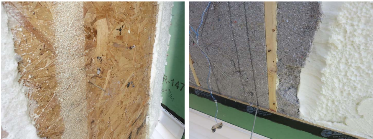
Figure 41. Sheathing and framing conditions at south-facing walls
