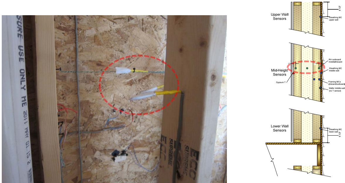
Figure 27. Stud bay cavity T/RH sensor locations
