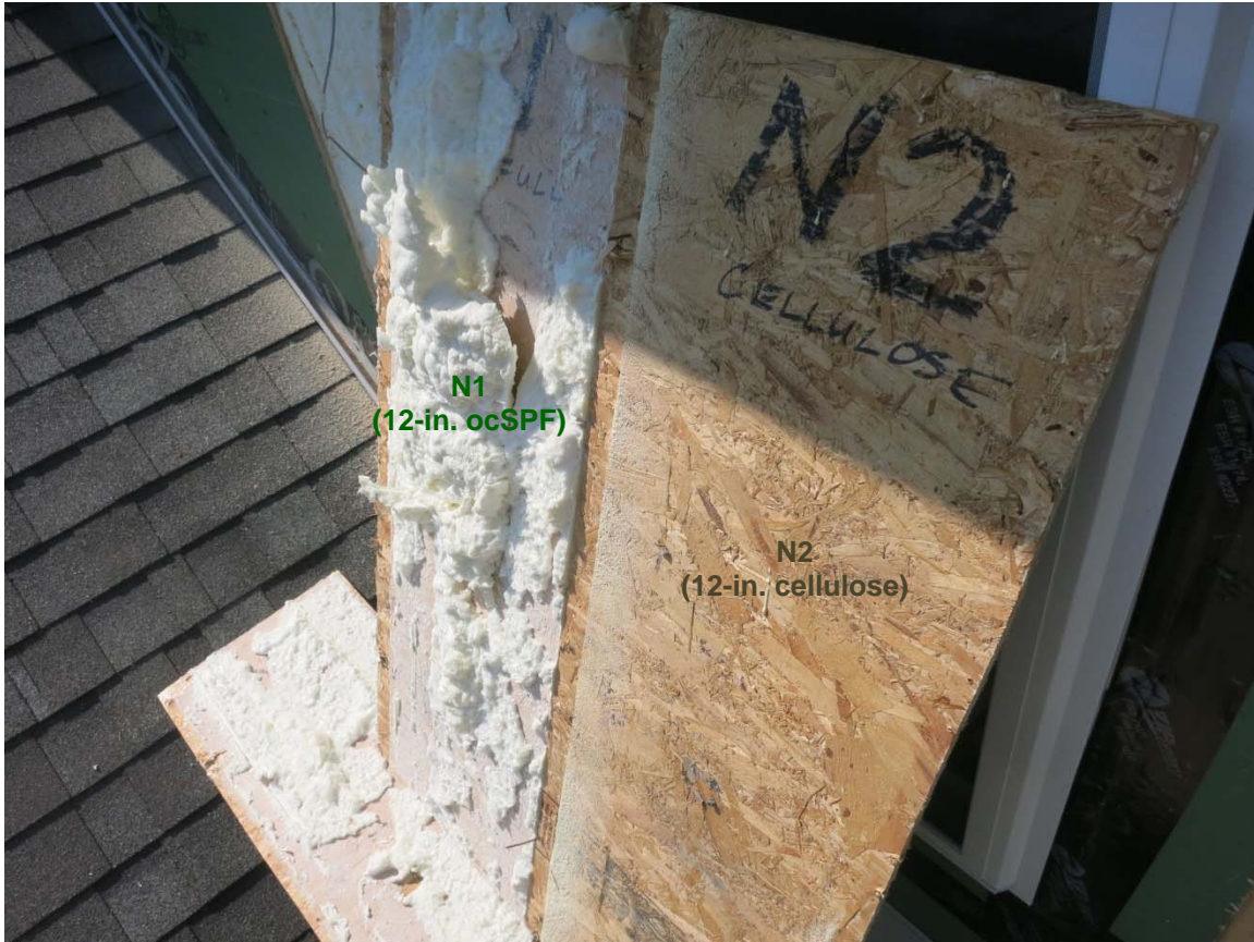
Figure 43. South-facing wall sheathing conditions (12-in. ocSPF/N1 and cellulose/N2)
