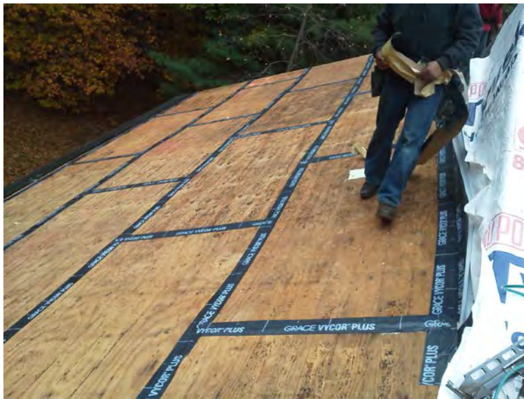
Figure 6. Taped wood panel roof sheathing as air control membrane
