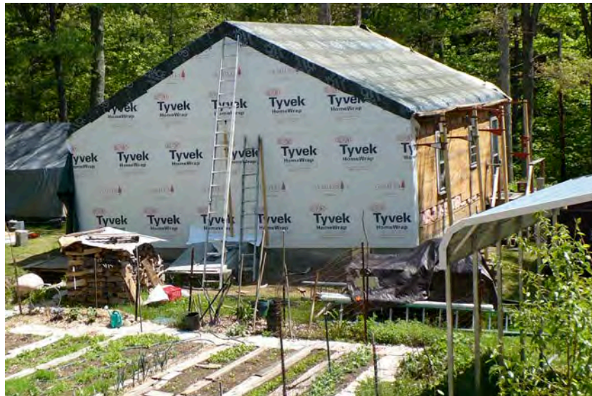
Figure 8. “Chainsaw” transition of air and water control membrane at rake
