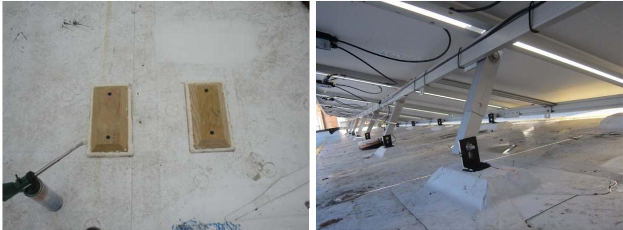
**Figure 21: PV system rack attachment during construction (left) and completed (right)**
