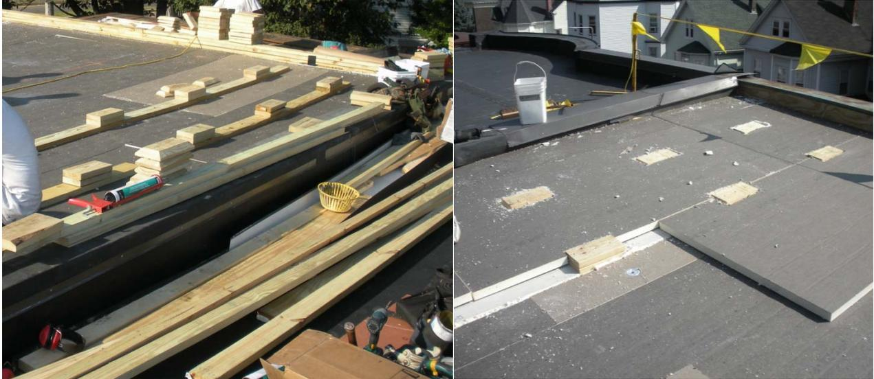
**Figure 19: Blocking for future PV installation**
