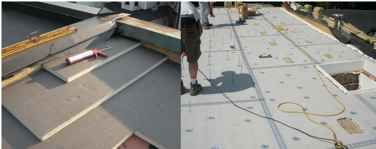
**Figure 18: Rigid insulation in multiple layers with staggered seams (left); insulation cover board (right)**
