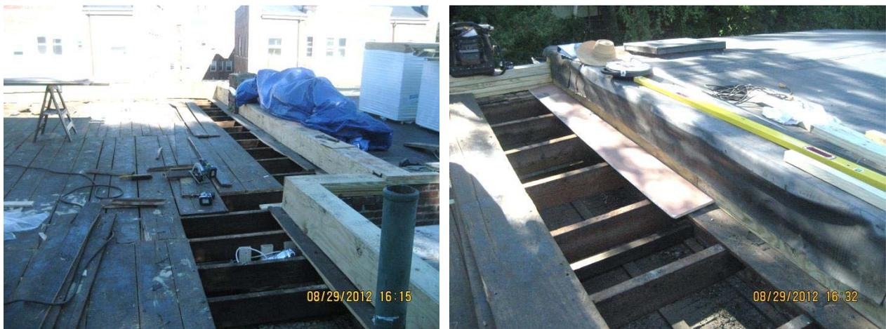
**Figure 14: Existing boards removed near roof perimeter with P.T. plywood installed at parapet (left); strip of OSB sheathing with integrated water resistive barrier at parapet (right)**
