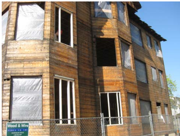
Figure 13: Windows and doors are removed
