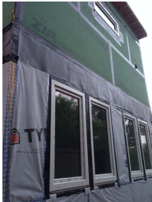
Figure 15: Re-install existing windows or install new units
