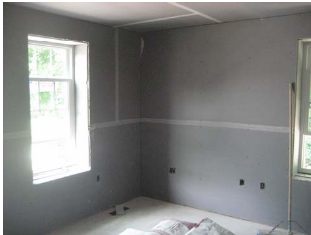
Figure 19: New gypsum board installed
