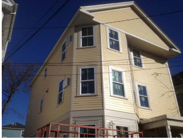
Figure 16: Completed cladding and trim
