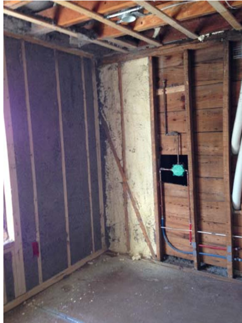
Figure 18: ccSPF and cellulose insulation
