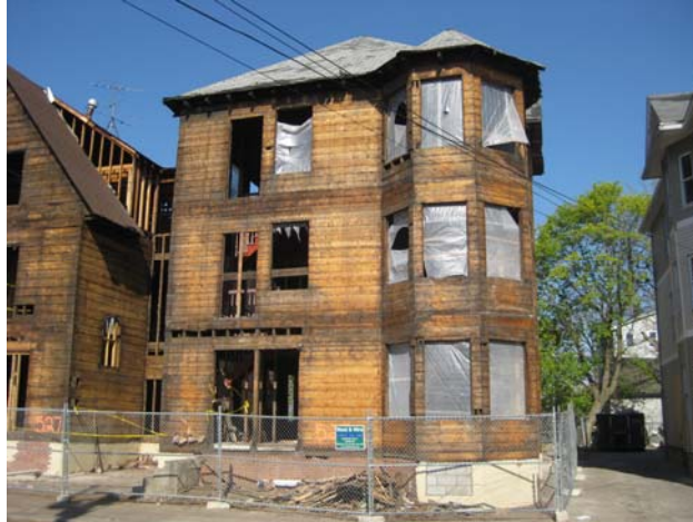
Figure 12: Exterior finishes removed and existing wall sheathing is exposed
