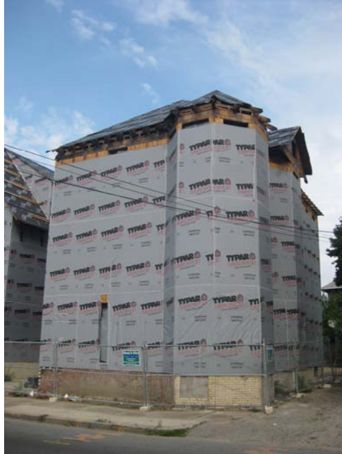
Figure 14: Water and air control membrane is in place
