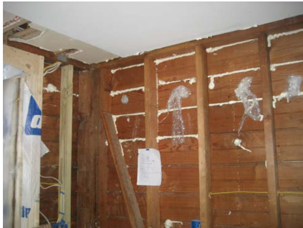
Figure 17: Interior finishes removed
