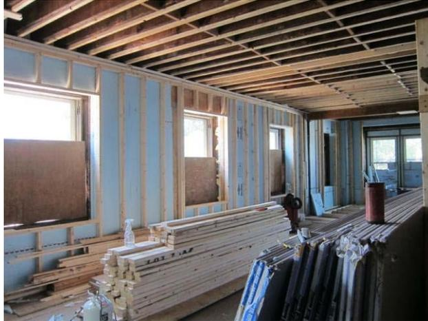
**Figure 24: Framing installed inboard of insulation**
