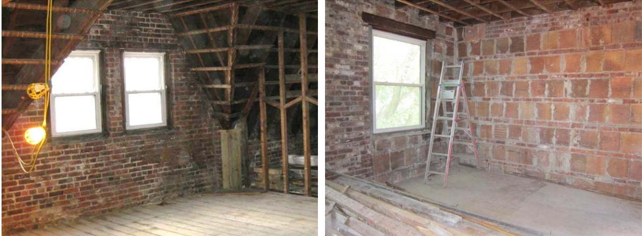
**Figure 5: Exterior wall conditions at solid brick (left) and hollow clay block infill (right) conditions**
