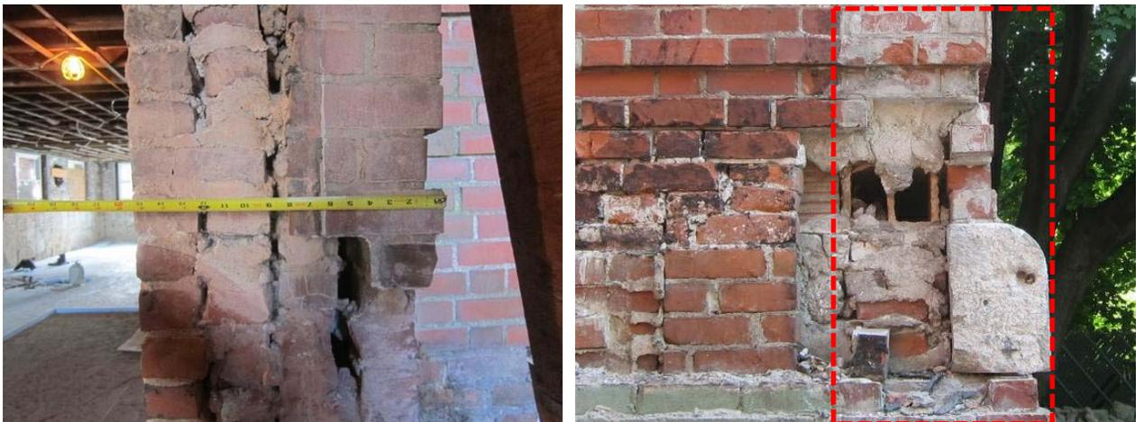
**Figure 6: Wall section at solid brick (left) and at hollow clay block infill (right) conditions**
