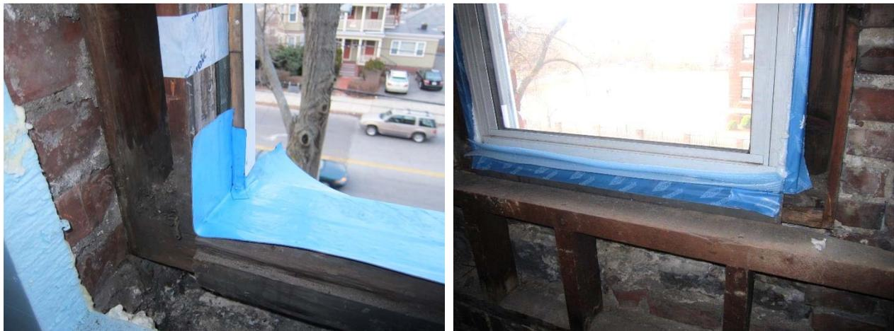
Figure 19: Openings properly flashed (left); Window re-installed (right)
