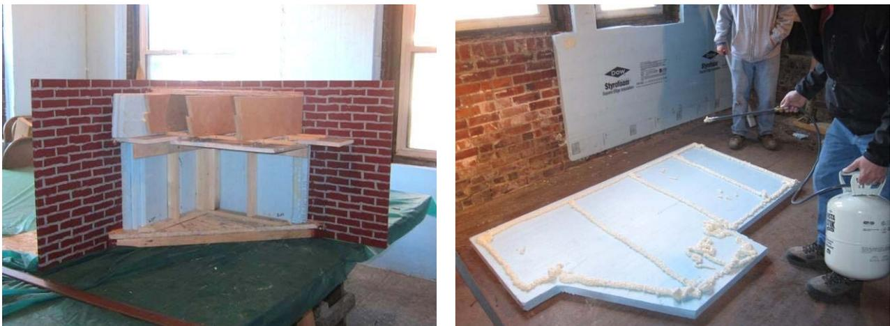
**Figure 17: Mockup (left); Use of polyurethane adhesive (right)**
