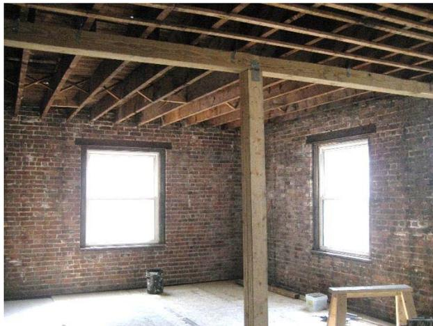
**Figure 15: Interior furring, lath and plaster removed**
