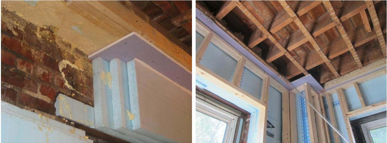
**Figure 20: Floor/ceiling fire separation gypsum board (left); Conditions after interior framing (right)**
