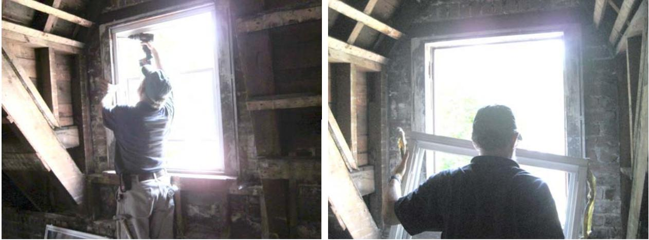
**Figure 16: Removal of existing window (left) and window removed (right)**
