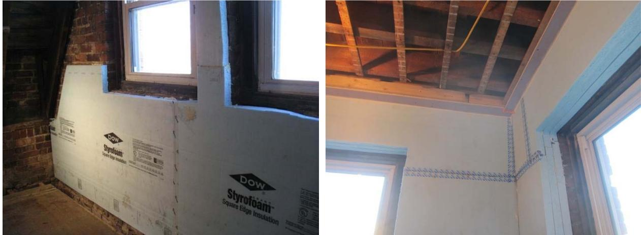
Figure 18: Installation of foam on masonry (left); Multiple layers of insulation (right)
