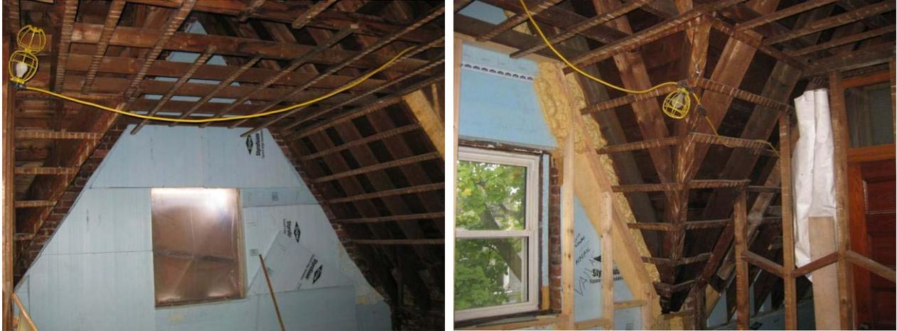
**Figure 22: Rigid wall insulation left clear of roof (left) and infill with spray foam (right)**
