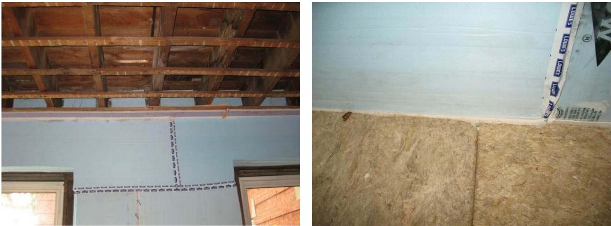
**Figure 23: Rim joist foam blocks (left); air seal between rigid foam and floor (right)**
