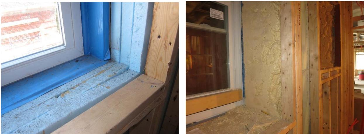
**Figure 21: Rigid wall insulation around window (left) and infill with spray foam (right)**
