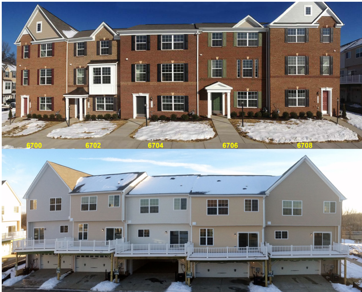
Figure 1. Villages at Pepper Mill Building 13 (5 units), front and rear elevations
