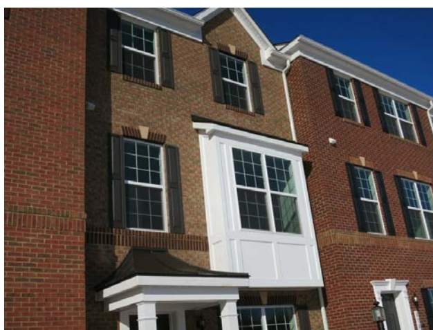
Figure 30. Front bump out bay detail at unit 6702
