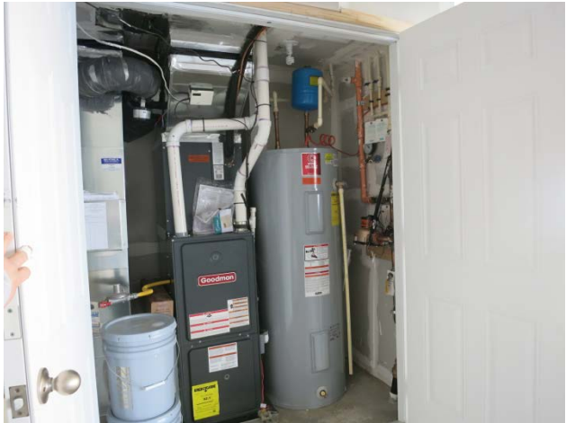
Figure 71. Furnace and water heater at mechanical room (Unit 6700); supply register
