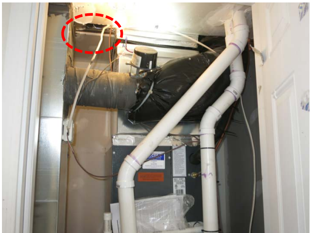
Figure 73. Ceiling penetrations at mechanical room (Unit 6702)
