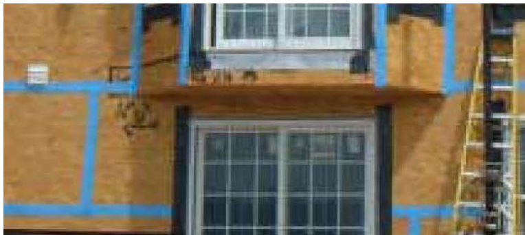
Figure 27. Overhang detail at taped sheathing condition
