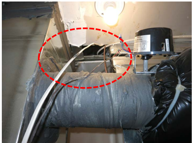
Figure 73. Ceiling penetrations at mechanical room (Unit 6702)
