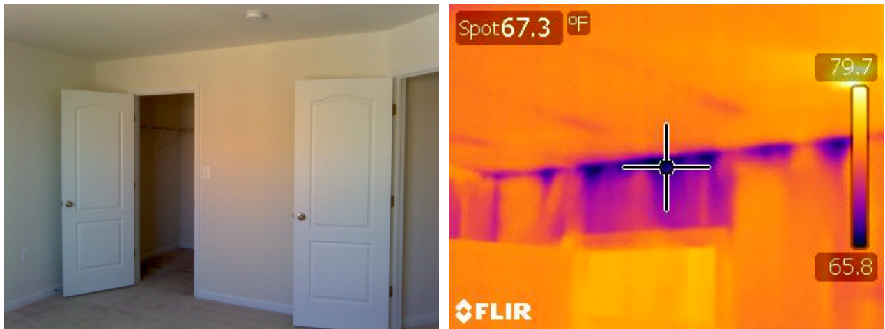
Figure 34. Interior wall under attic (third floor), Unit 6702
