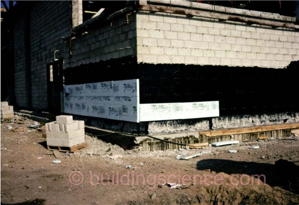
Photograph 5: "Trowel-on" drainage plane
