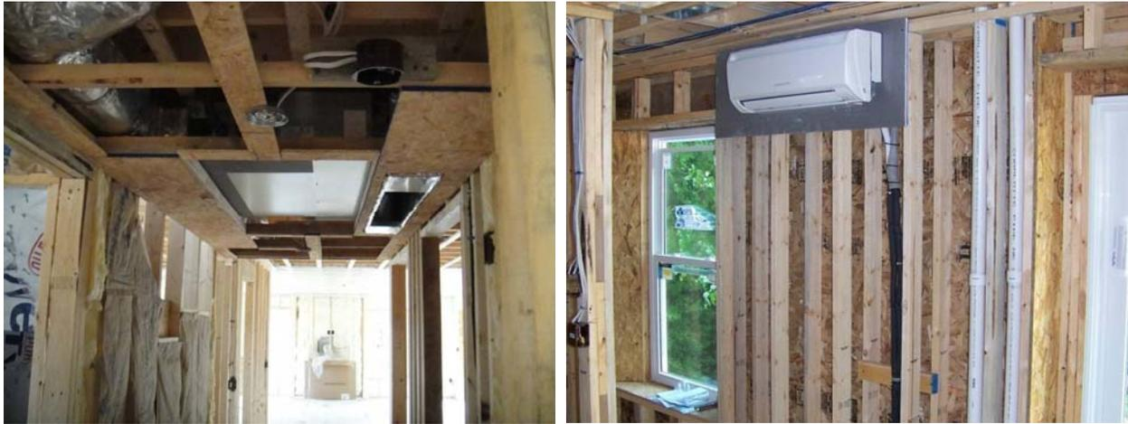
**Figure 2** *Minimally-ducted mini split mounted in dropped ceiling space (left) and single-point wall-mounted ductless split indoor unit (right)*
