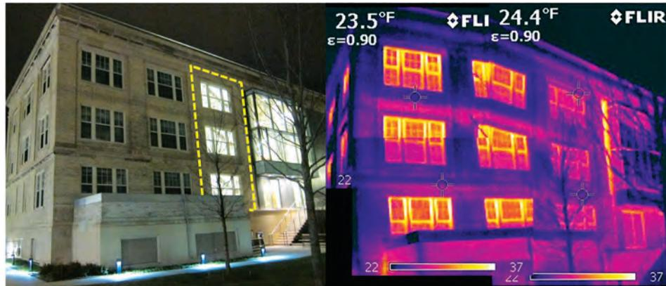
**Figure 19** Rear (north) elevation visual and infrared images (composite infrared image) with uninsulated stairwell wall highlighted.
