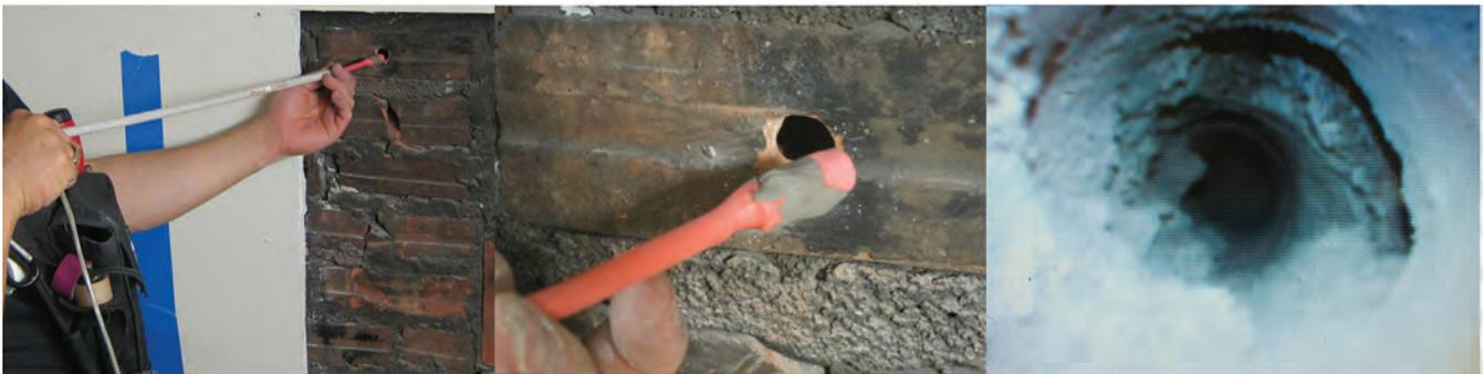
**Figure 4** (Left) Installation of combined temperature and “plug” (wood cylinder) sensor; (middle) sensor encapsulated in clay for capillary contact; (right) boroscope image of installation hole.
