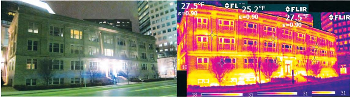
**Figure 18** Front (south) elevation visual and infrared images (composite infrared image). There is a significant thermal anomaly (indicating heat loss) at the entryway; this is consistent with the heated but uninsulated (due to historic finishes) entryway, and possibly air leakage around the entry doors.
