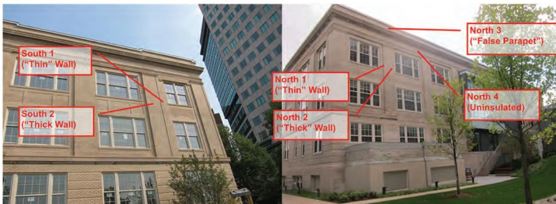
**Figure 2** South (front) and north (rear) monitoring locations and wall type nomenclature.
