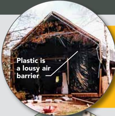
Peel-and-stick membrane was available when the author completed this retrofit, but it seemed like an excessive step when the air-control layer would be covered with foam anyway. Turns out that plastic, with its many holes, and a single layer of foam (that shrunk) didn't work so well at controlling air movement.
