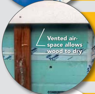
A common criticism of the author's wall assembly was that the furring strips needed to be pressure-treated or they would rot. Because the whole point of a vented airspace behind siding is to allow the siding to dry, the author reasoned that the furring strips ought to dry quickly, too. He was right. Not only did the paint job last 16 years, but the furring strips were in pristine condition as well.
