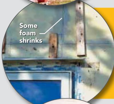
The biggest surprise was not that heat escaped between the joints of a single layer of foam, but that the gaps got bigger. Gaps are clearly visible above this window where the EPS foam panels shrunk, opening cracks in the mastic. On the house, where the author used XPS (drawing right), the panels stayed put, and the tape stuck tight.
