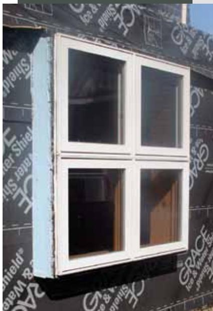
When thickening walls by 8 in., one of the difficult design details is how to install and trim windows. The author chose to cantilever plywood boxes past the frame and to install the windows with masonry straps. Naysayers cautioned that the boxes would sag under the weight of the windows, but time told a different story.
