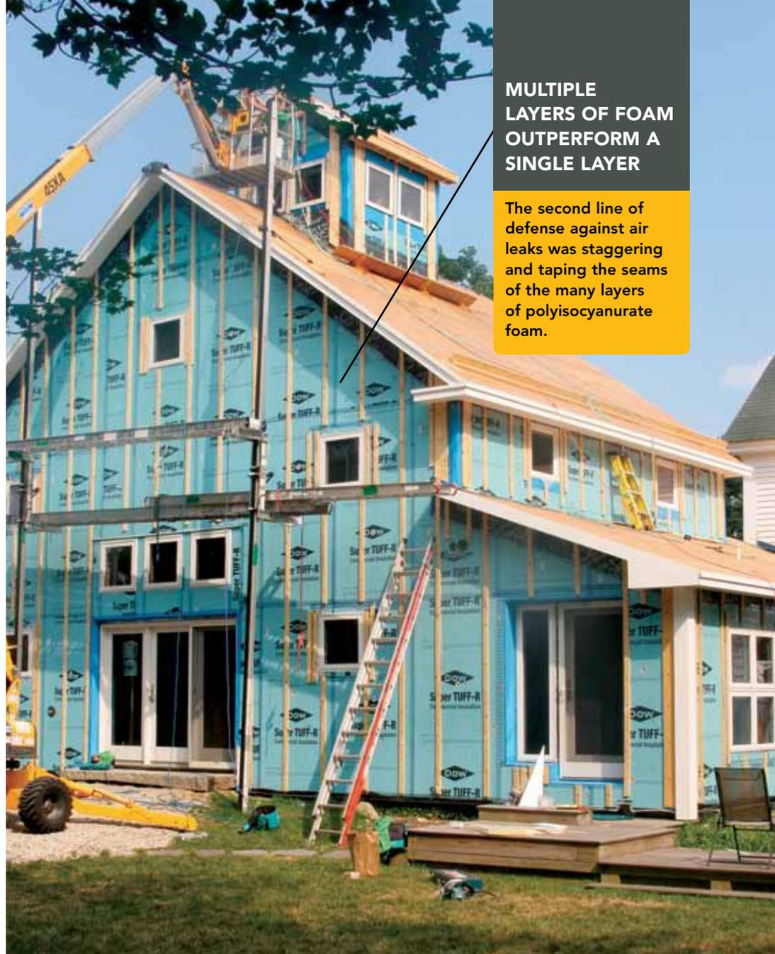
**MULTIPLE LAYERS OF FOAM OUTPERFORM A SINGLE LAYER**
