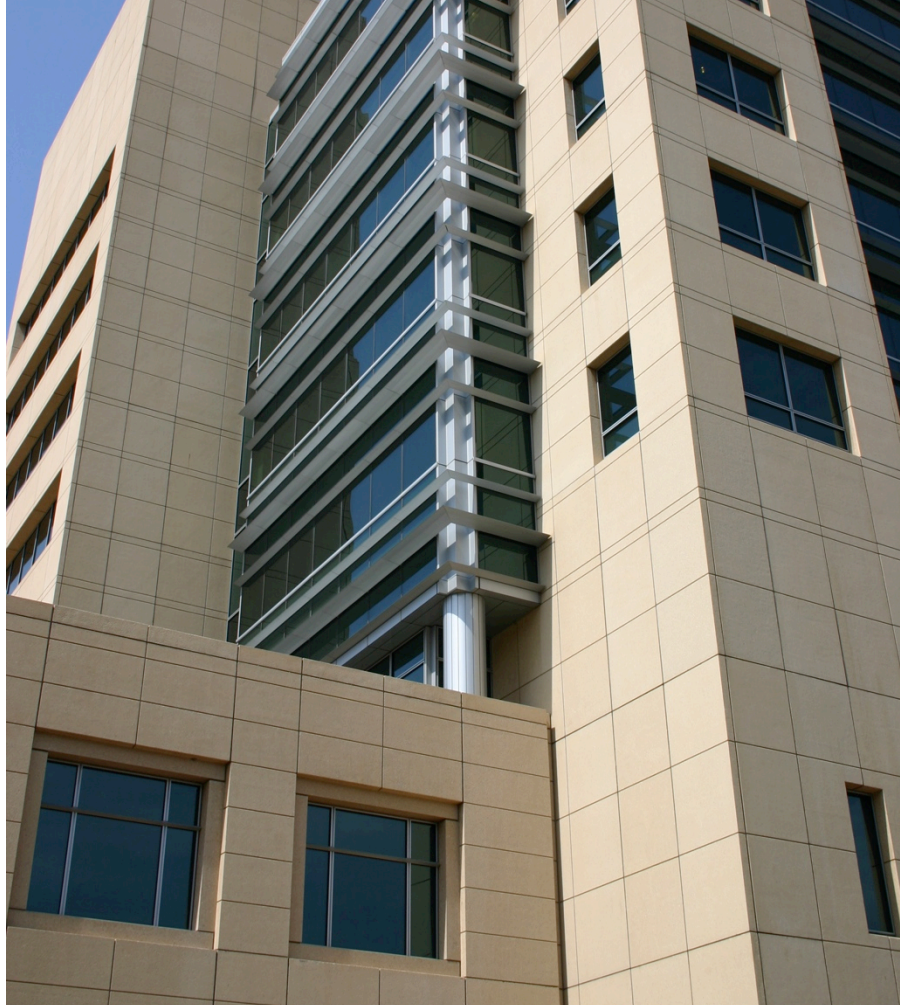
Figure 1: Attention to detail will ensure precast concrete wall panels provide high-performance enclosures.
