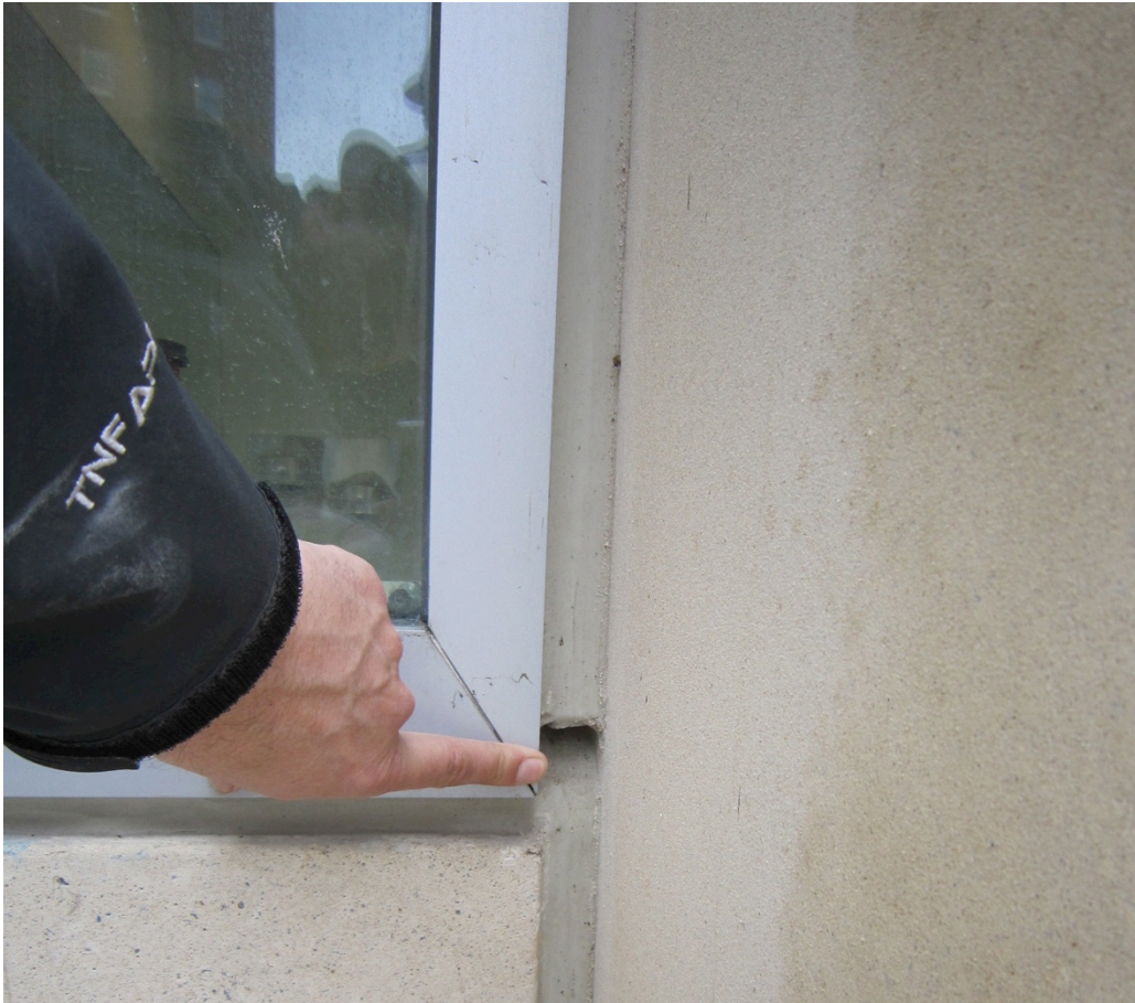
Figure 18: Weephole in a drained two-stage joint
