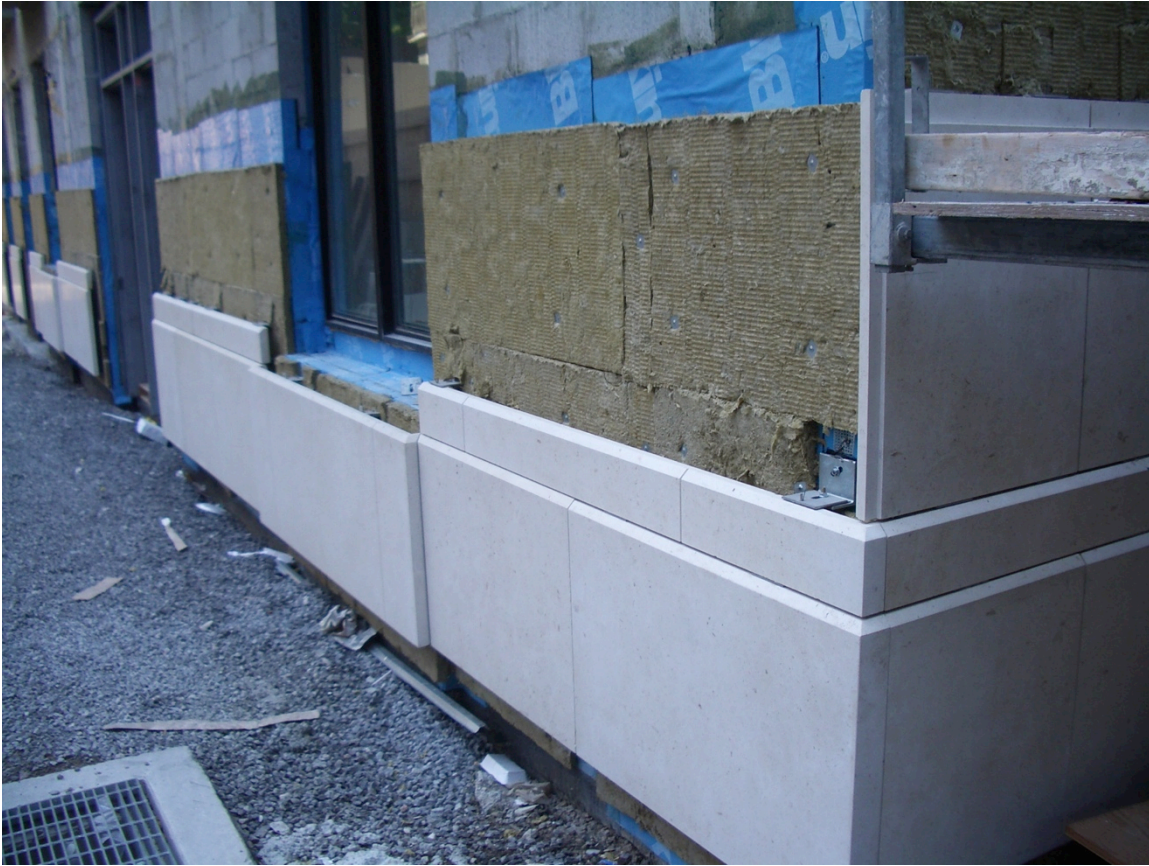
Figure 4: Small-format, handset precast installed as drained system
