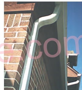
Gutters and downspouts
