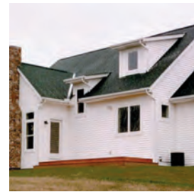
Proper grading around house
