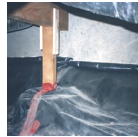
Polyethylene ground cover in crawlspace
