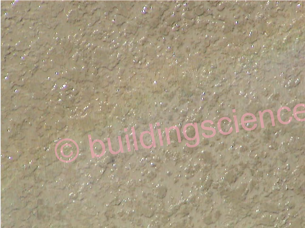
Photograph 70: Fiber Reinforced Stucco Rendering to Control Cracking
