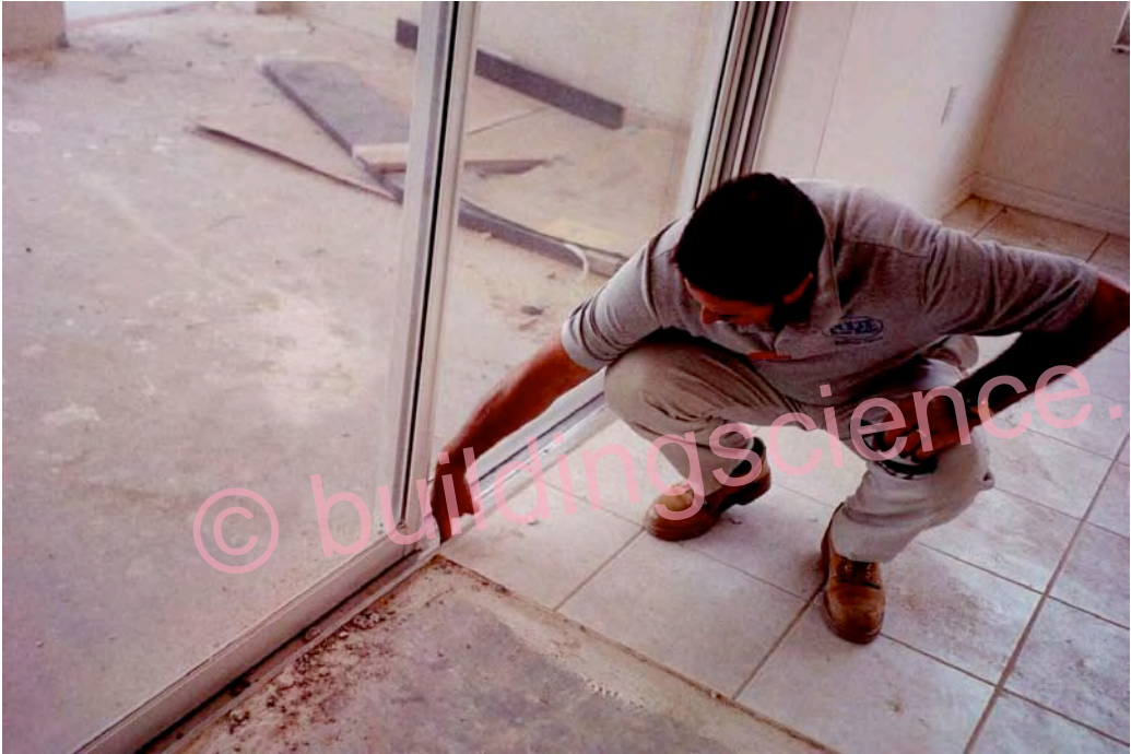
Photograph 30: Sliding Door Unit In Seat in Slab Directing Door Leakage Outward
