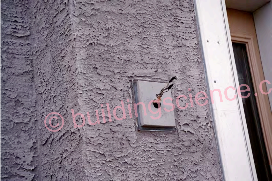
Photograph 36: Flashed Electrical Box
