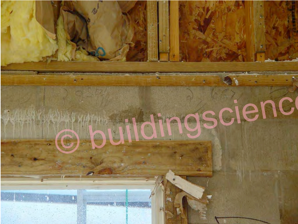
Photograph 17: Water Entry Between Floors
