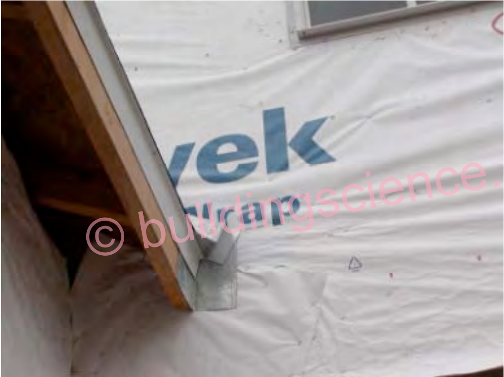
Photograph 38: Recommended KickOut Flashing Detail
