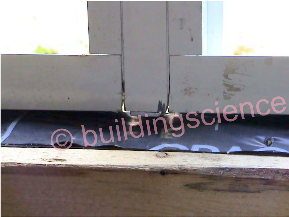
Photograph 26: Mulled Window Unit Leakage Paths
