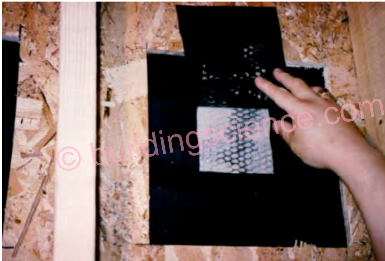
Photograph 10: Asphalt Saturated Felt As Bond Break Over Building Paper
