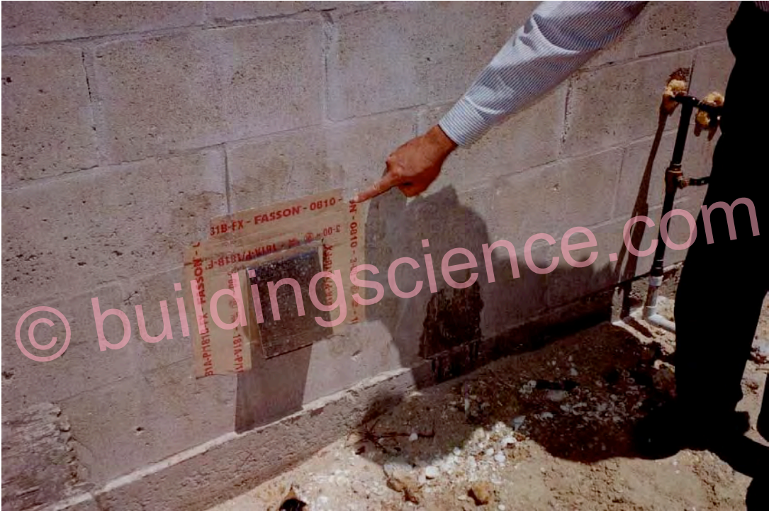
Photograph 36: Flashed Electrical Box
