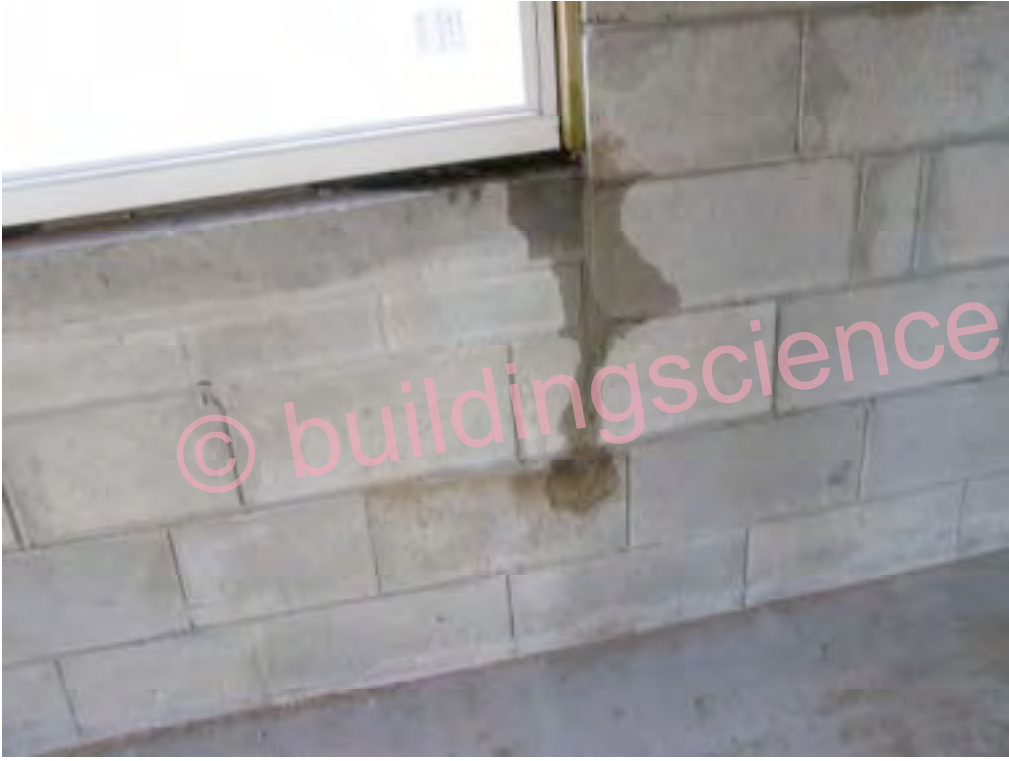
Photograph 24: Window Corner Leakage
