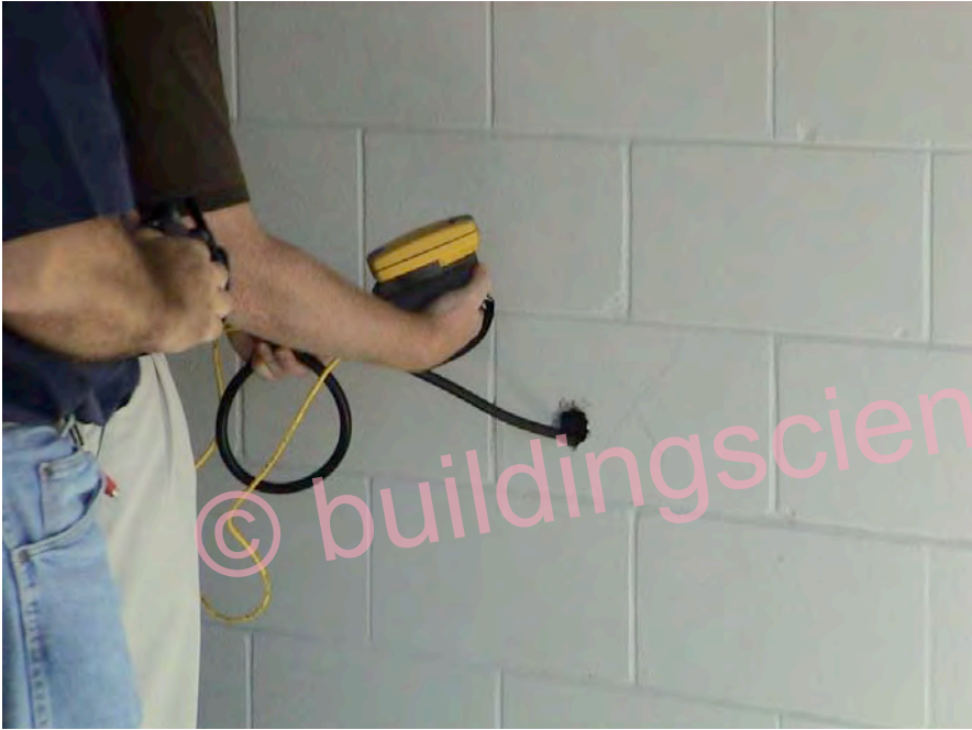
Photograph 45: Camera Probe Leak Detection
