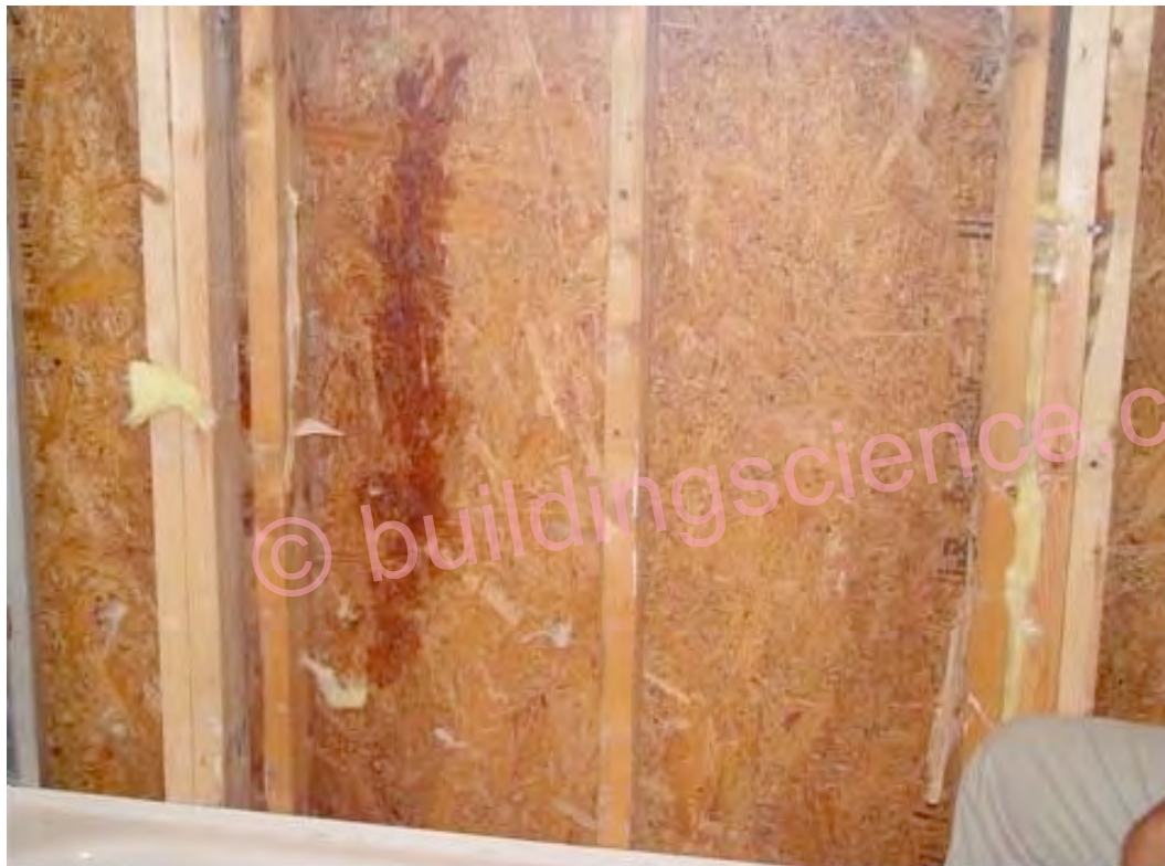
Photograph 2: Rainwater Entry into Second Floor Frame Assembly
