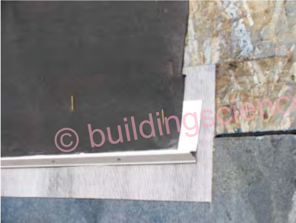
Photograph 20: Primary Drainage Plane Lapped Over Control Joint Flashing
