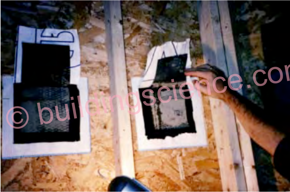
Photograph 12: Paper Backed Lath As A Bond Break
