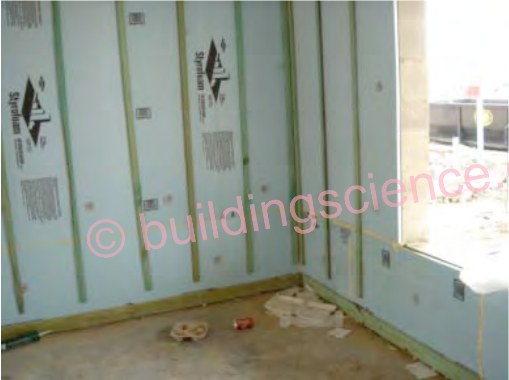
Photograph 64: Rigid Foam Interior Lining Protecting Interior Surfaces
