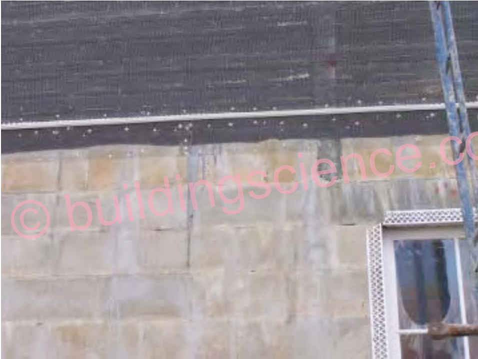
Photograph 17: Water Entry Between Floors
