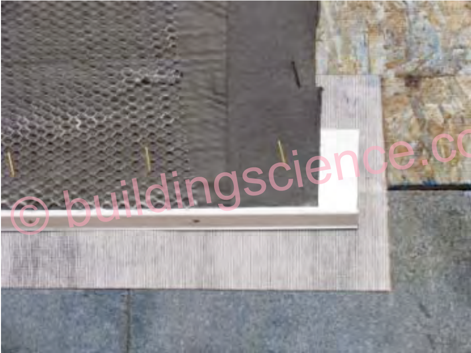
Photograph 22: Stucco Rendering Applied At Draining Control Joint
