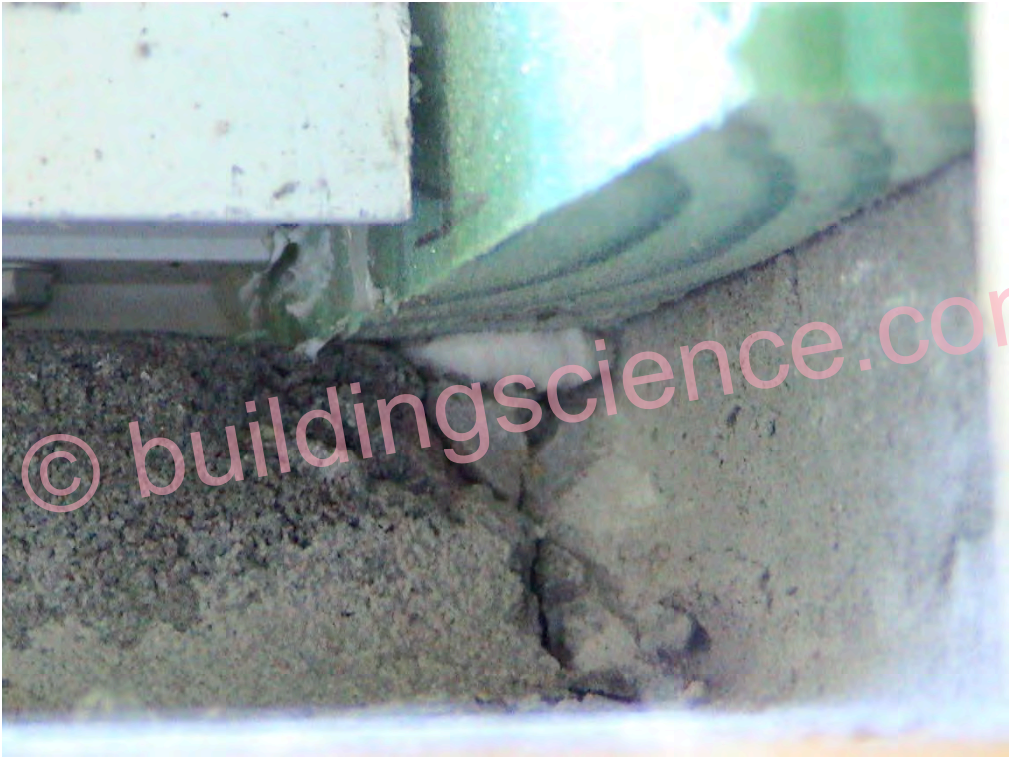
Photograph 26: Mulled Window Unit Leakage Paths
