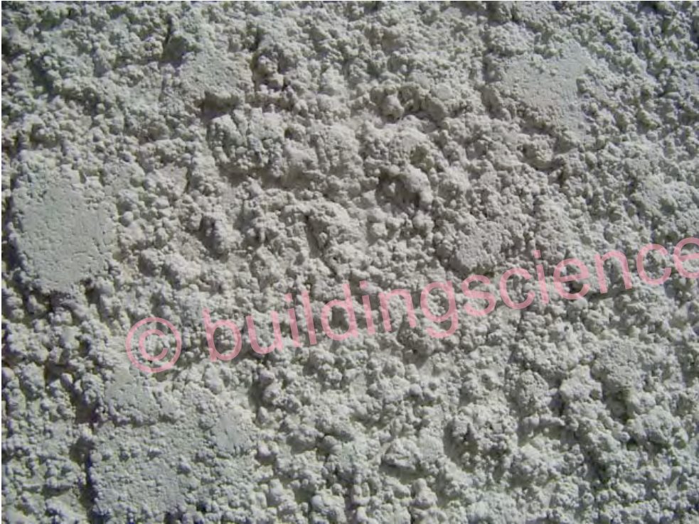
Photograph 66: Paint Coating Over Rough Surface
