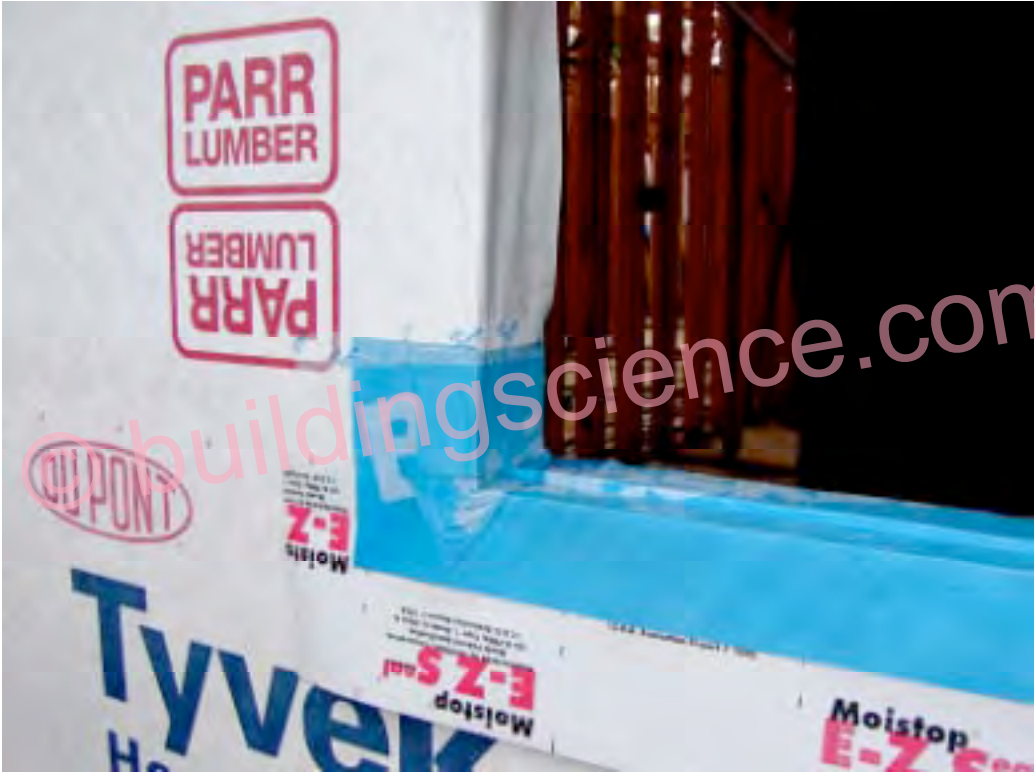
Photograph 30: Sliding Door Unit In Seat in Slab Directing Door Leakage Outward
