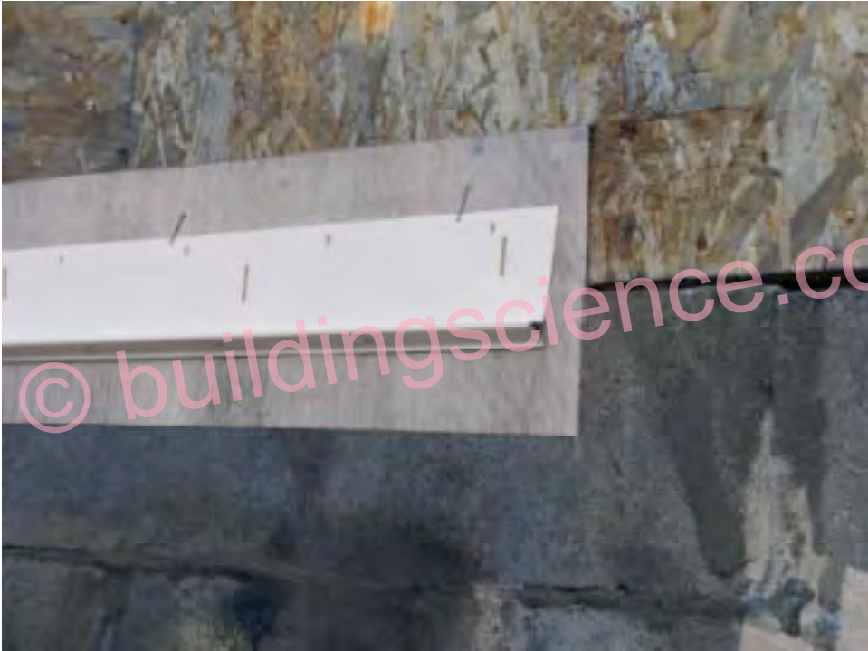
Photograph 20: Primary Drainage Plane Lapped Over Control Joint Flashing
