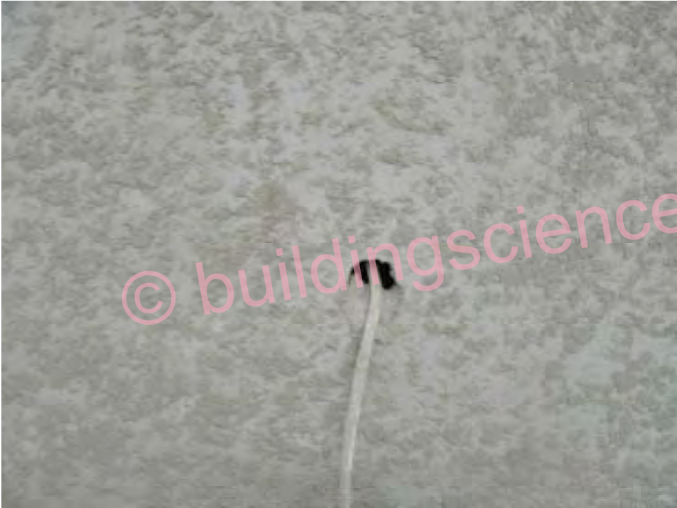
Photograph 32: Typical Maintenance Intensive Service Opening
