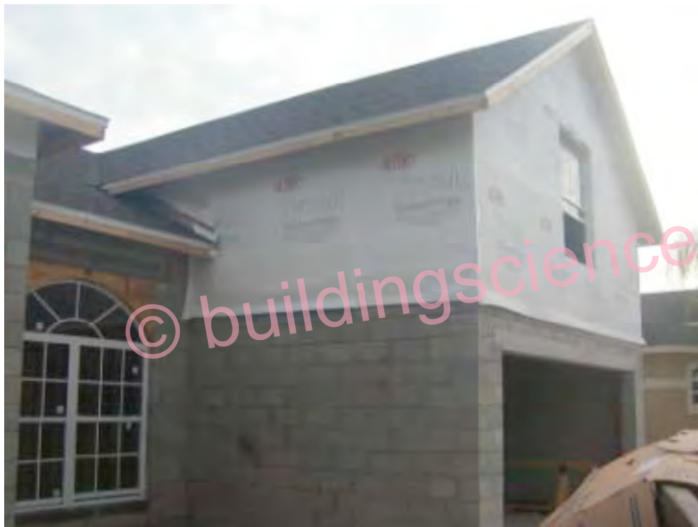
Photograph 13: Enhanced Drainage With A Profiled Plastic Housewrap
