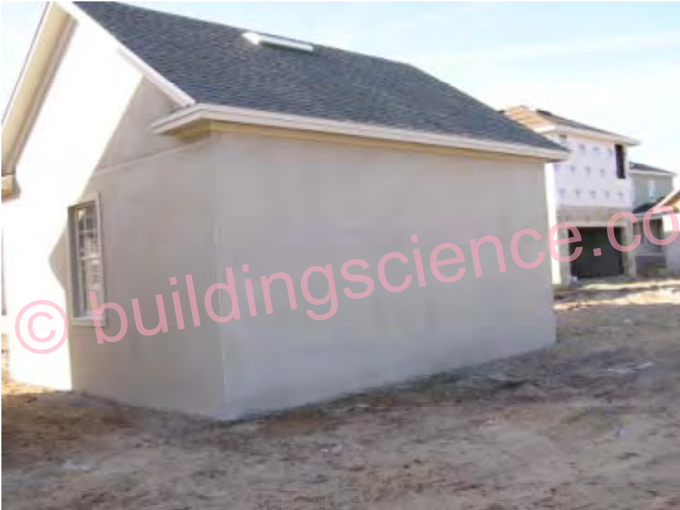
Photograph 53: Painted Stucco Rendering Test Wall
