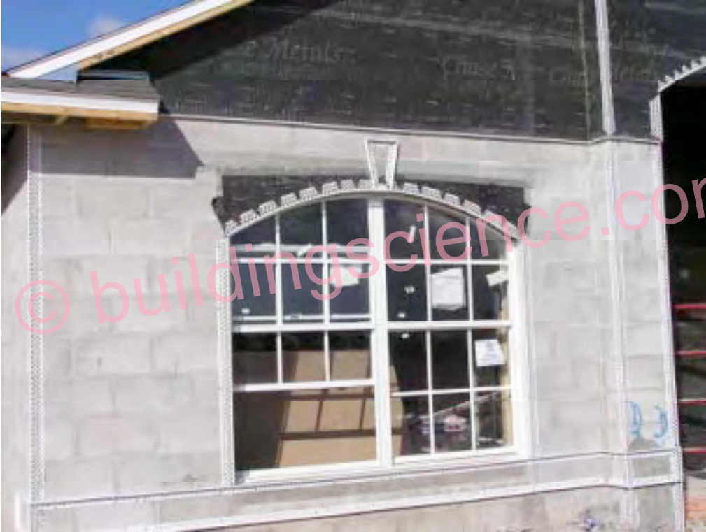
Photograph 24: Window Corner Leakage
