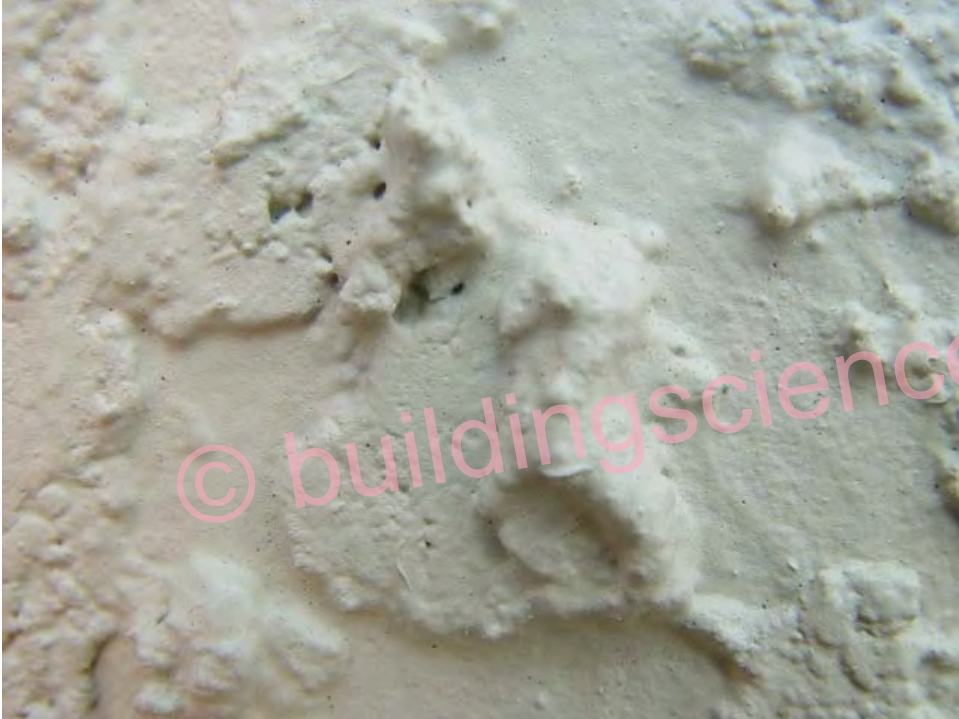
Photograph 68: Paint Coating – 10 Mil Thickness
