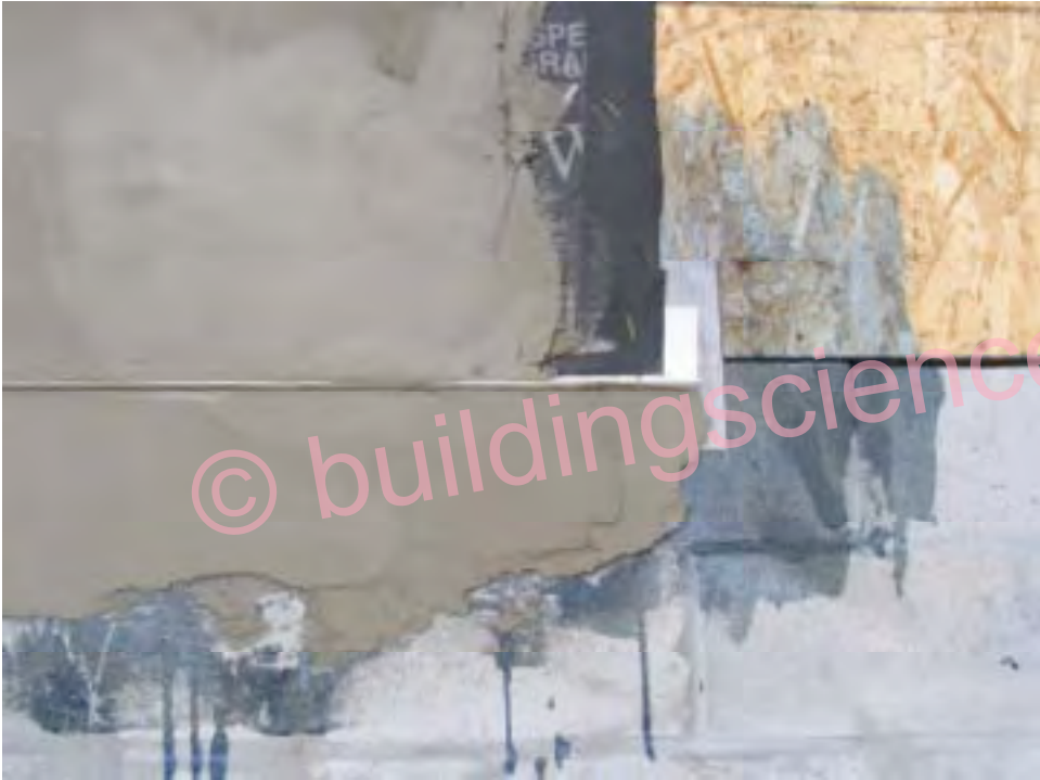
Photograph 22: Stucco Rendering Applied At Draining Control Joint
