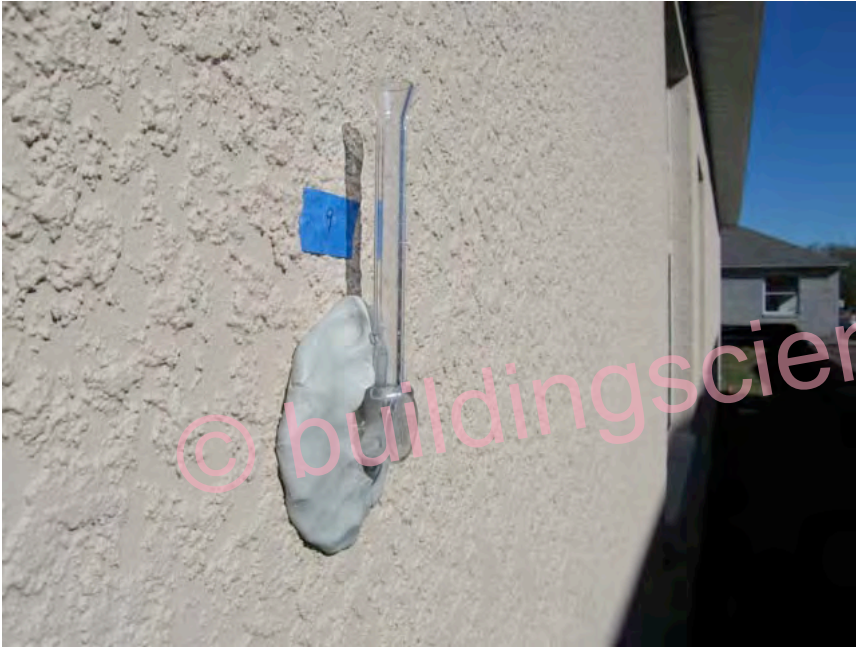
Photograph 43: Rilem Tube Hydrostatic Head Test
