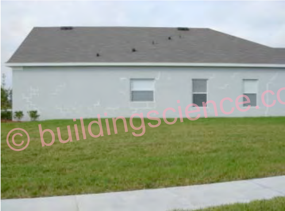
Photograph 70: Fiber Reinforced Stucco Rendering to Control Cracking
