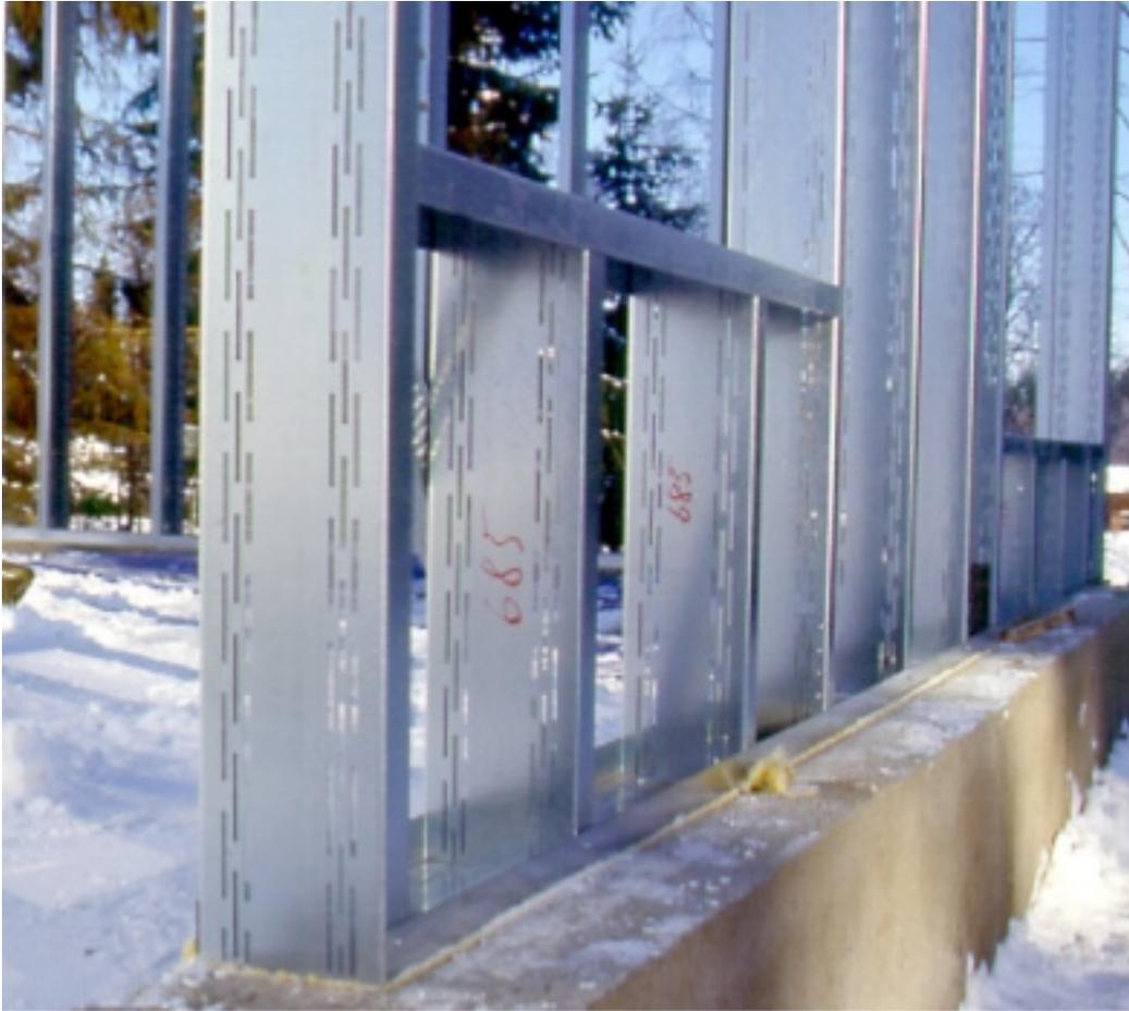
**Figure 5: Thermally Efficient Steel Framing in Finish Housing (Nieminen & Salonvaara 2000)**
