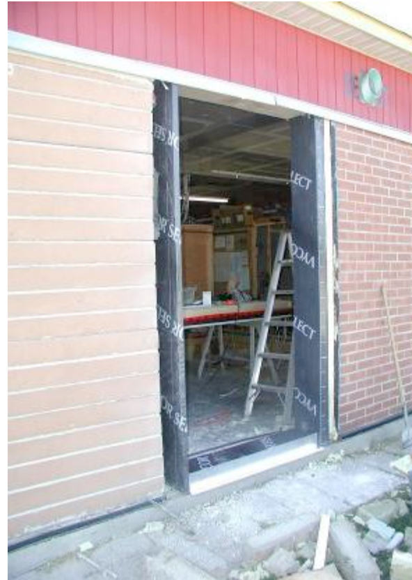
Figure 2.2: Opening perimeter details for removable test walls
