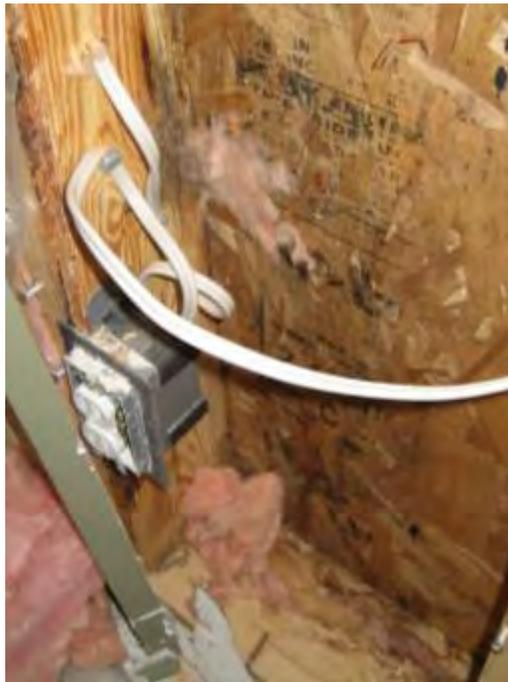
**Figure 29 : Example of air leakage condensation durability issues.**
