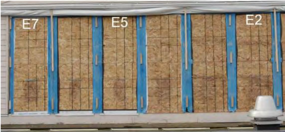
**Figure 40 : Exterior OSB sheathing on the east orientation immediately following deconstruction**
