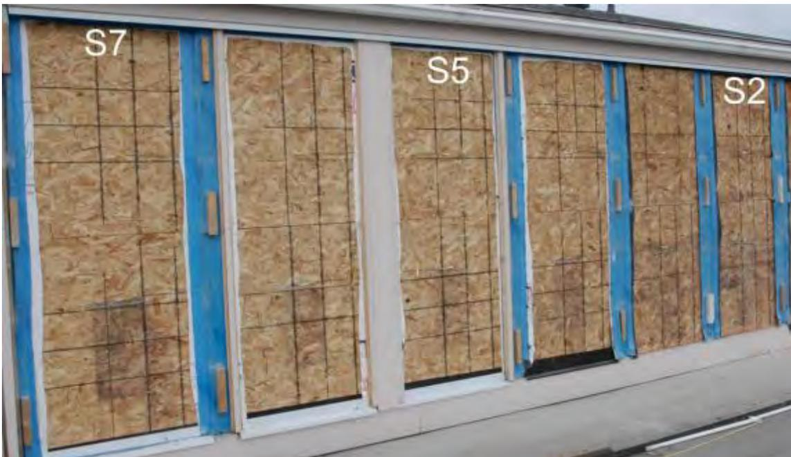
**Figure 41 : Exterior OSB sheathing on the south orientation immediately following deconstruction**
