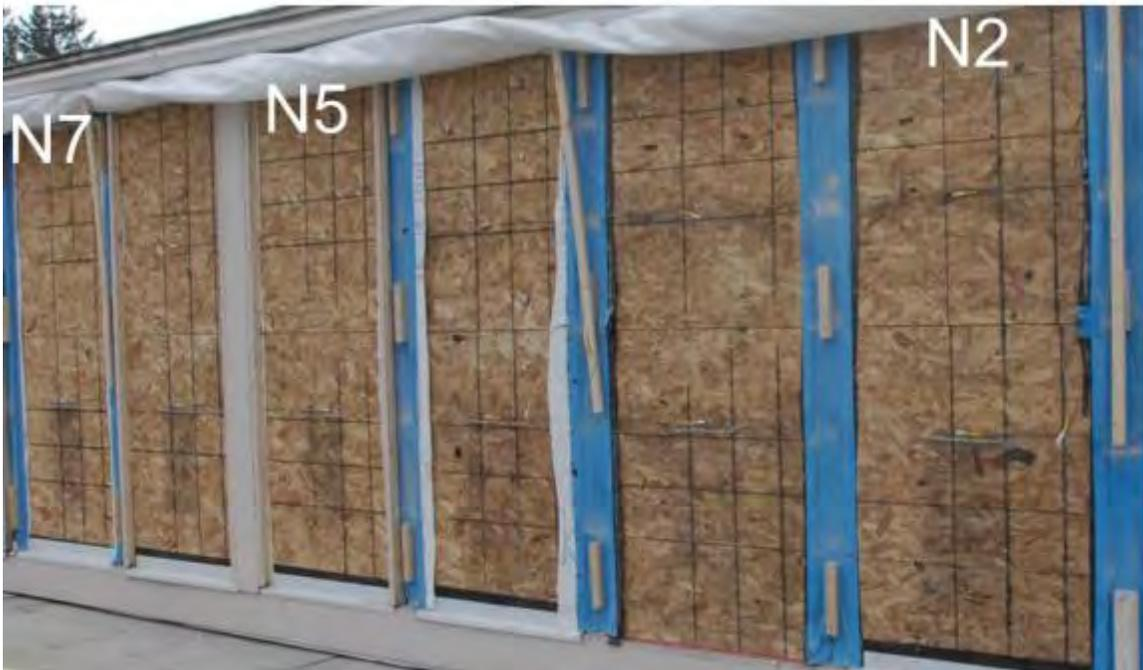
**Figure 39 : Exterior OSB sheathing on the north orientation immediately following deconstruction (photo taken from the opposite direction of Figure 38)**
