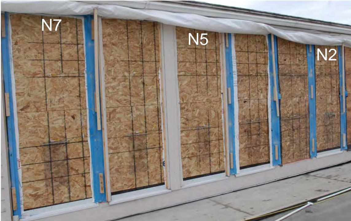
**Figure 38 : Exterior OSB sheathing on the north orientation immediately following deconstruction**
