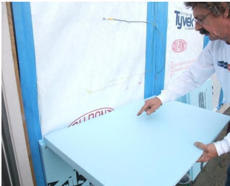
**Figure 12 - Installation of Dow XPS 1.5" Insulation**
