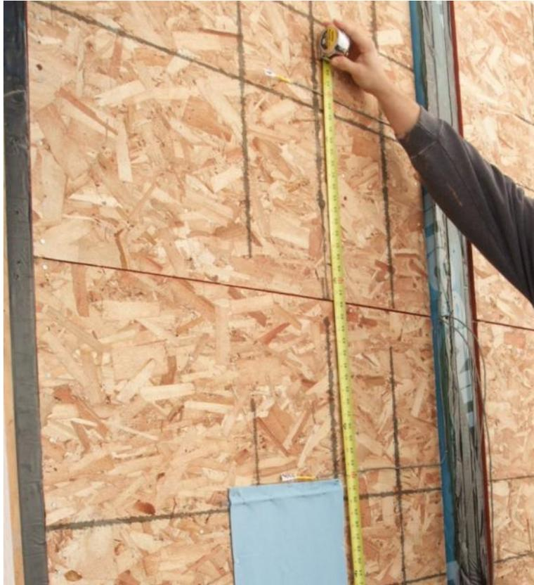
**Figure 11 - Exterior Upper and Lower T/RH Sensors**
