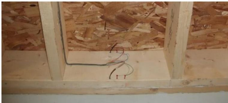
**Figure 9 - Bottom Plate MC/T Sensors**
