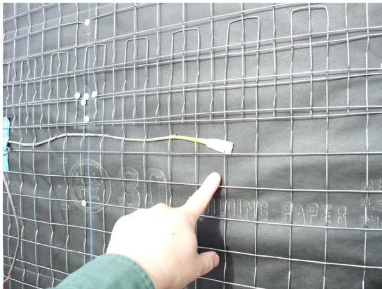
**Figure 10 - Exterior Mid-Height T/RH Sensor Outboard of Building Paper**
