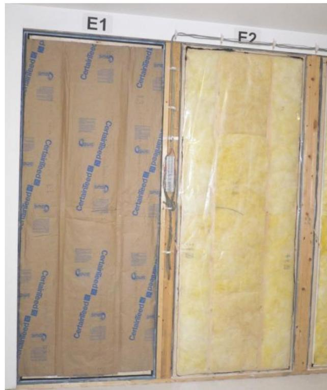
**Figure 17 - Interior Vapor Control and Stud Space Insulation**
