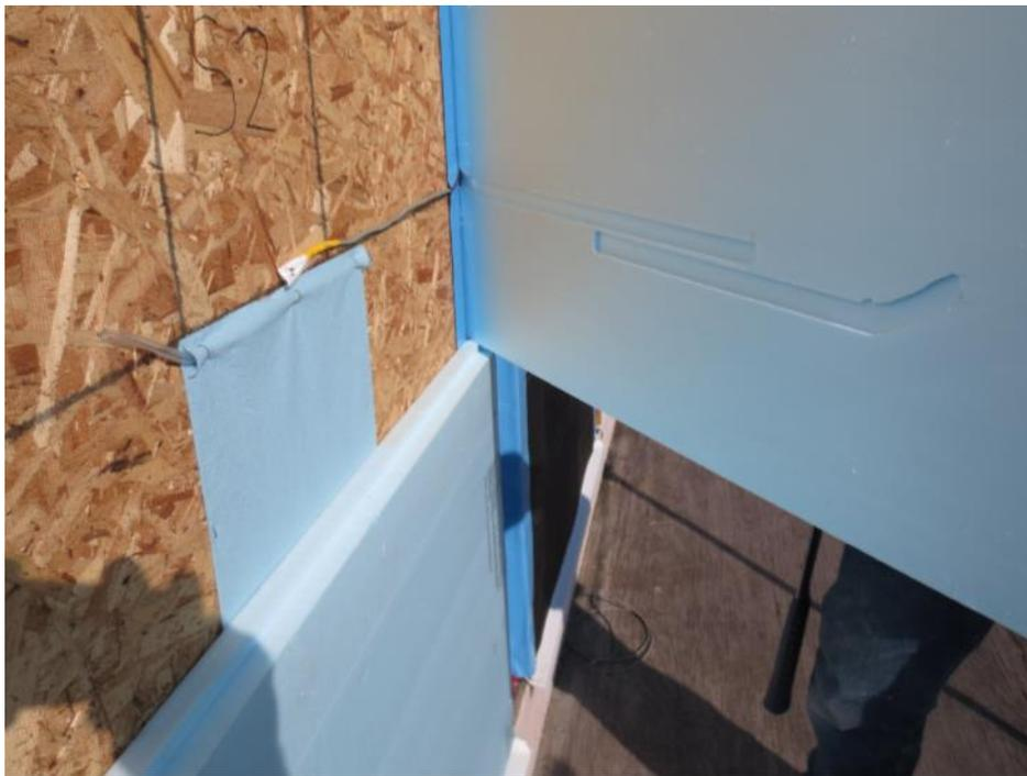
**Figure 20 – Sensor and wetting apparatus tube pockets in XPS Insulation**
