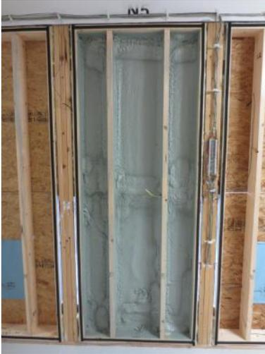
**Figure 8 : North Wall 5 with approximately 2" of closed cell 2pcf spray foam**
