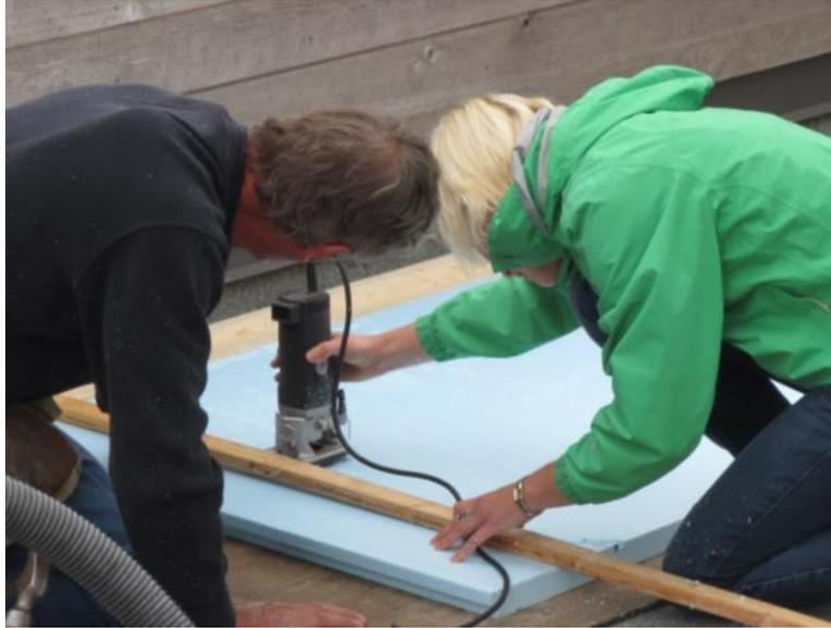
**Figure 19 – Creating small grooves on the interior surface of board foam insulation**
