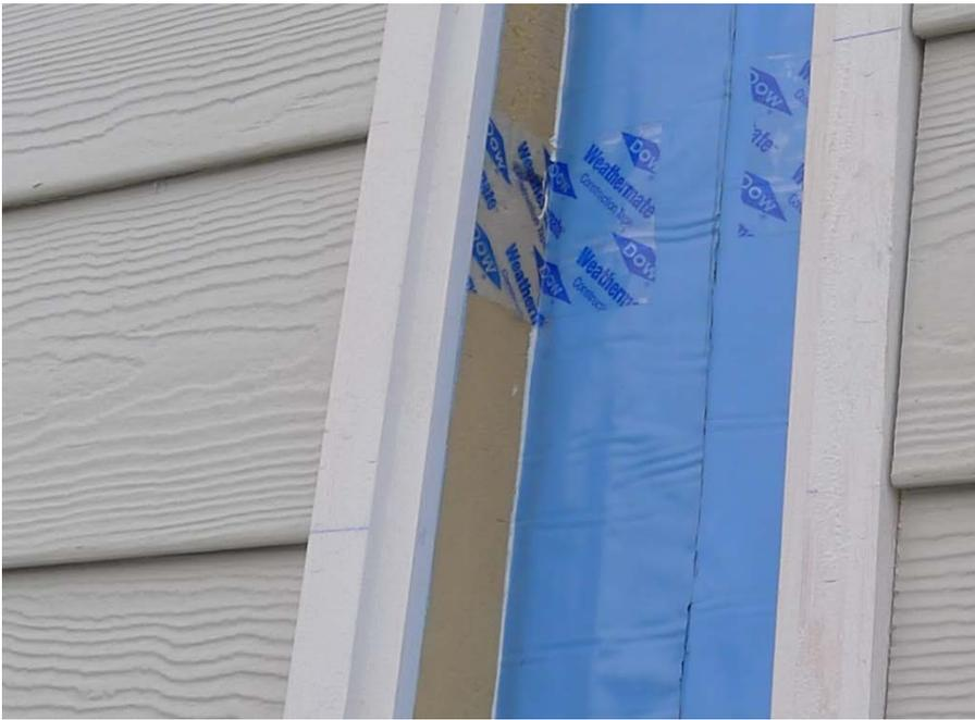
**Figure 12 : Sealant installed at the interior surface of exterior insulation**
