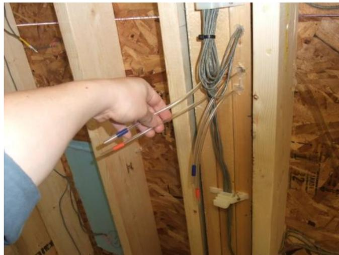
Figure 23 - Wetting Apparatus Injection Tubes
