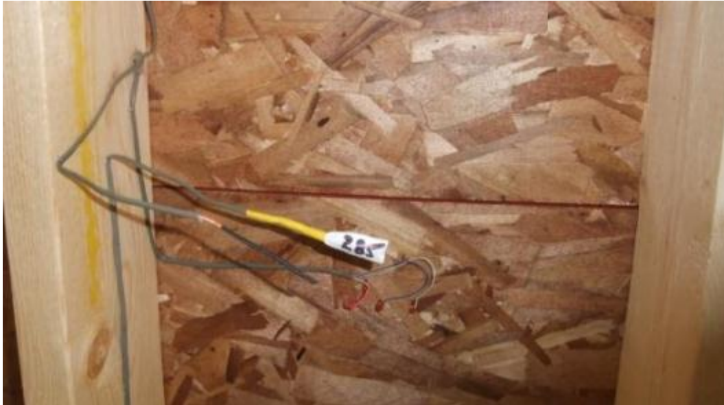
Figure 4 : Relative Humidity and temperature sensor installed in a stud bay (with moisture content pins installed below).
