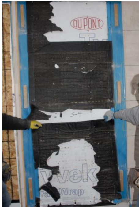
Figure 18 : Wall 4 - Deconstruction showing building paper over DrainWrap
