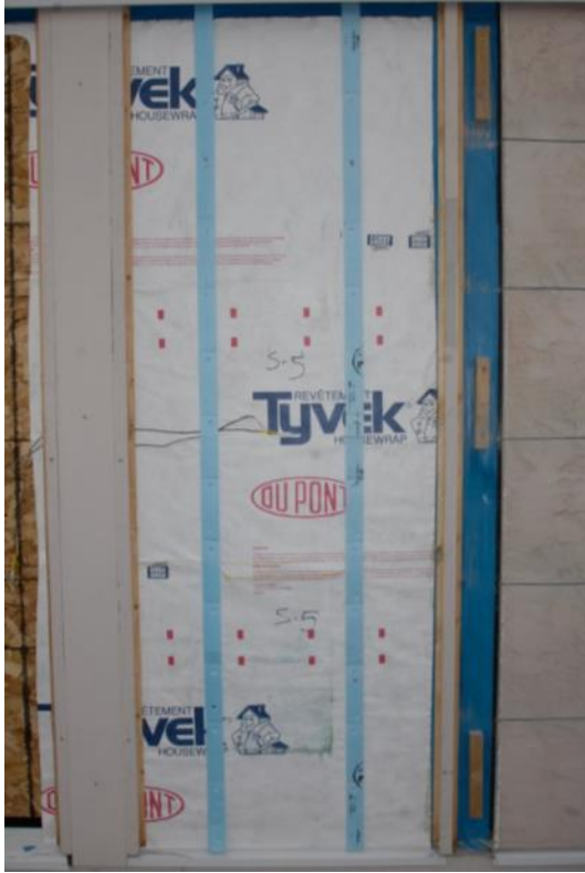
Figure 16 :3/8” XPS strips installed over sheathing membrane behind HardiePlank
