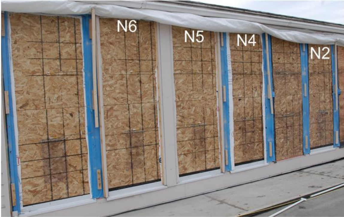
Figure 35 : Exterior OSB sheathing on the North orientation immediately following deconstruction
