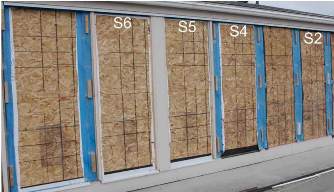
Figure 37 : Exterior OSB sheathing on the South orientation immediately following deconstruction
