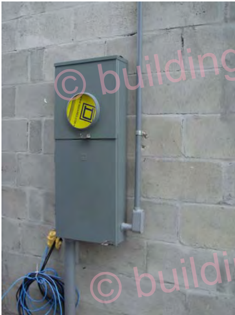
Figure 15: Panel installed before installation of the drainage plane
