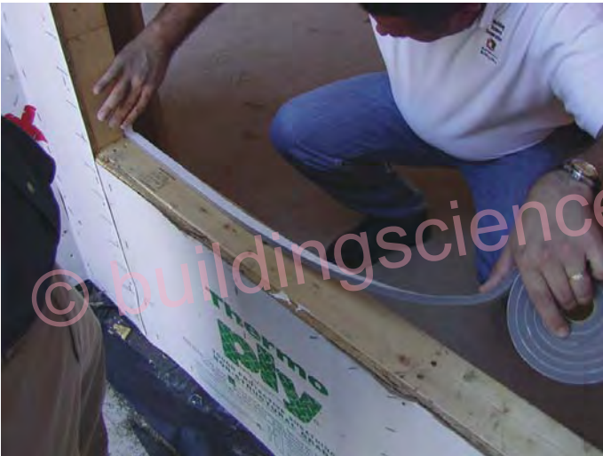
Figure 31: Weather seal gasket used as a backdam
