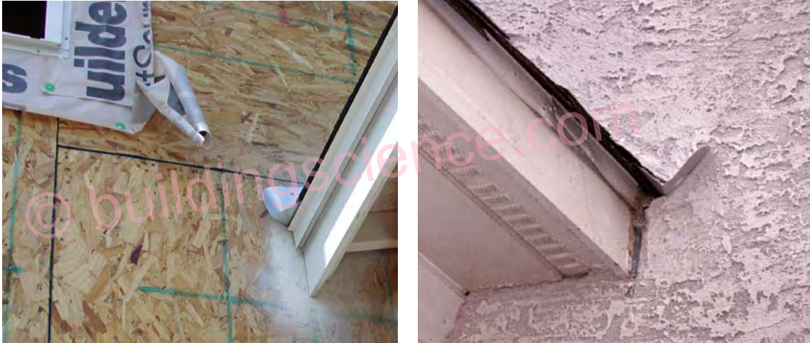
Figure 12: Kick out flashing installations
