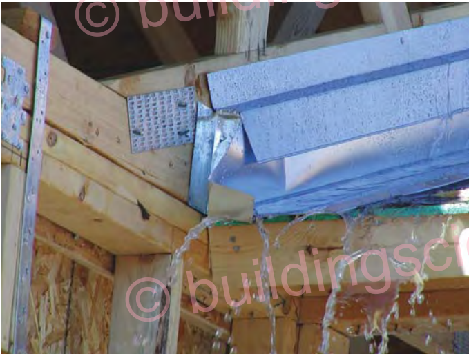
Figure 13: Poorly folded kick out flashing
