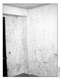
Mold growth on exterior walls was one of the most visible symptoms of moisture problems at this Cleveland Housing Authority apartment.
