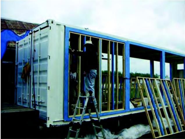
**Figure 1** Installation of specimen wall framing in container.
