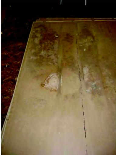
**Figure 17** *Mold on brick west wall gypsum wallboard.*
