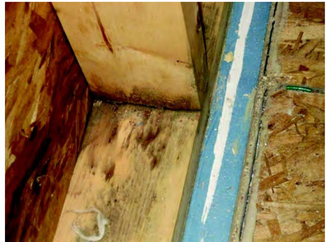
**Figure 18** *Moisture on bottom plate.*
