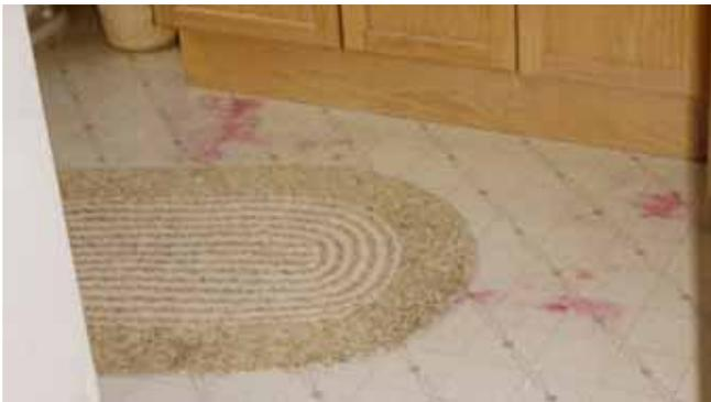
**Photograph 4: Vinyl Flooring**—Pink spots due to moisture problems arising from the impermeability of the vinyl flooring and ventilated and insulated crawlspace underneath.
