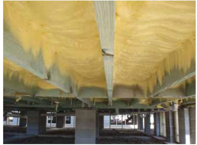
**Photograph 6: Spray Foam Between Joists**—Floor framing is not completely encased with spray foam in this application. Works only where the crawlspace is open to the outside.
