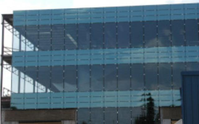
**Photo 1:** An all-glass “high-performance” thermally-broken curtainwall with low-e, argon-filled glazing units and R-12 spandrel insulation. Sleek appearance but dismal performance by any normal standard. The R-value of the combined spandrel and glazing is less than R-4, and the solar gain is high enough to require air-conditioning on cold sunny winter days.
