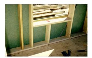
Correct window framing using Advanced Framing with single horizontal and vertical framing members
