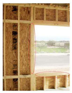
Extra framing used unnecessarily around window opening
