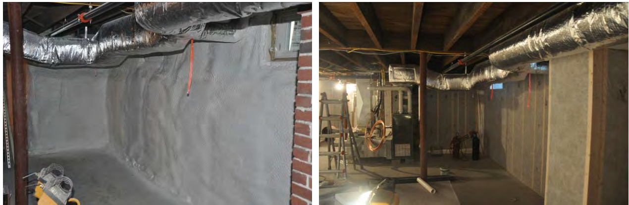
Figure 25. Basement with spray foam (L); and added cellulose in framed wall (R)
