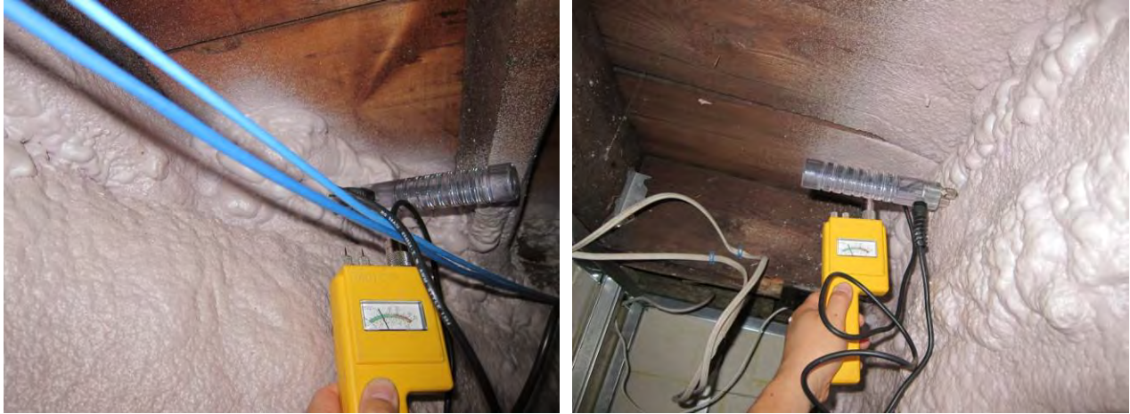
Figure 59. Sill beam moisture content measurement, Somerville Office
