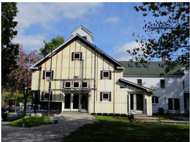
Figure 47. Westford House/Barn recladding and sill beam inspection
