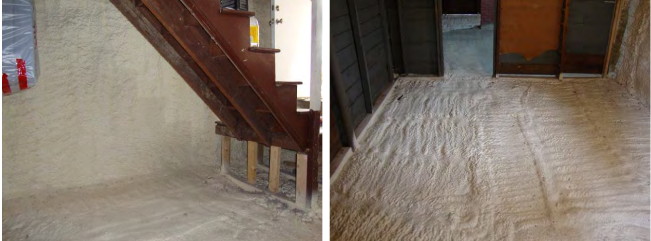
Figure 33. Spray foam applied to walls and slab (© 2011 by Byggmeister; reprinted with permission)
