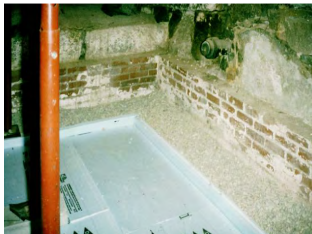
Figure 19. Sill beam lift and slab insulation and drainage (Lstiburek 2010a)
