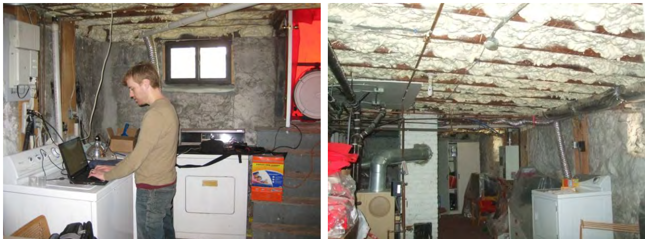
Figure 3. Arlington, MA Duplex basement ceiling spray foam, and nullified air leakage testing
