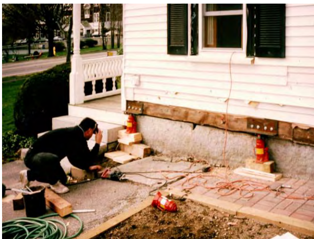
Figure 19. Sill beam lift and slab insulation and drainage (Lstiburek 2010a)
