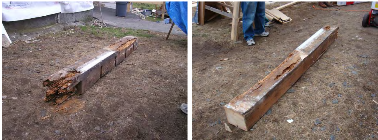
Figure 43. Damaged sill beams from Bedford Farmhouse
