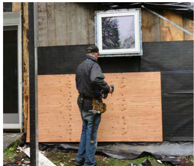
Figure 47. Westford House/Barn recladding and sill beam inspection
