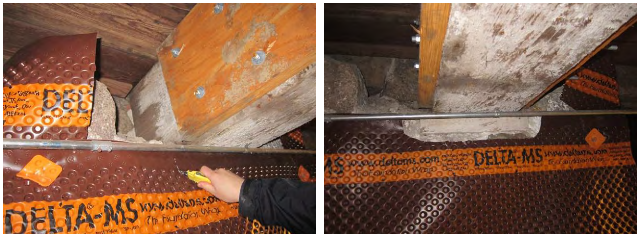
Figure 23. Air gap membrane venting to underside of beam (L); retrofitted detail (R)
