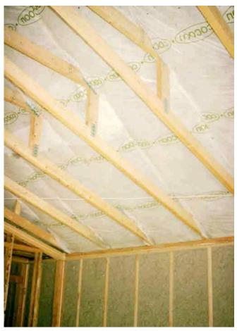
**Photograph 1: Flow-Through Assembly**—The most common insulation is netted cellulose although spray applied fiberglass, netted fiberglass and fiberglass batts are options.
