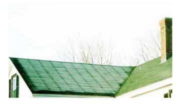
**Photograph 4. Thermal Bridging**—Guess whose house that was? Yup. It was mine. I am not as smart as I think I am most of the time. At the time this photograph was taken the underside of the roof was insulated with closed-cell spray polyurethane foam (SPF).
