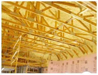
Photograph 2: Open-cell Spray Polyurethane Foam (SPF)—You cannot use open-cell in IECC climate zones 5 or higher unless the foam is used with a Class II (or Class I) vapor retarder. With open-cell foam a significant amount of moisture via vapor diffusion will pass upwards through it during cool periods and during the winter in cold climates—too much to be driven back down during sunny weather and
