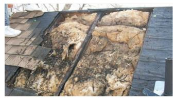
**Photograph 6: Unvented Cathedral Ceiling**—No one argues that it is a dumb idea to shove a bunch of fiberglass batts into a cathedral ceiling with no provision for ventilation air to remove some moisture. The results are often catastrophic.
