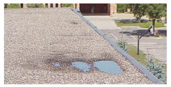
**Photograph 7: Flat Roof**—There are a gazillion of these roofs that are uninsulated and need to be addressed.
