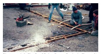
**Photograph 8: Flat Roof Being Dense Packed**—The roof is opened up and cellulose is being blown into the roof cavity dense packing it. The guy in the middle is Jim Fitzerald, the absolute best guy in the world, and he could not make it work consistently. Does that tell you something, or what?
