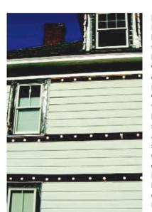
Photograph 1: **Retrofit Wall** Insulation-Note the characteristic holes through which the cellulose is injected into the wall cavities from the exterior. The holes are subsequently filled and the removed siding replaced. Quality control is often done with an infrared camera to make sure that no cavities are missed.
