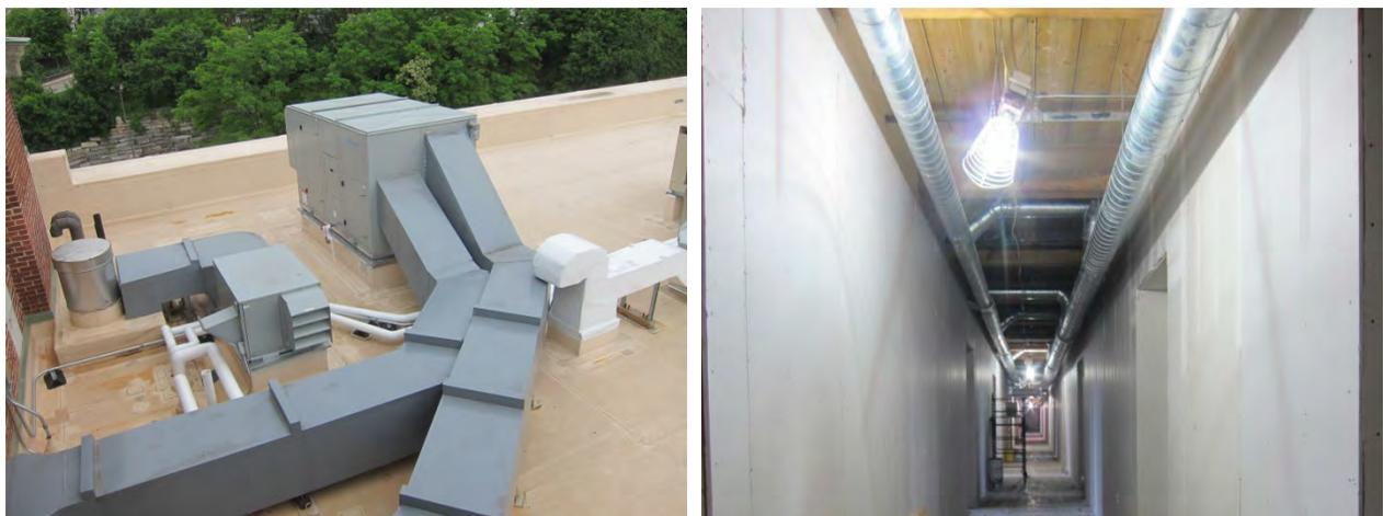
Figure 20. Rooftop HRV, with supply/exhaust ducts (L); supply and exhaust ductwork in corridor (R)
