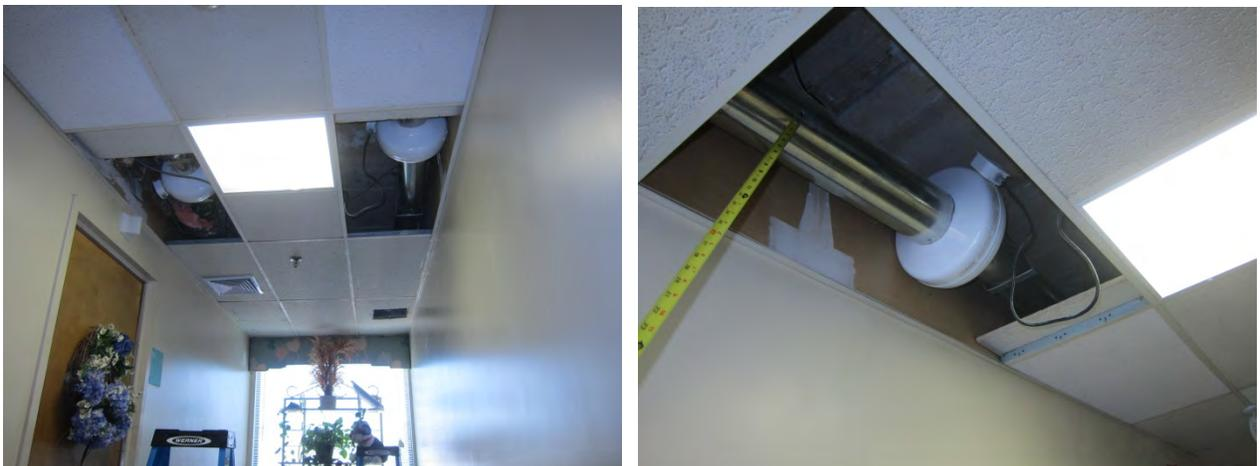
**Figure 88. Inline fans and registers in suspended ceiling**
