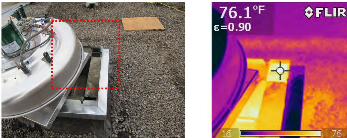
**Figure 70. Stack-driven air leakage at unsealed corners of exhaust shaft roof curb**
