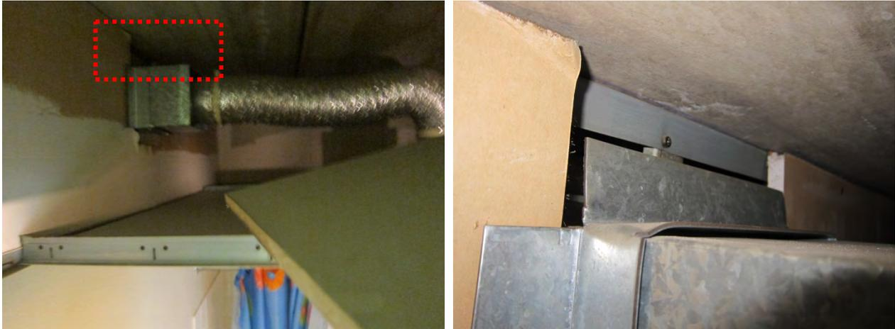
**Figure 48. Exhaust duct penetration at demising wall, showing lack of air barrier continuity**
