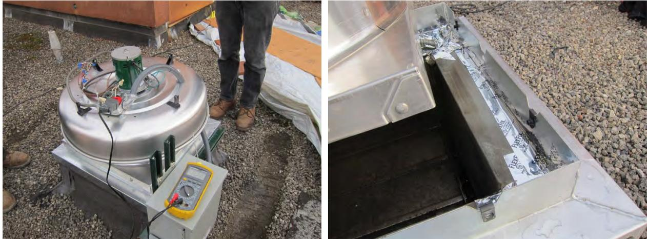
**Figure 61. Amperage measurements at rooftop exhaust fan (L); temporary seal of roof curb (R)**
