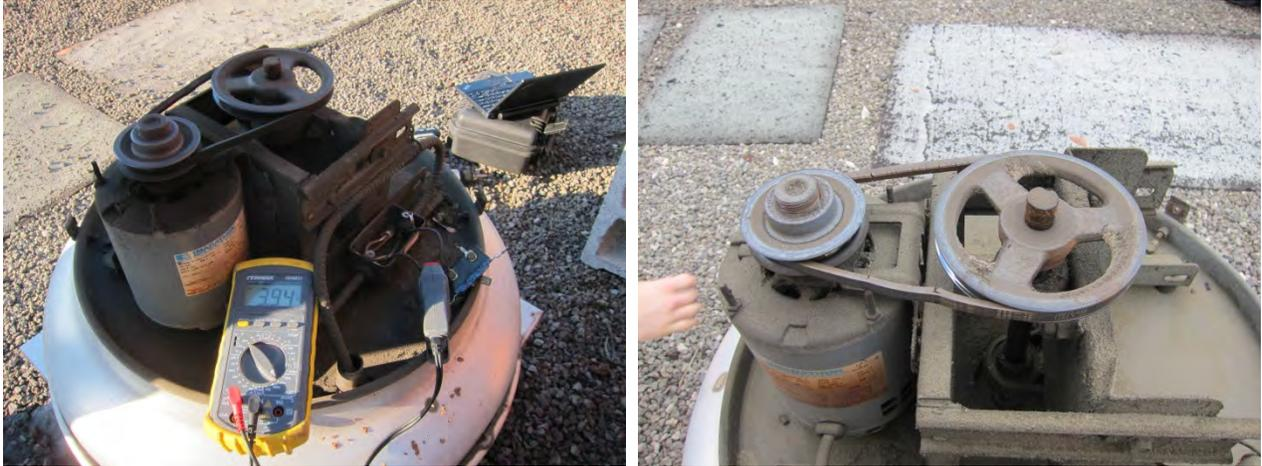
Figure 36. Measurement of amperage draw (L); loose fan belt at EF-2 (R)
