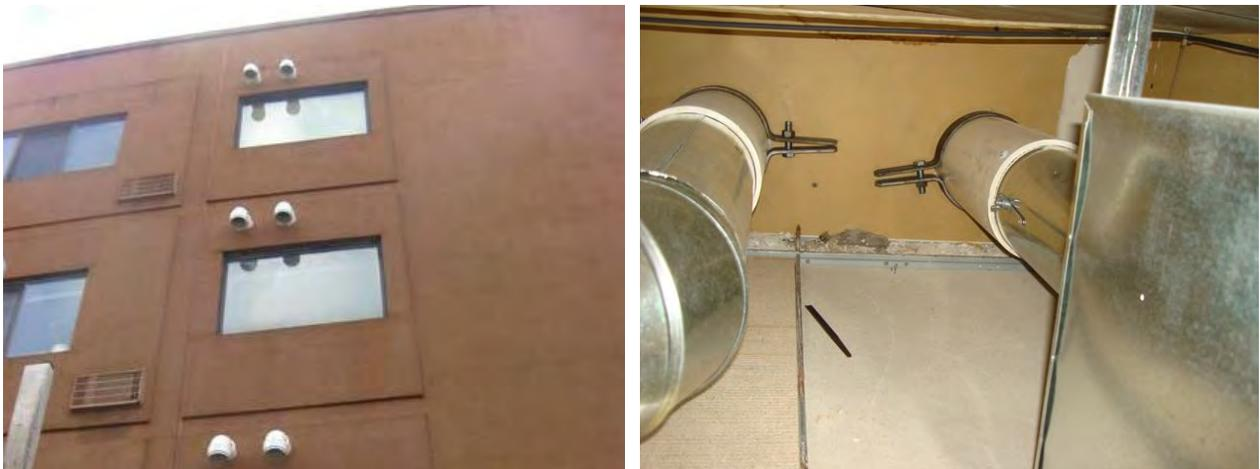
**Figure 87. Corridor ventilation exterior view (L) and connections above suspended ceiling (R)**
