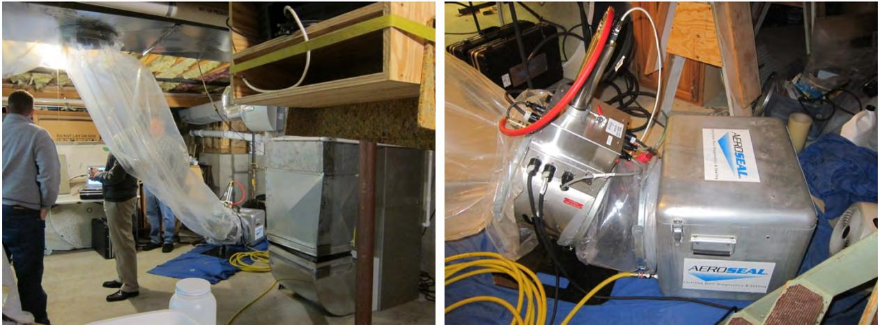
**Figure 26. Aerosol duct sealing of residential HVAC system (L); with close-up of equipment (R)**
