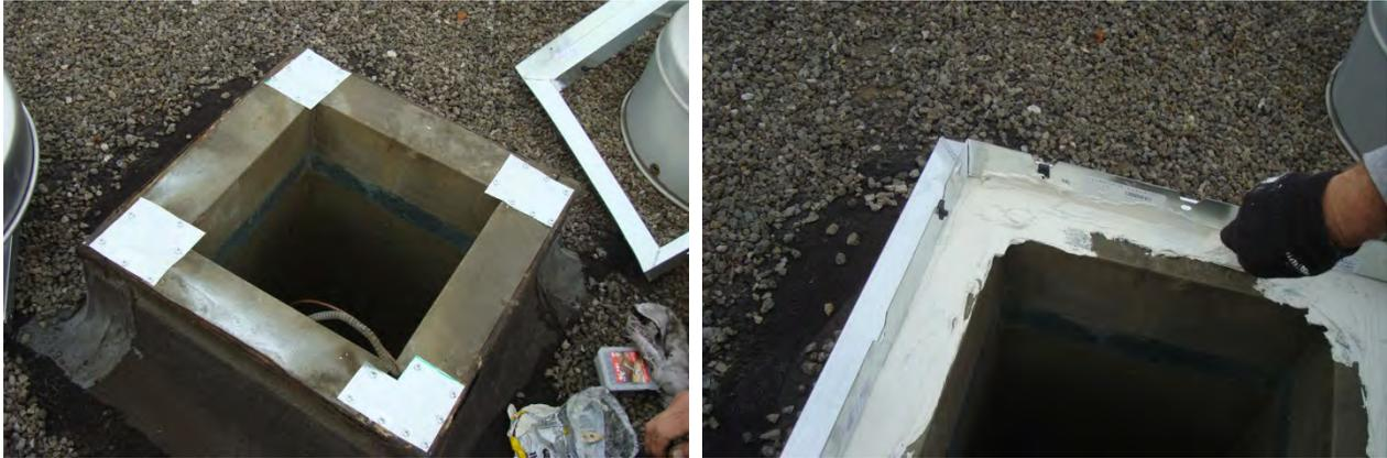
**Figure 71. Mastic and sheet metal retrofit air sealing of exhaust shaft roof curb**
