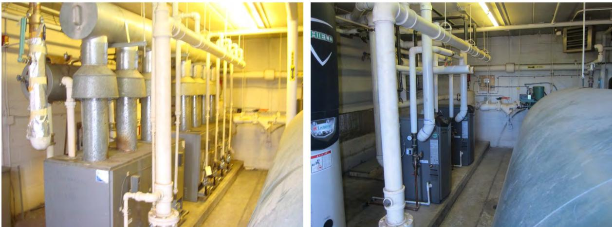
**Figure 8. Replacement of atmospheric boilers (L) with condensing sealed-combustion boilers (R)**
