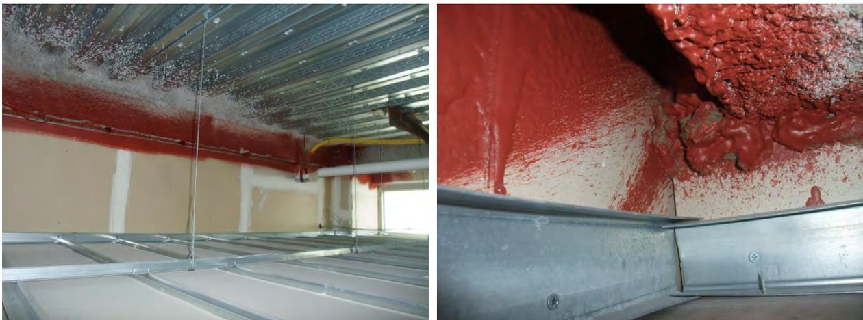
**Figure 49. Liquid spray-applied fire-rated sealant**
