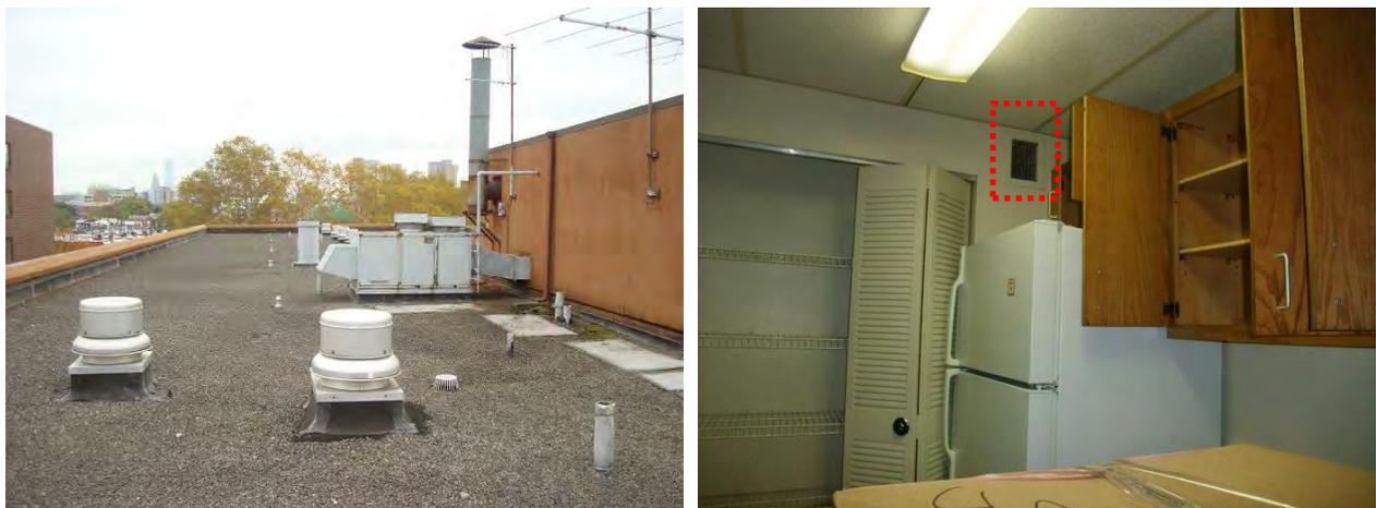
**Figure 15. Rooftop ventilation system components (L) typical kitchen exhaust grille (R)**
