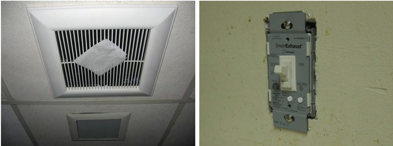
**Figure 52. Bathroom dwelling unit exhaust fan (L) and controller timer switch (R)**
