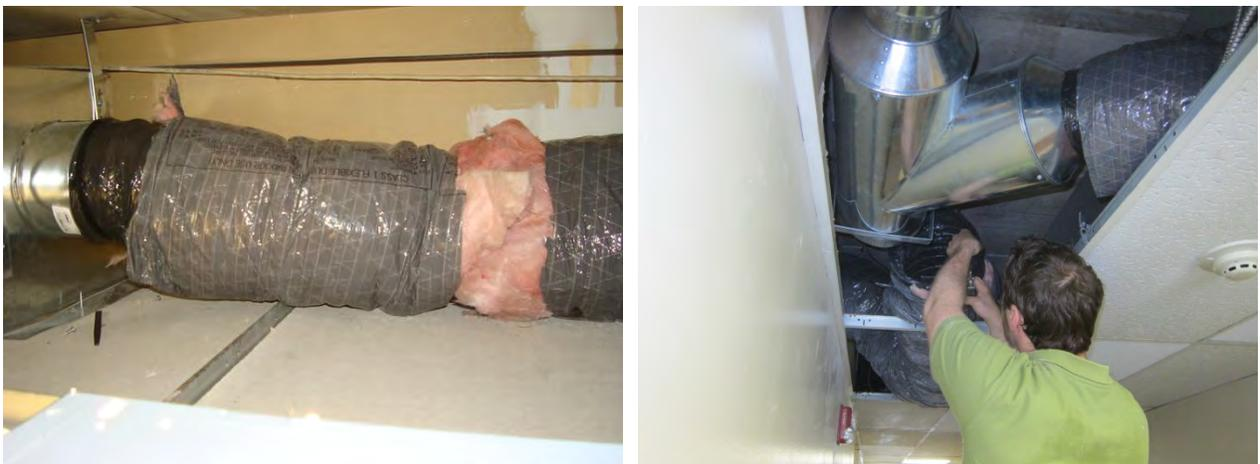
**Figure 89. Flexible duct connection (L) and wye connection (R)**
