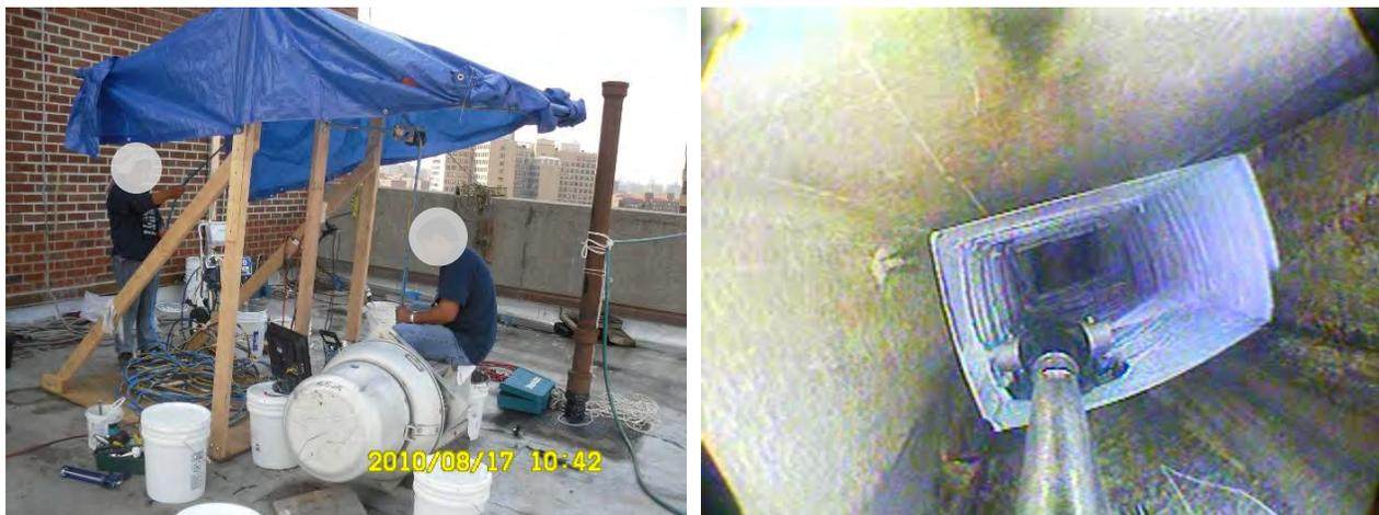
Figure 25. Remote shaft-sealing spray mastic system
