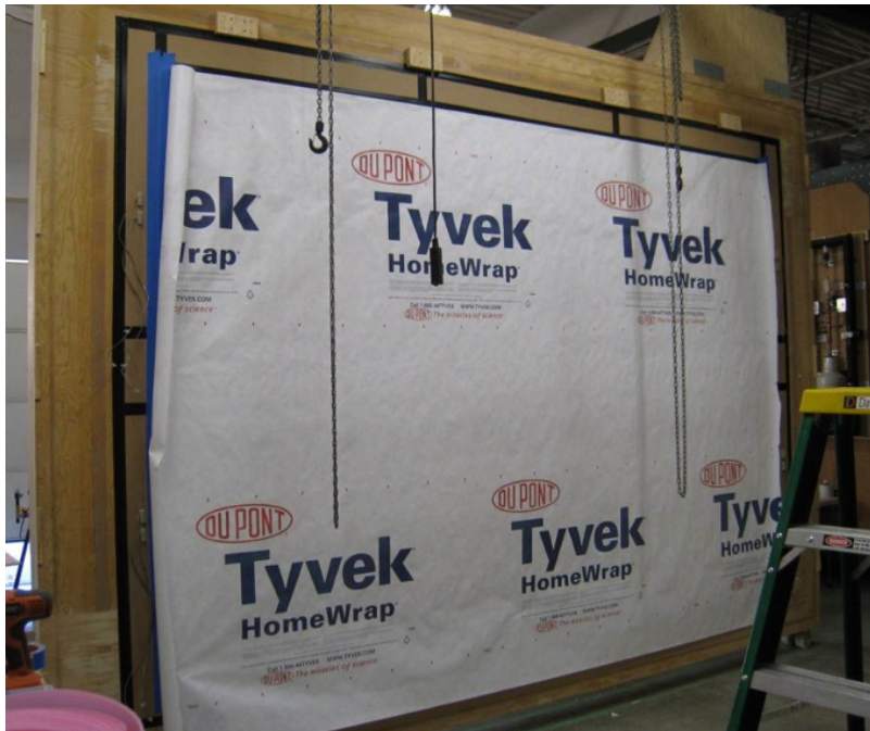
Figure 17 – Tyvek Installed but Untaped
