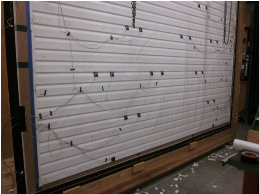
Figure 27 – Climate Box, Polyethylene Installed
