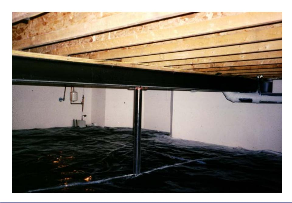
Conditioned Crawlspaces Not Unvented Crawlspaces
