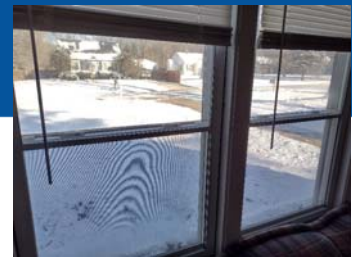
Interior low-e operable secondary window panels (storm windows) after siding replacement.
