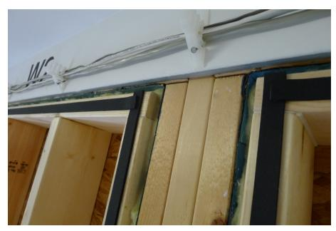
Figure 10 : Gasket installed on the interior edge of the framing as airseal
