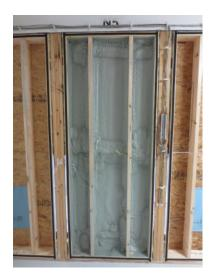
Figure 8 : North Wall 5 with approximately 2" of closed cell 2pcf spray foam
