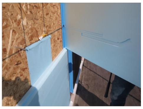
Figure 20 – Sensor and wetting apparatus tube pockets in XPS Insulation
