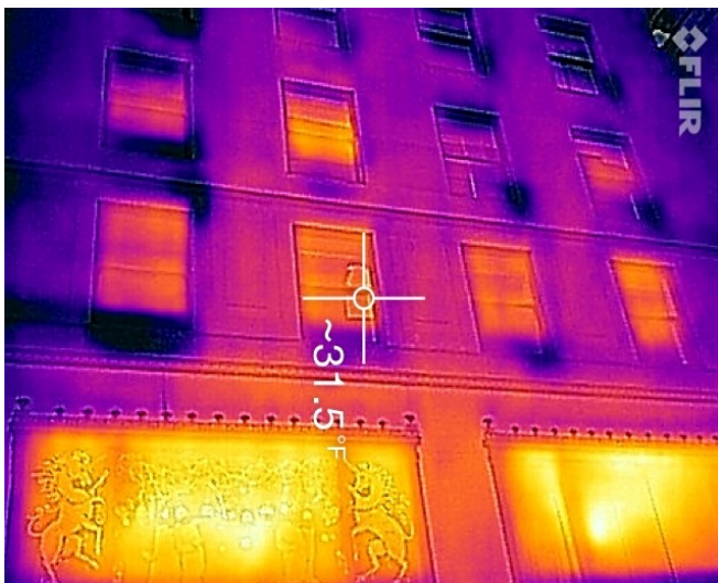
Figure 5: Exterior of masonry building, showing sill water runoff
