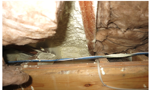
Figure 16: Spray foam imperfections at wood-to-wood joints
