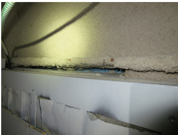
Figure 3: Beam-to-wall interface (above ceiling)
