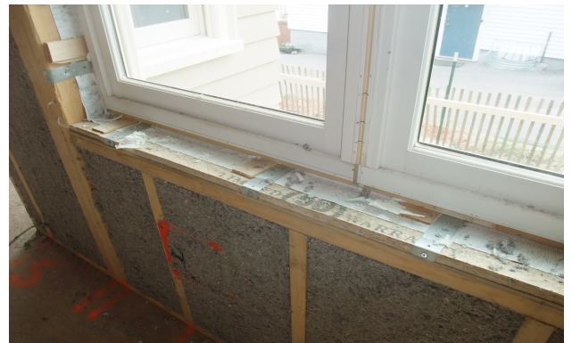
Figure 16: Spray foam imperfections at wood-to-wood joints
