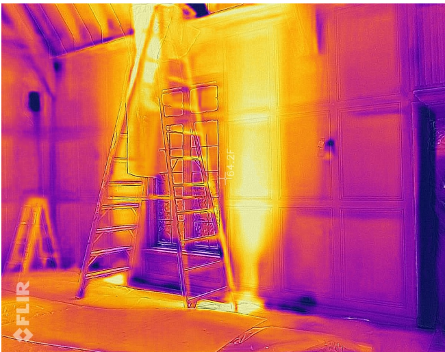
Figure 7: Hot “plumes” from floor registers in heating operation
