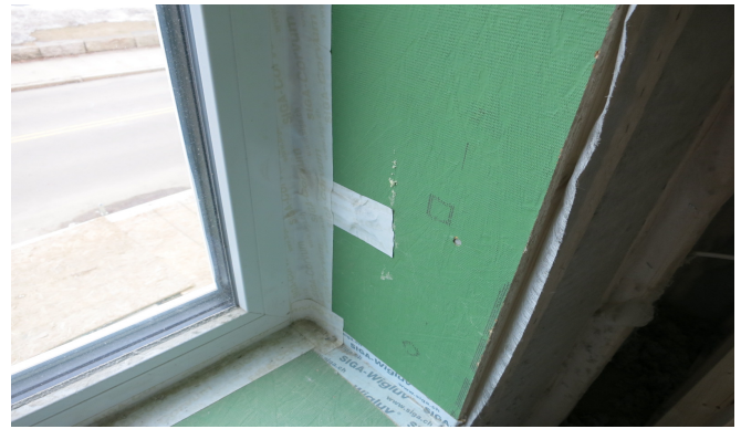
Figure 18: Air sealing window by covering installation clip with tape
